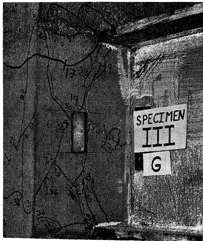
Fig. 4.10 A view of joint 3 after failure. (Top flange in tension in L1 and U1)
