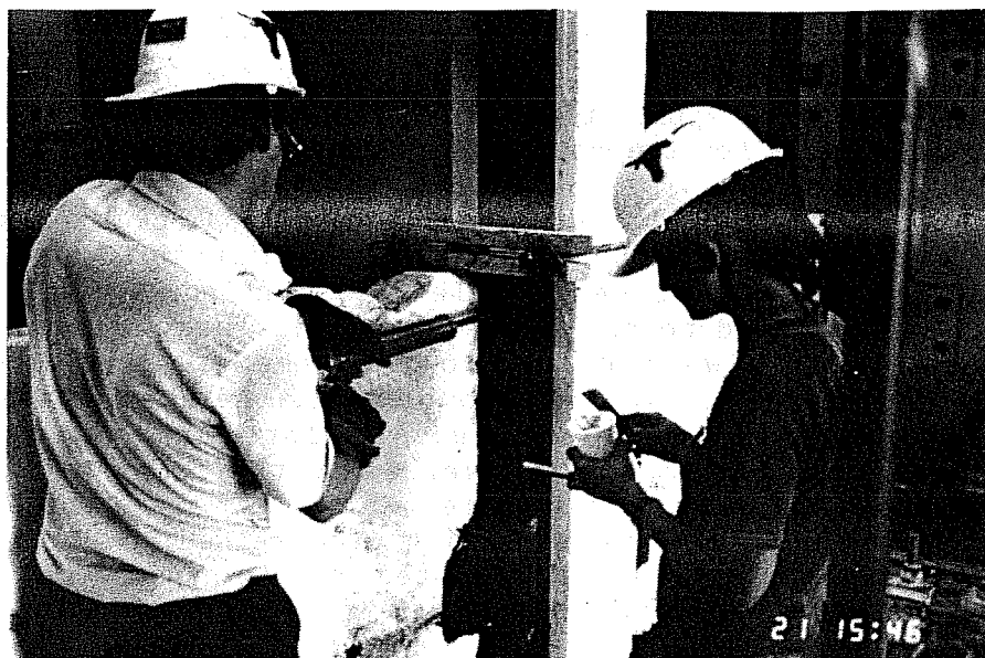
Fig. 3.23 Epoxy application procedure
