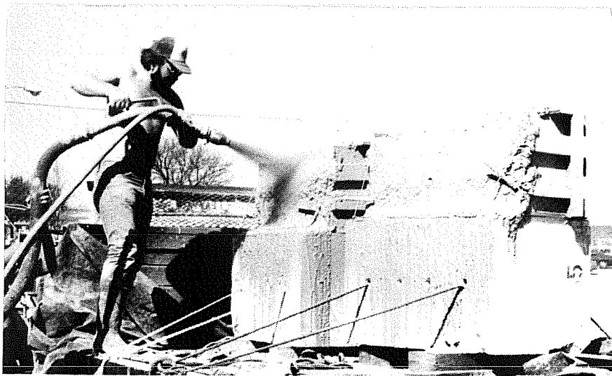
Fig. 3.29 Shotcreting process of wing wall 5B and 6B
