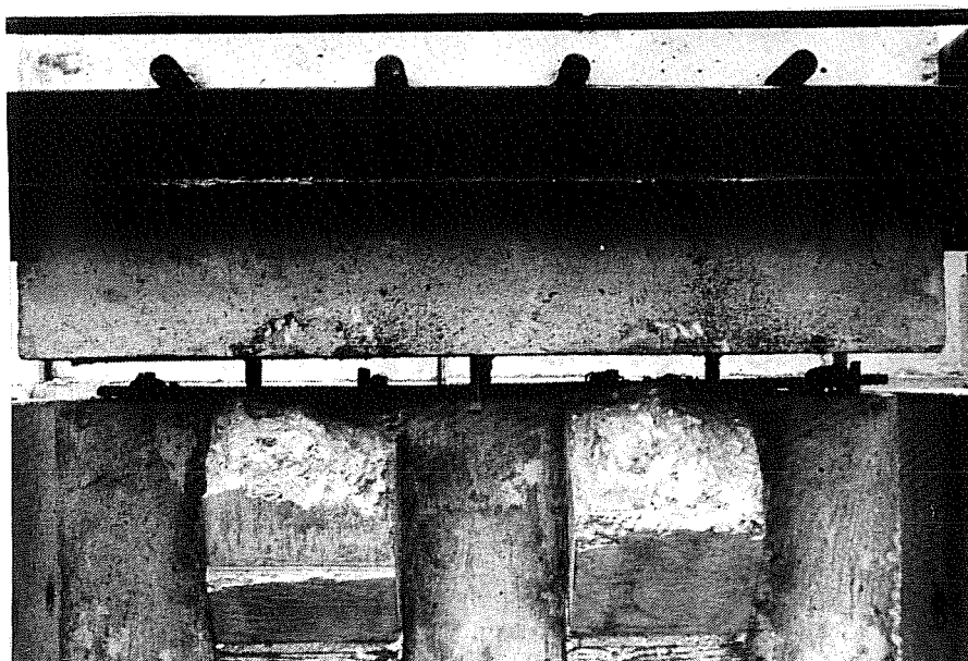
Fig. 3.18 Overhead casting position before drypacking
