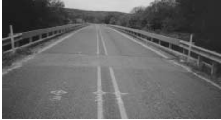
Figure 1.17: The surface of the Leon River Bridge
