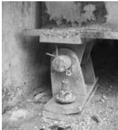
Figure 1.3: A rocker support at an abutment
