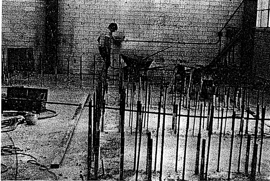
Fig. A13 Dowels in floor slab
