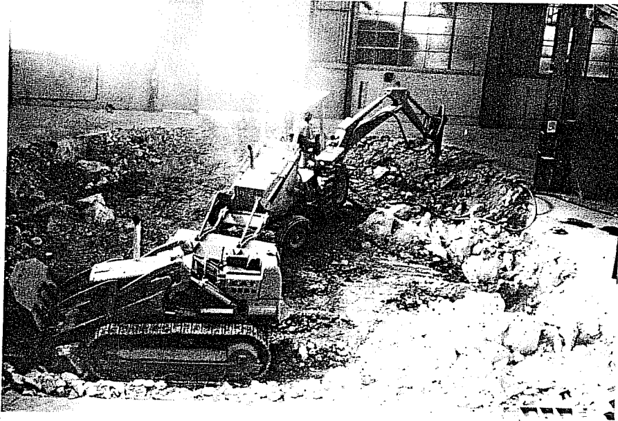
Fig. A1 Excavation for the floor slab
