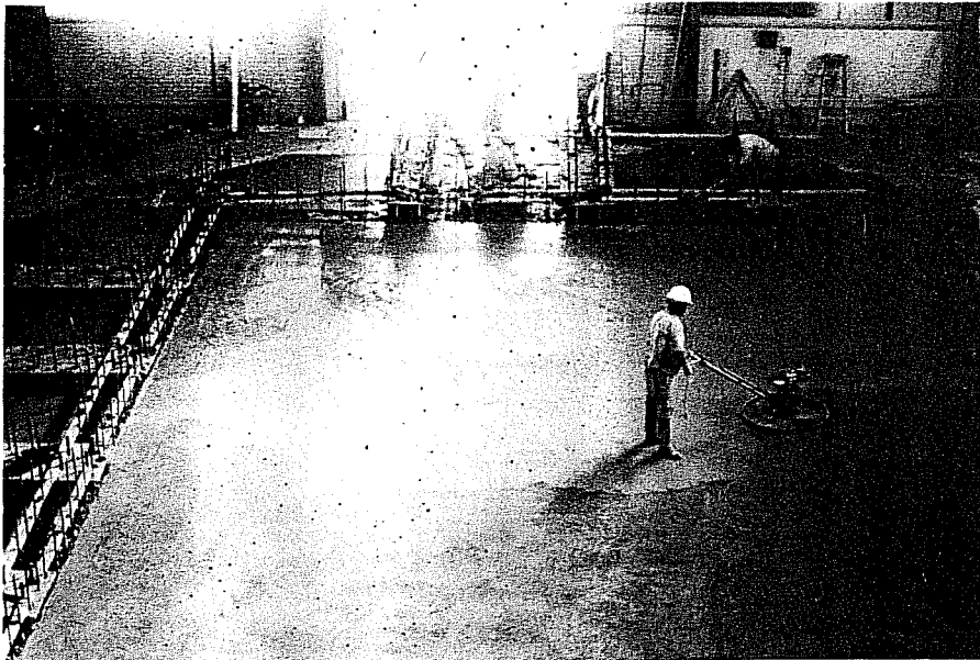
Fig. A12 Float finishing of the finished floor slab
