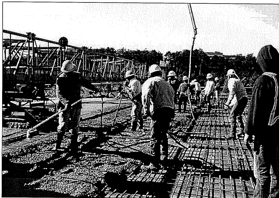
Figure 4. 11 Casting operations for the bridge decks
