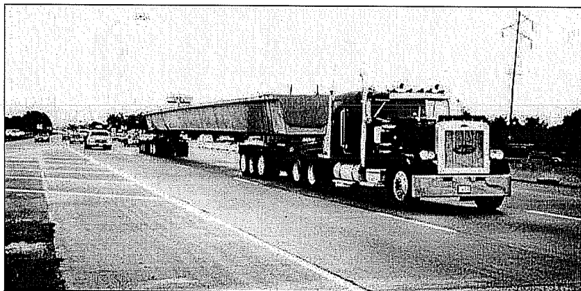
Figure 4.6 U-beam being transported to the job site
