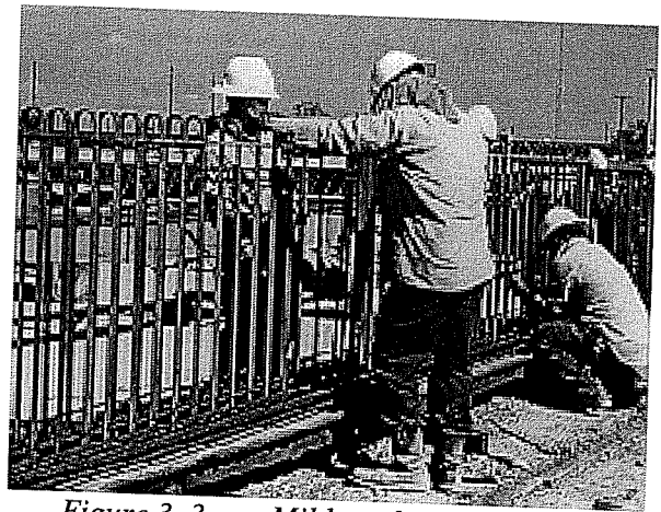
Figure 3.3 Mild steel reinforcement
