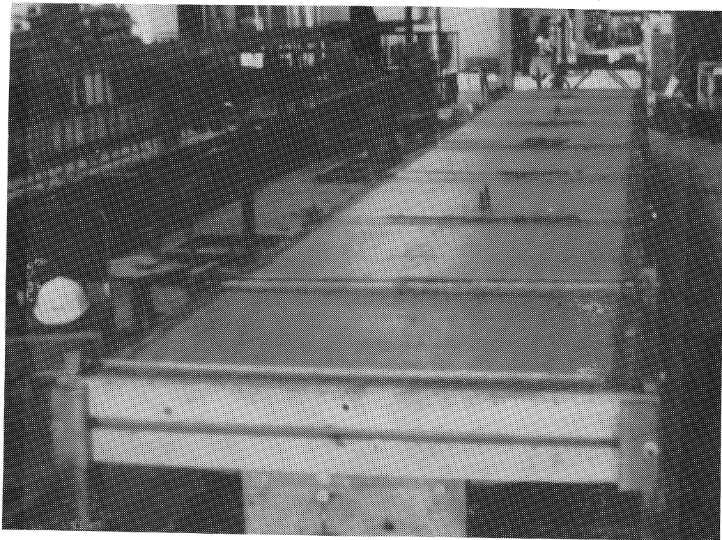
Fig. 2.19 Formwork prior to and after casting
