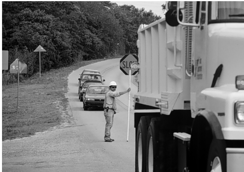
Figure 3.20 Traffic Control during Test
