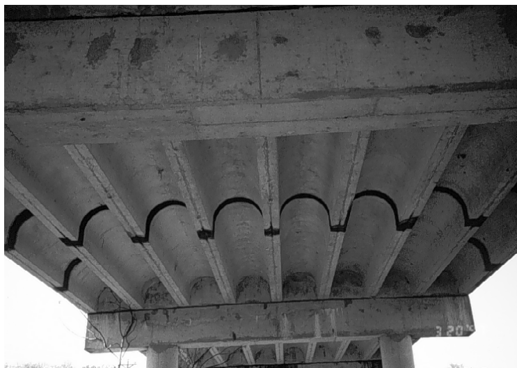
Figure 3.2 Instrumented Span Viewed from Below
