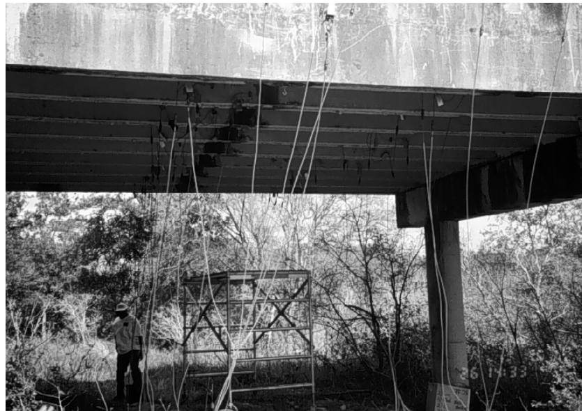
Figure 3.15 Cables Suspended from Bottom of Bridge
