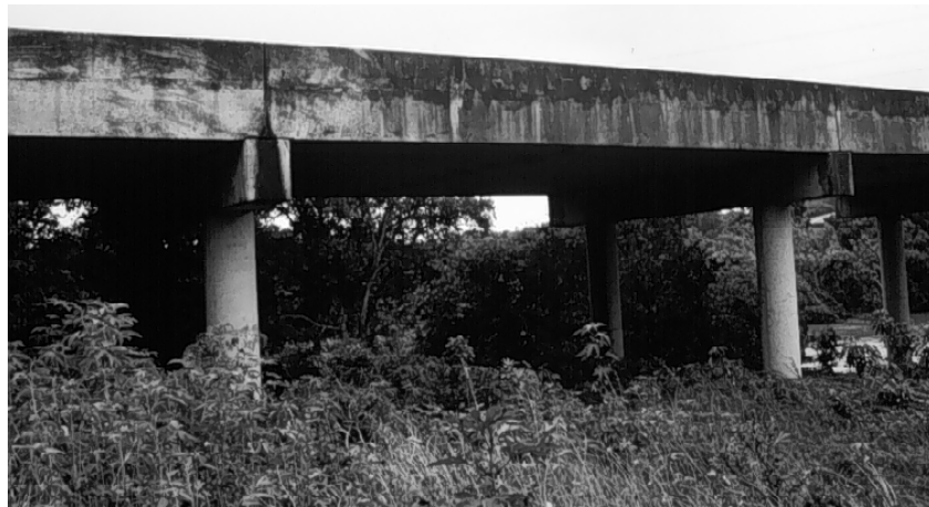
Figure 3.1 Instrumented Span Viewed from the South
