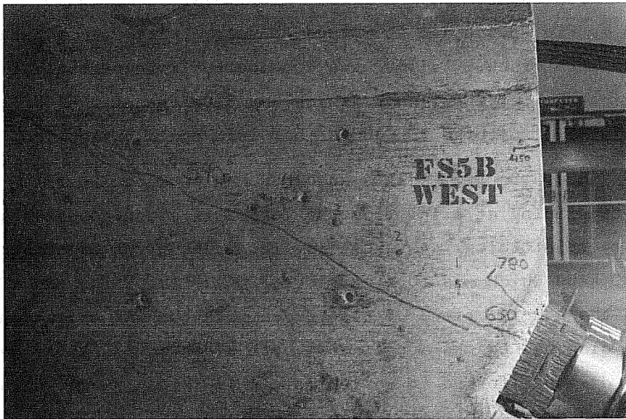
(a) First cracking at 540 kips along tendon path
