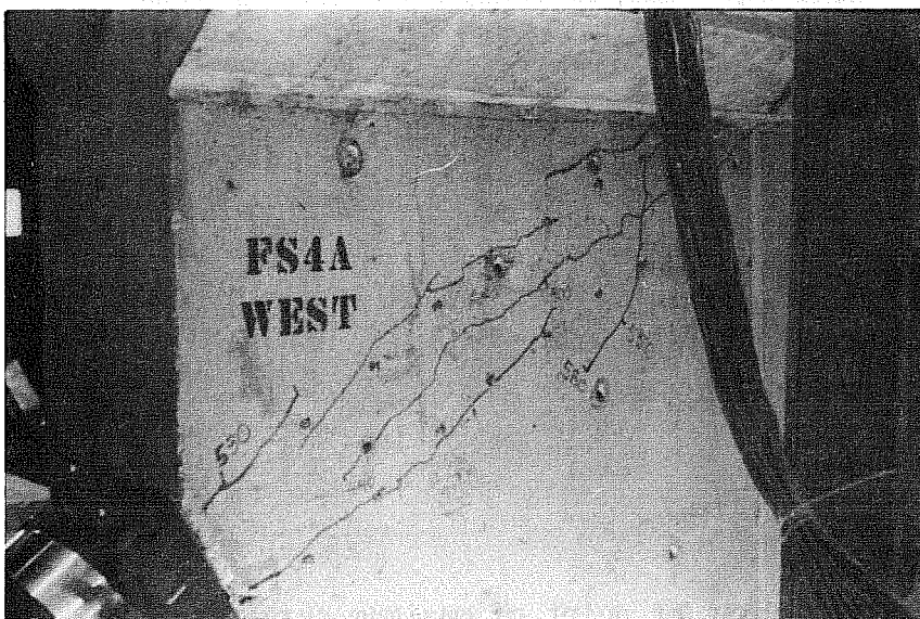
(c) Multiple longitudinal cracks prior to failure
