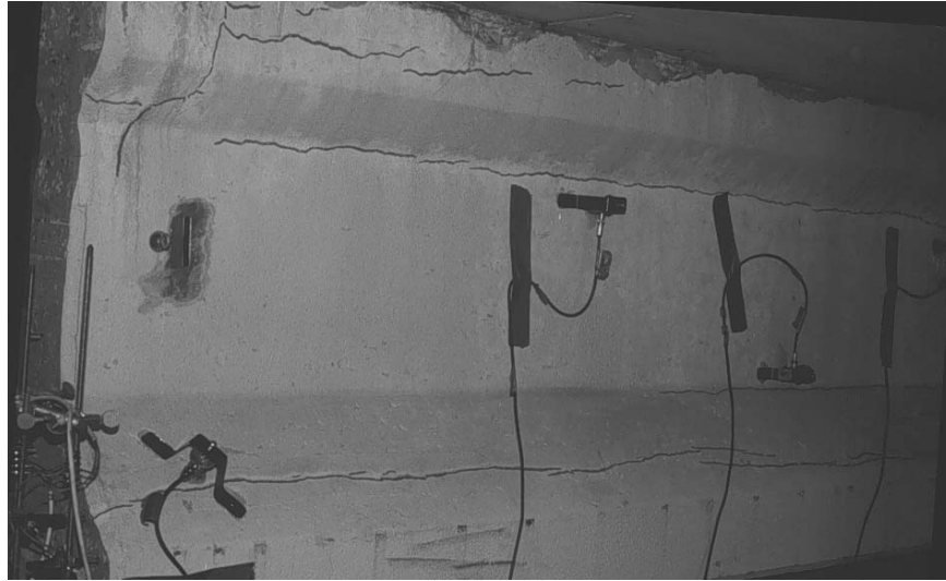
Figure 3.15 – East End of Girder 2
