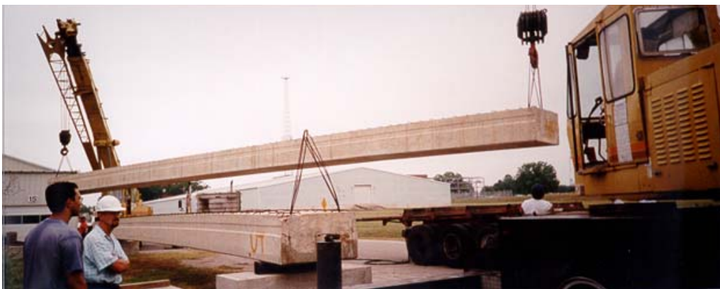
Figure 2.3 – Overall View of Box Girder
