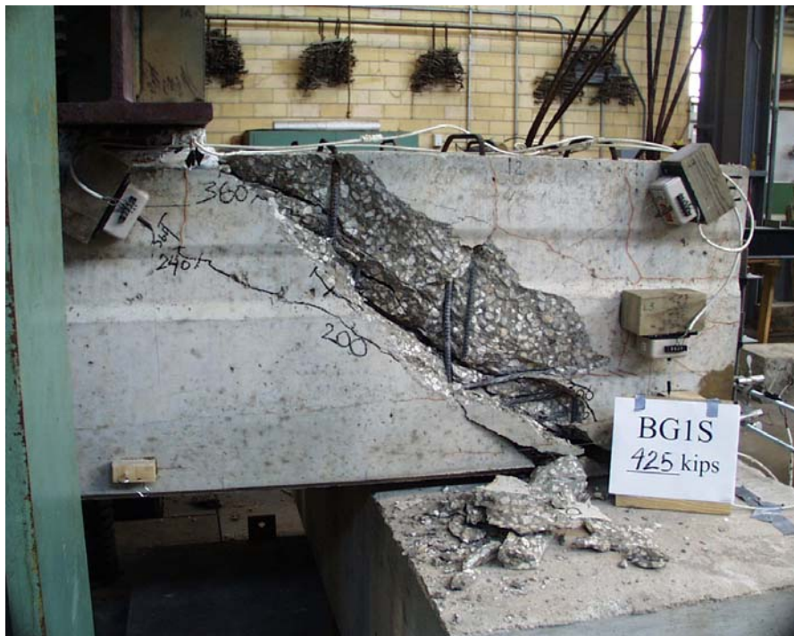
Figure 4.33 – Compression Strut Failure of BG1S
