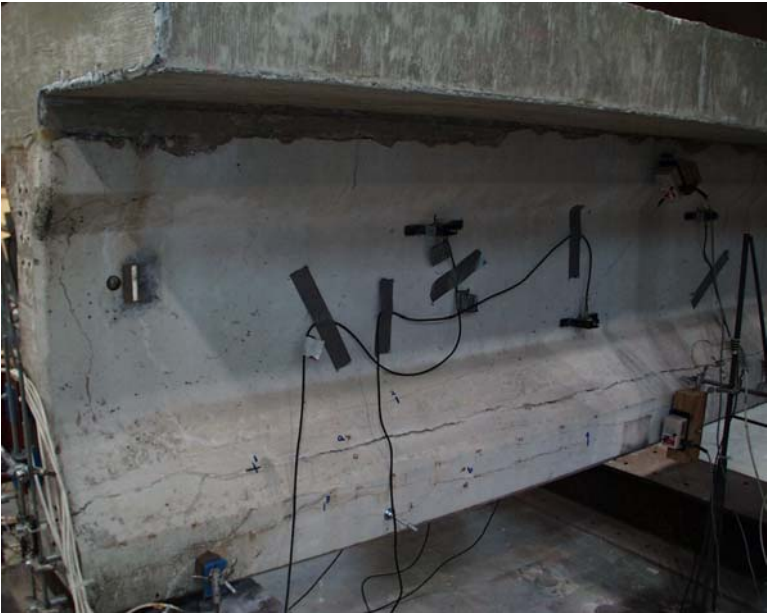
Figure 3.14 – East End of Girder 1
