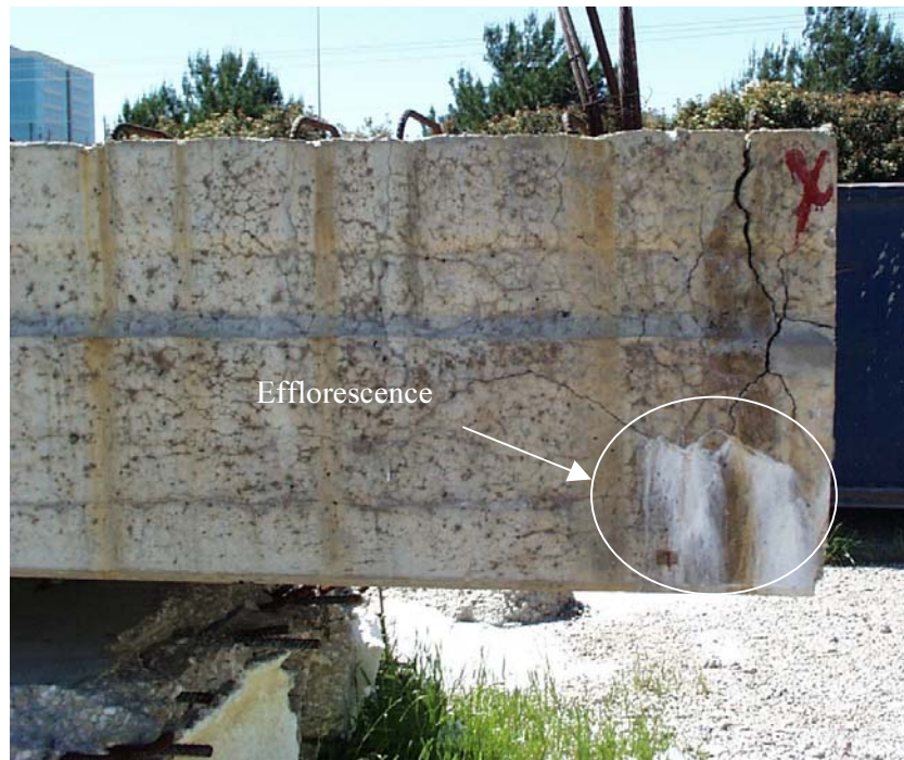
Figure 3.10 – Side View of A-End of BG4
