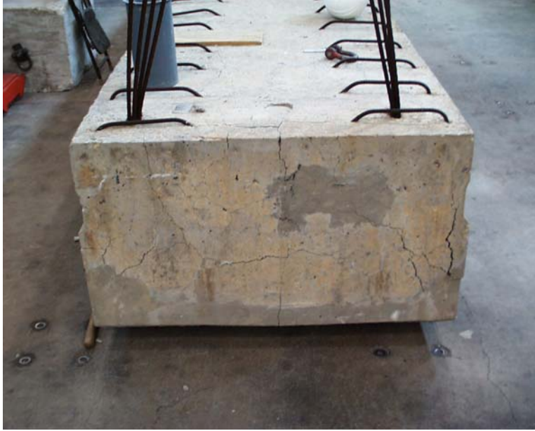
Figure 3.7 – End View of A-End of BG3
