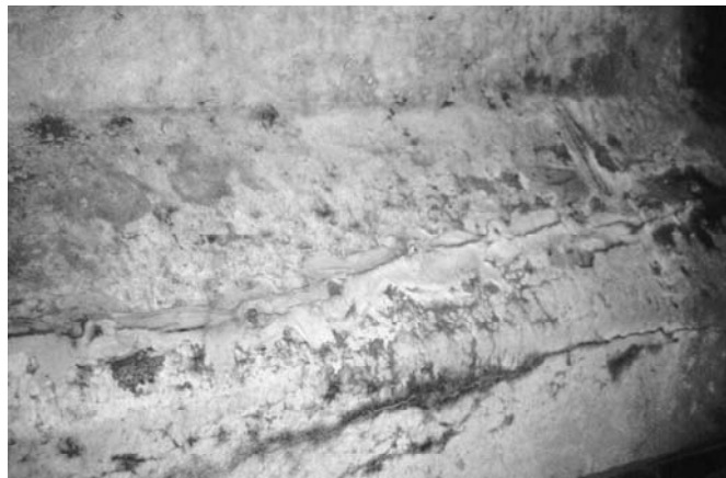
Figure 7.3 Injected sealant on I-10 structure
