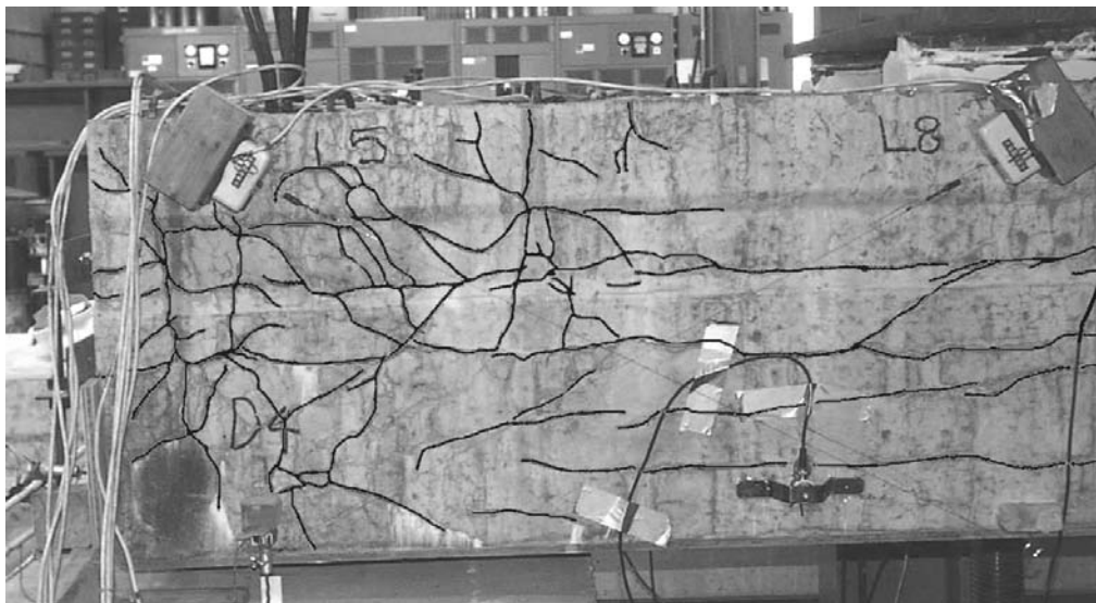
Figure 4.39 Pre-existing cracks on the east face of BG4S
