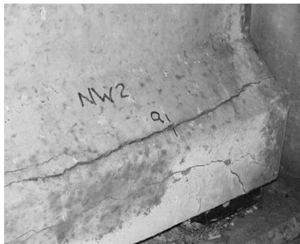
Figure 7.12 Point “a” on NW Girder 2 of US-90 structure
