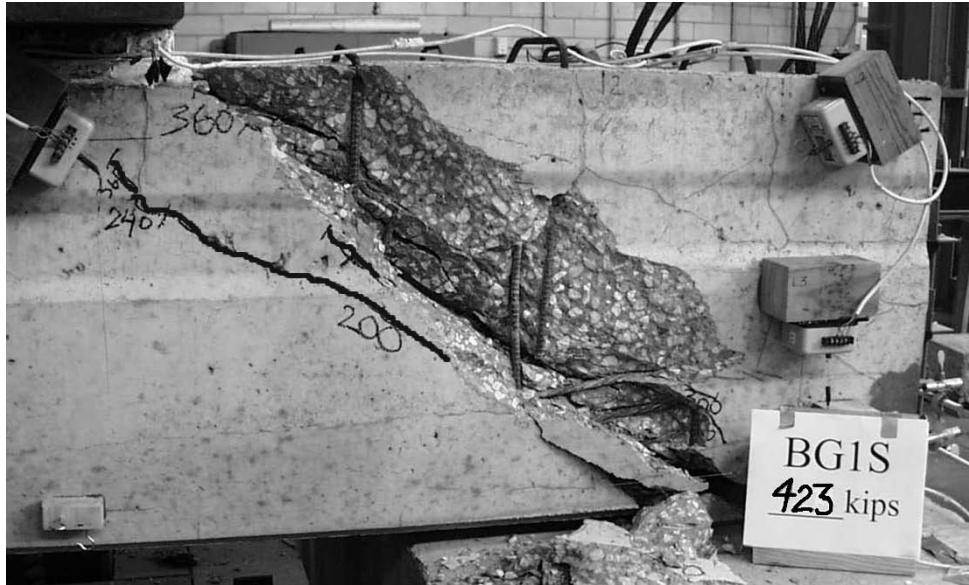
Figure 4.22 Failure of the east face of BG1S at 423 kips (1880 kN)
