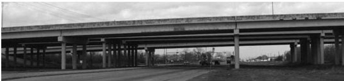
Figure 6.4 Beltway 8 at State Highway 3
