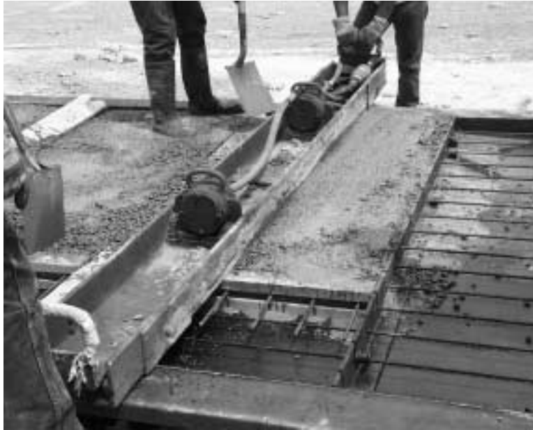
Figure 8.8 Lightweight Concrete Panel Casting
