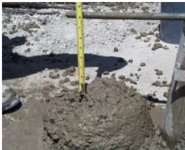
Figure 4.8 Slump of First Batch of 6000 psi Concrete
