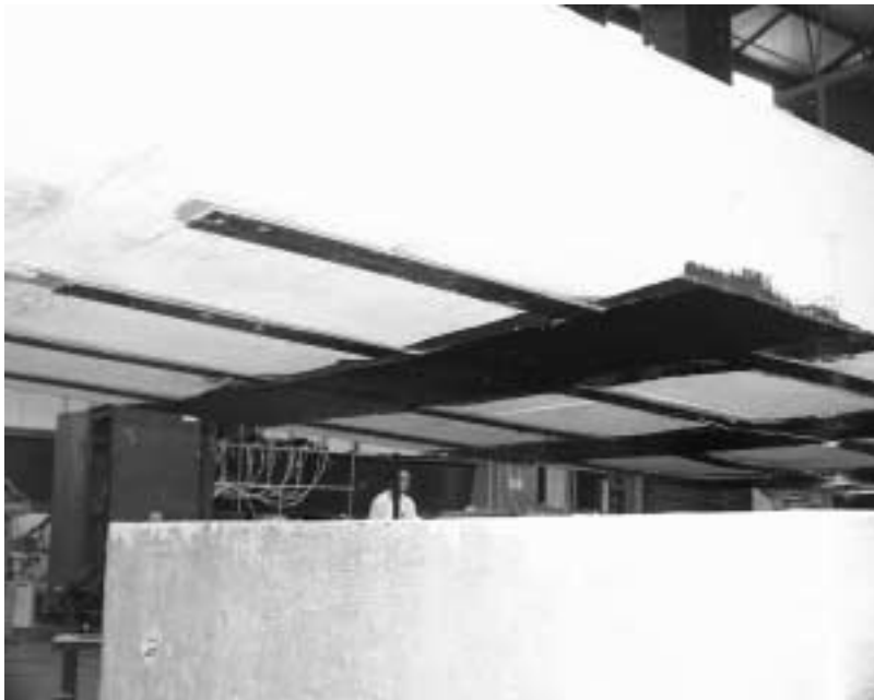
Figure 7.8 South End of the CFRP Plates Still Attached After Failure of Specimen FS-1
