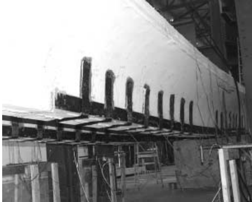
Figure 4.8 East Joist of Specimen J-1 Before CFRP Debonding
