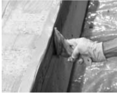
e) Positioning CFRP plate on beam
