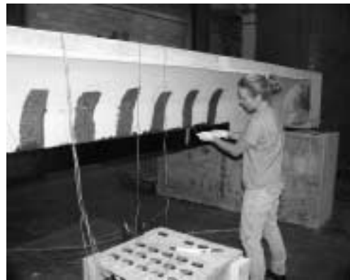
f) Coating placed sheets with epoxy
