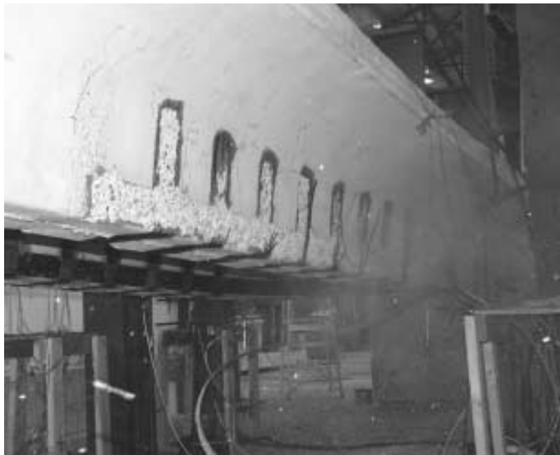
Figure 4.9 East Joist of Specimen J-1 at Failure
