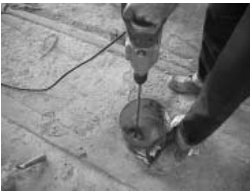
c) Mixing epoxy paste
