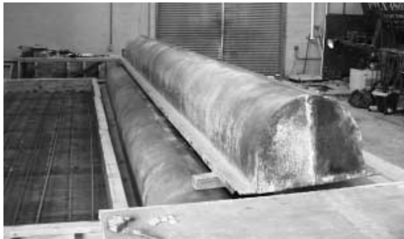
Figure 3.1 View of Metal Pan-Forms inside the Laboratory
