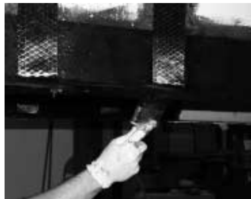
f) Coating placed sheets with epoxy
