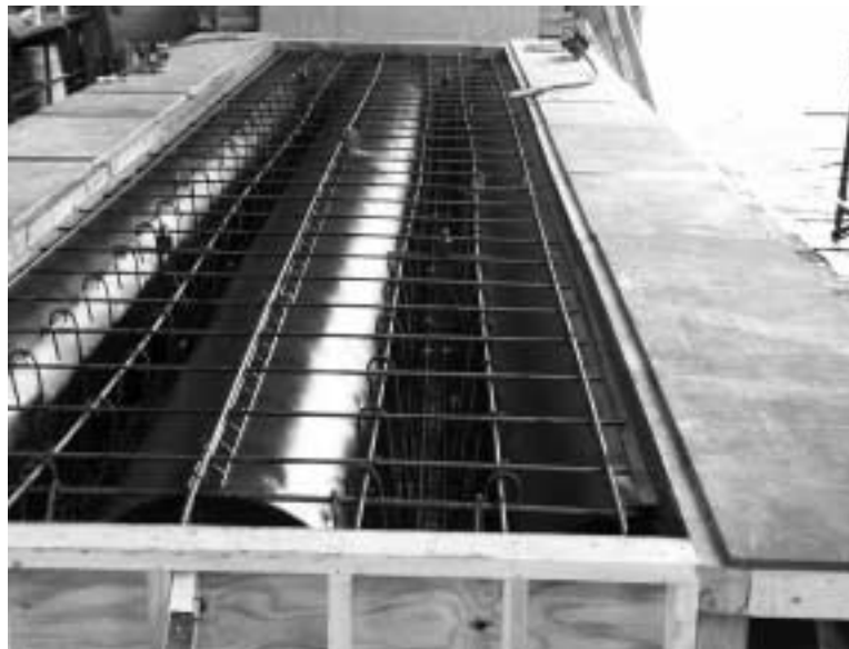
Figure 3.6 Specimen Reinforcement and Formwork
