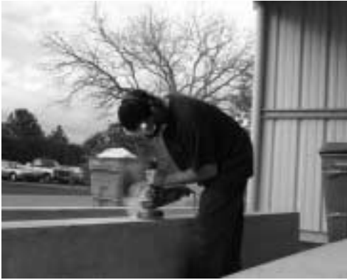
b) CFRP plate cleaning
