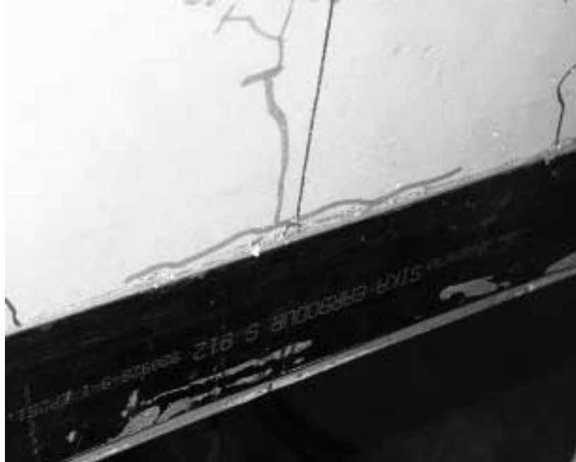
Figure 4.6 Observed Initial Debonding of CFRP Plate on East Joist
