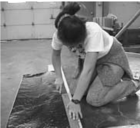
c) Applying epoxy to surface
