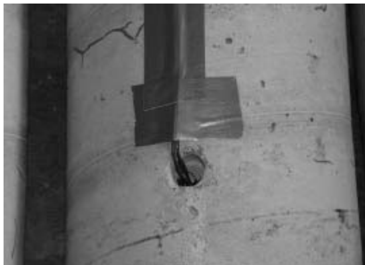
Figure 8.6 Installation of the embedded electrodes
