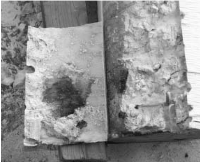
Figure 6.13 Moisture trapped beneath the surface in the splash zone of specimen CNC14
