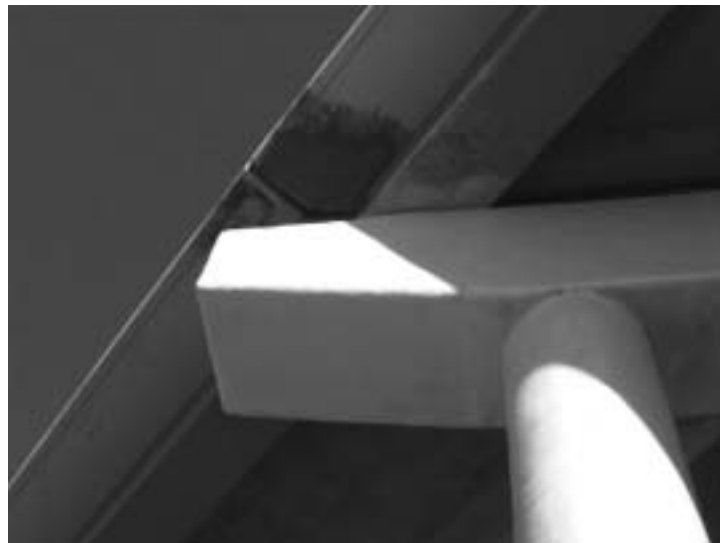
Figure 1.2 Bridge bent and column wrapped with FRP after repair of corrosion damage
