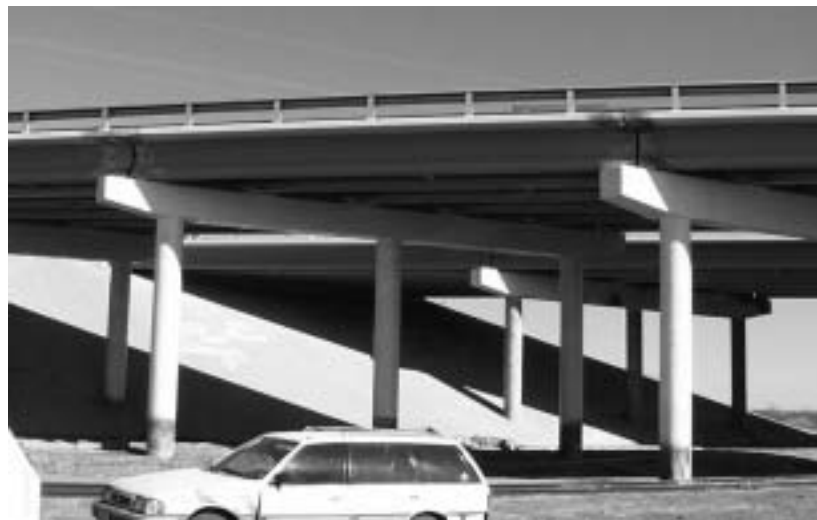
Figure 5.12 Structure #2 encapsulated with FRP wrap
