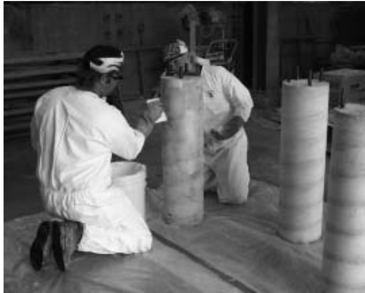
Figure 8.2 Filling voids with a thickened epoxy filler
