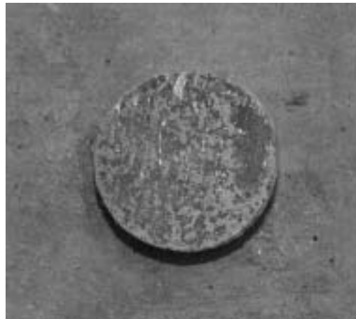
Figure 6.12 Failure at the epoxy/concrete interface on Test #2
