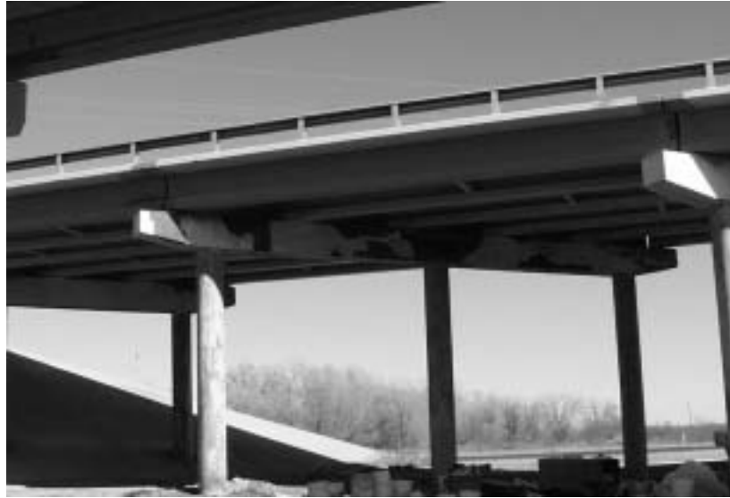
Figure 5.11 Structure #1 prepared for encapsulation
