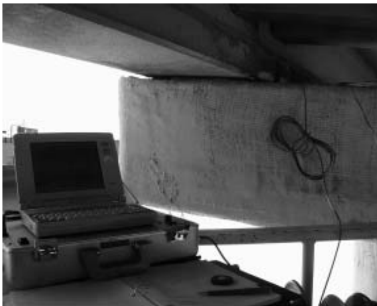
Figure 7.2 PR-Monitor test setup for Structure #12
