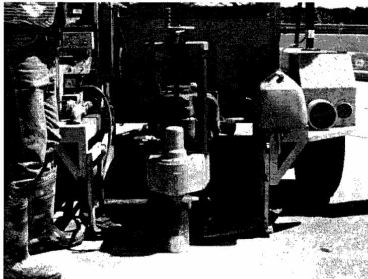
Figure 4.10 Drilling of Concrete Core in Progress.
