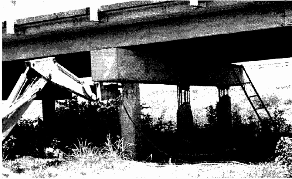
Figure 5.1 Removal of Bent Cap in Progress at Unit-N.
