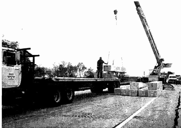
Figure 5.8 Barrier Placement on Flatbed of Trailer.
