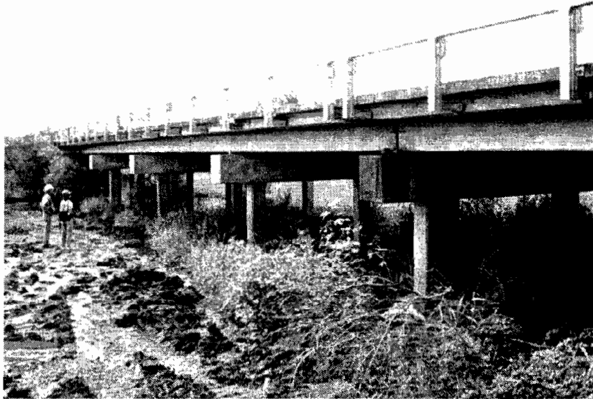
Figure 4.3 View of Big Creek Relief Bridge from East Side.
