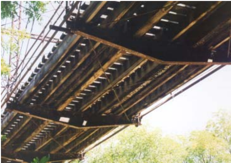
Figure A.17: View of deck from underneath main truss span
