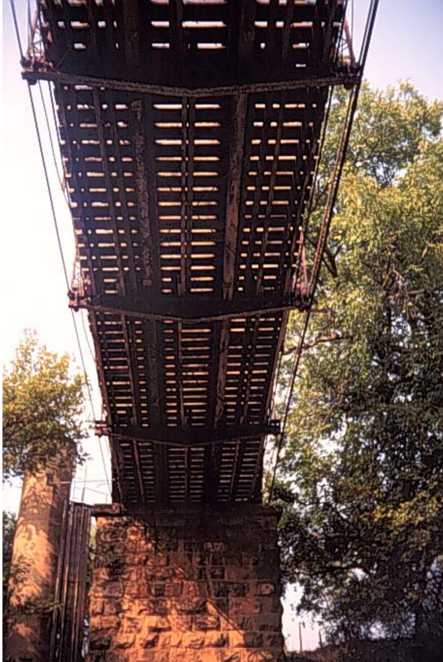
Figure A.20: South stone masonry pier
