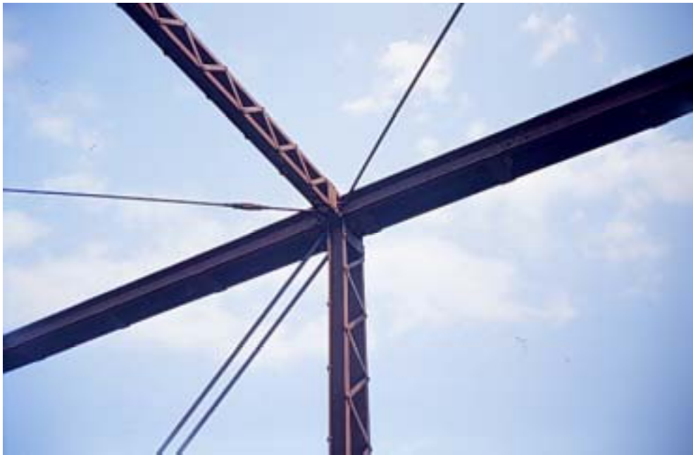
Figure A.15: Upper chord joint U2
