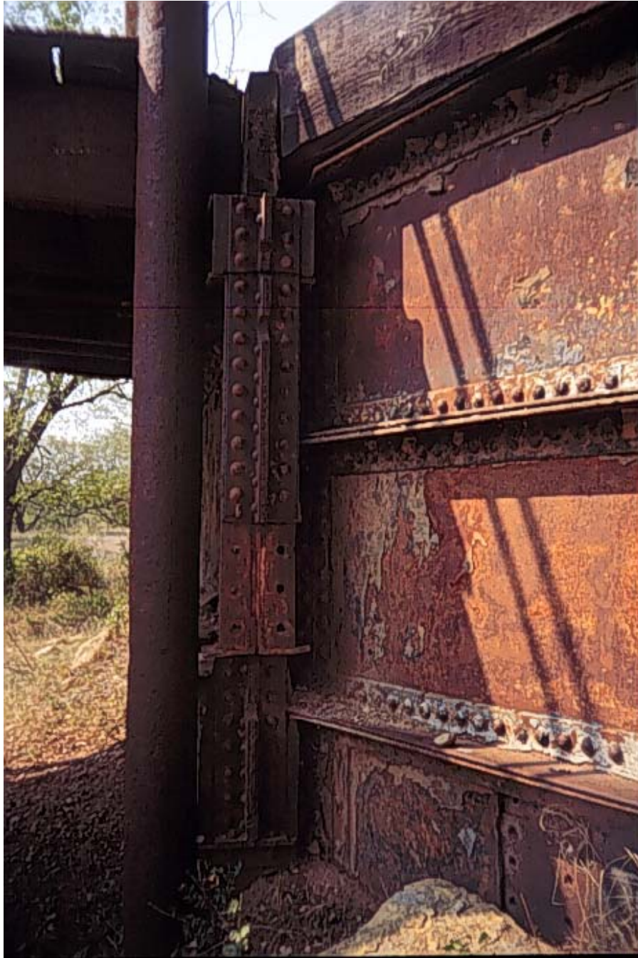
Figure A.38: Metal retaining wall at the north abutment
