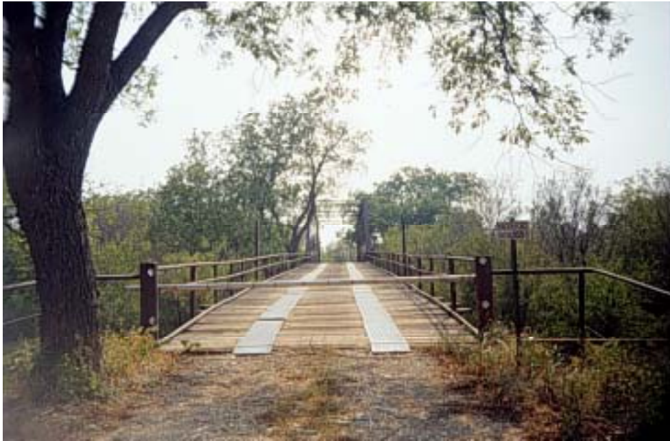
Figure A.1: Case study bridge – View looking south
