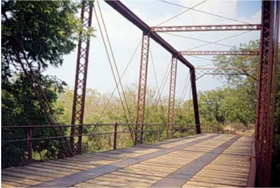
Figure A.5: Upstream truss
