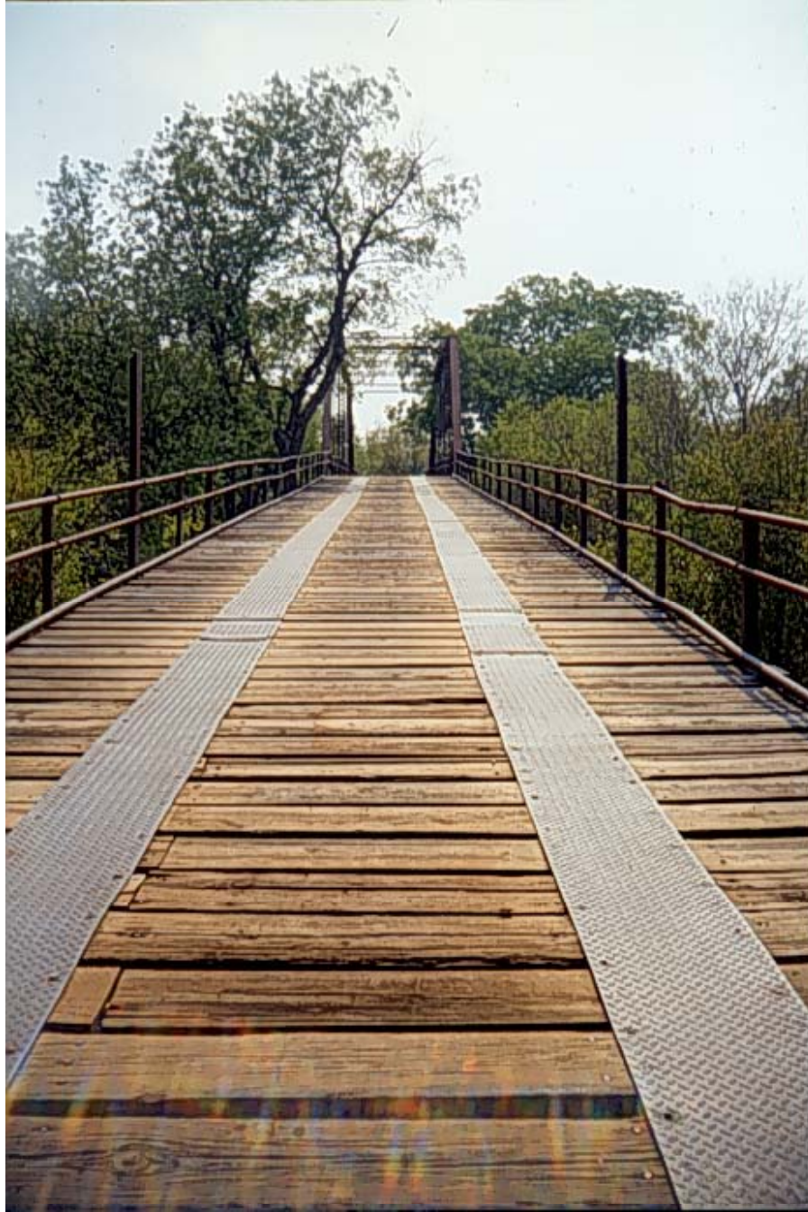
Figure A.27: Timber deck on the north approach span
