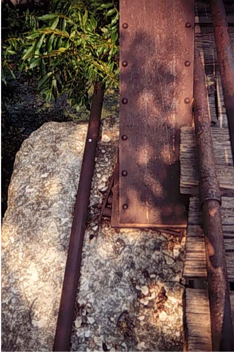
Figure A.7: Roller support at southwest corner of main truss span
