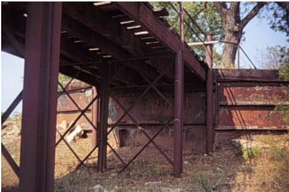
Figure A.37: Metal retaining wall at the north abutment
