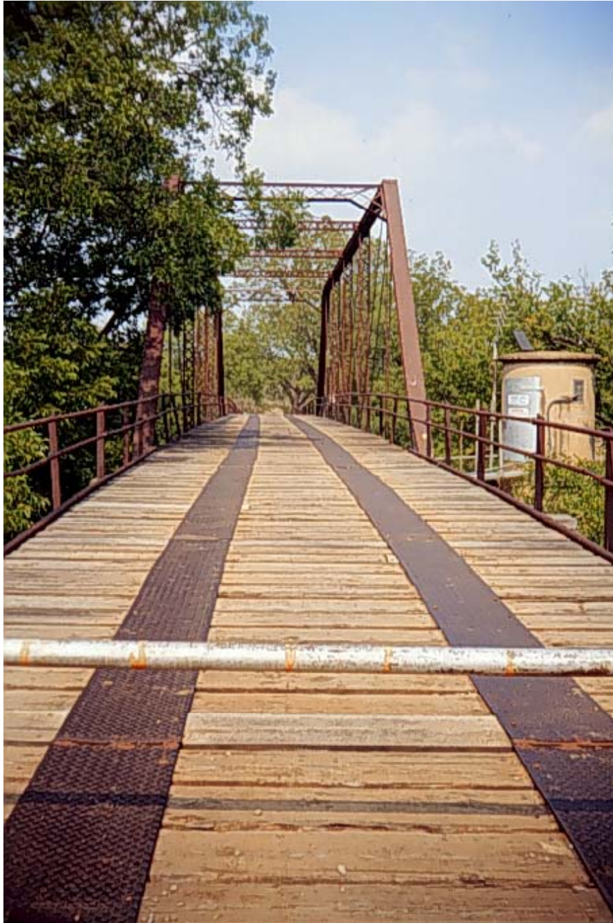
Figure A.25: Timber deck on the south approach span
