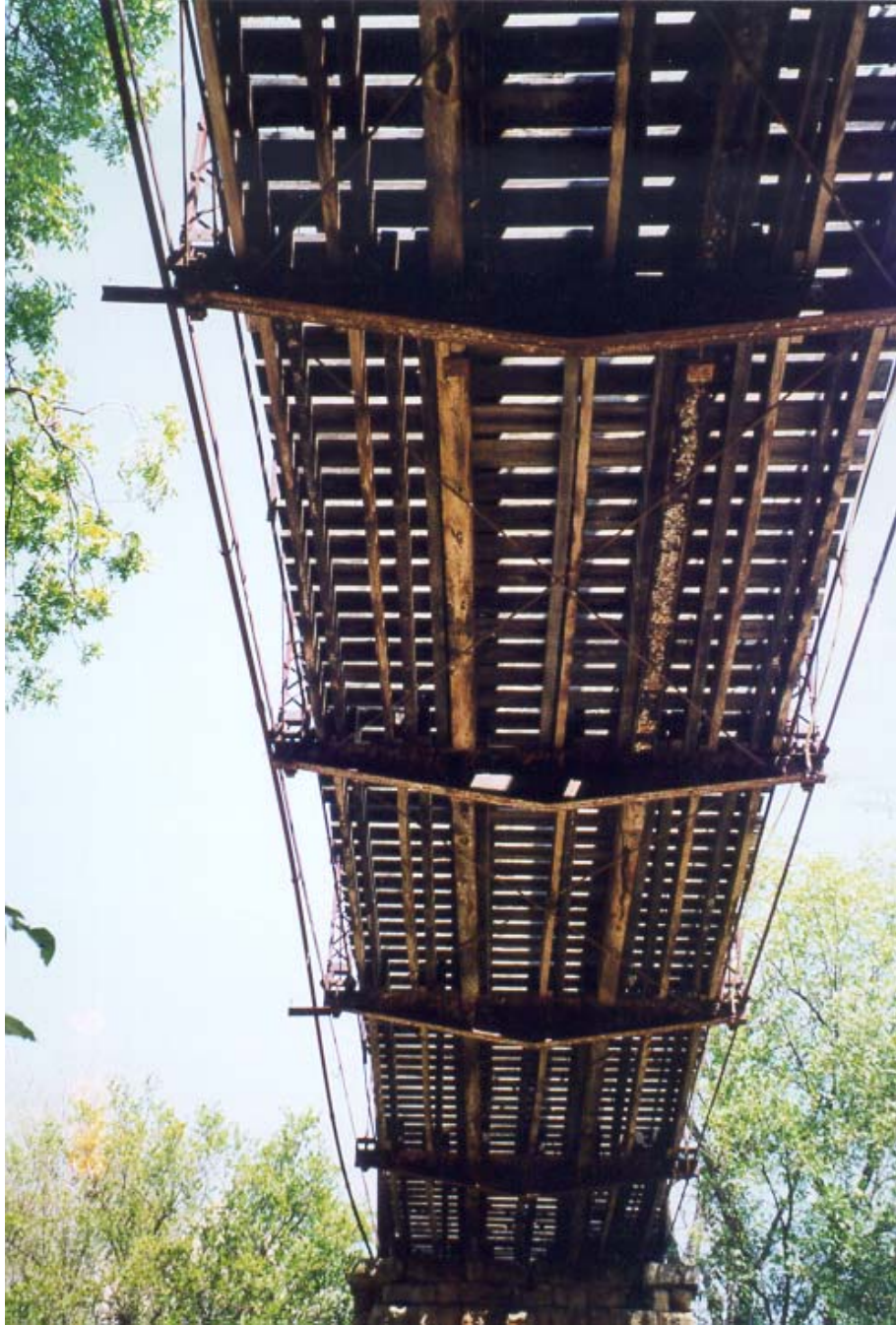
Figure A.18: View of deck from underneath main truss span
