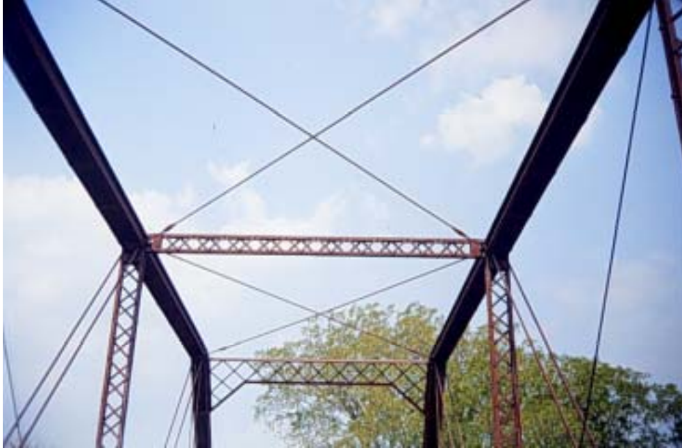
Figure A.21: Top lateral bracing system
