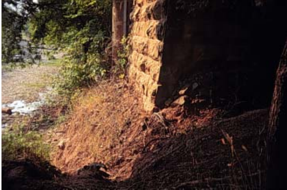
Figure A.30: Base of the south pier
