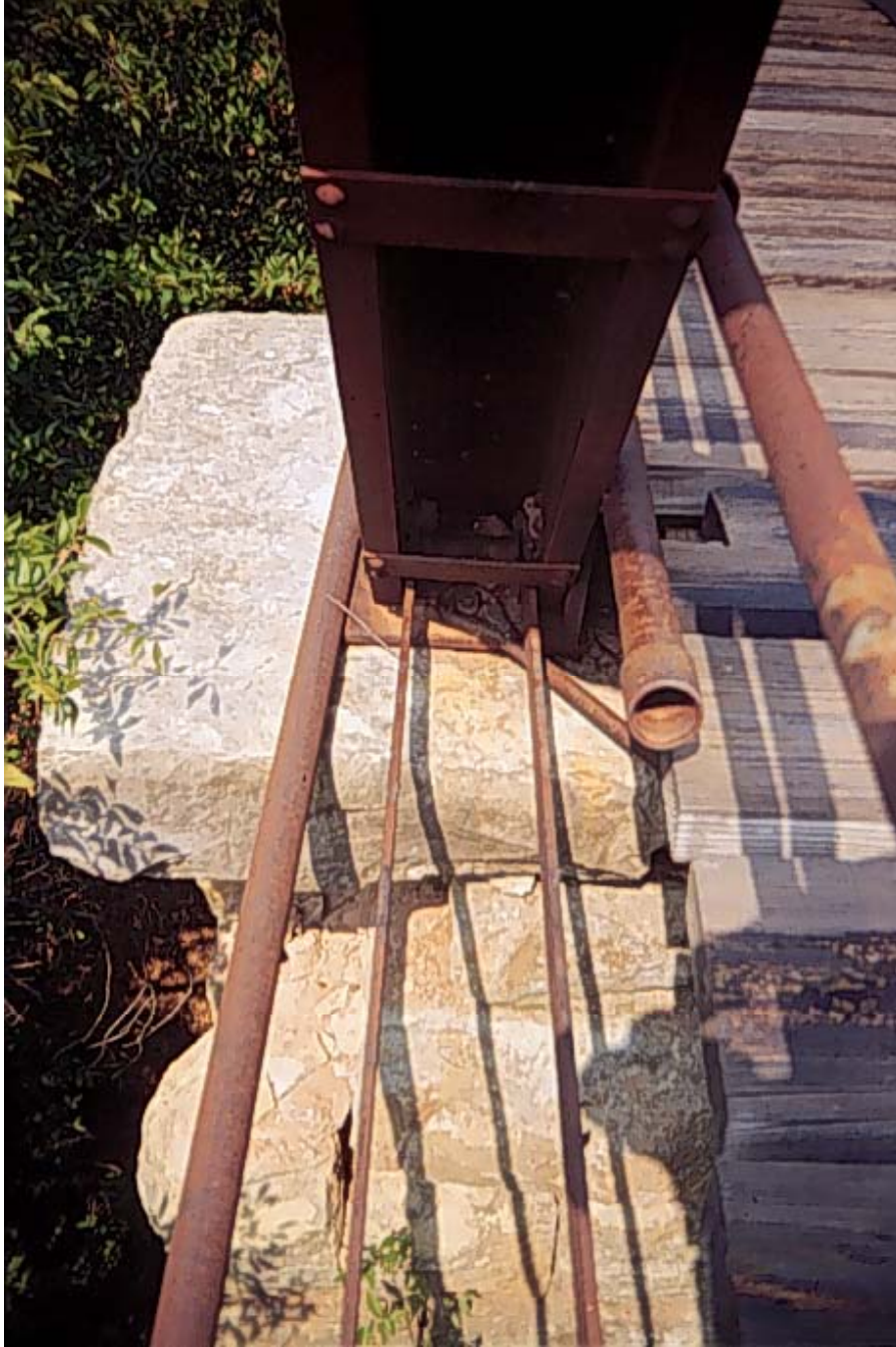
Figure A.8: Hinge support at northwest corner of main truss span
