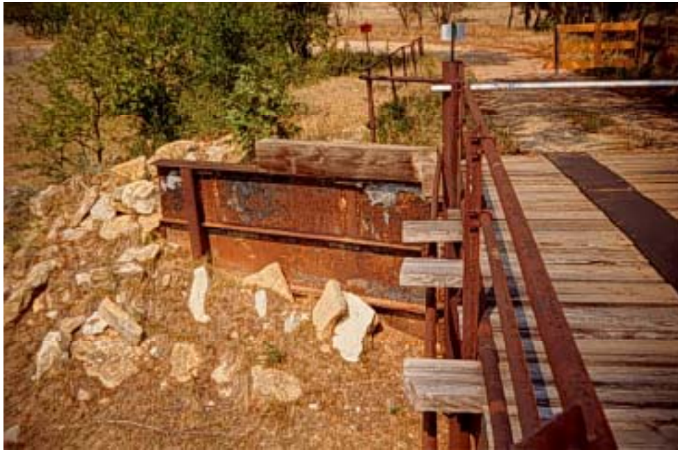
Figure A.31: Metal retaining wall at the north abutment
