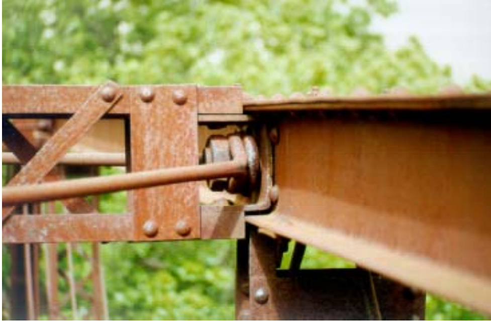
Figure A.16: Top bracing connection
