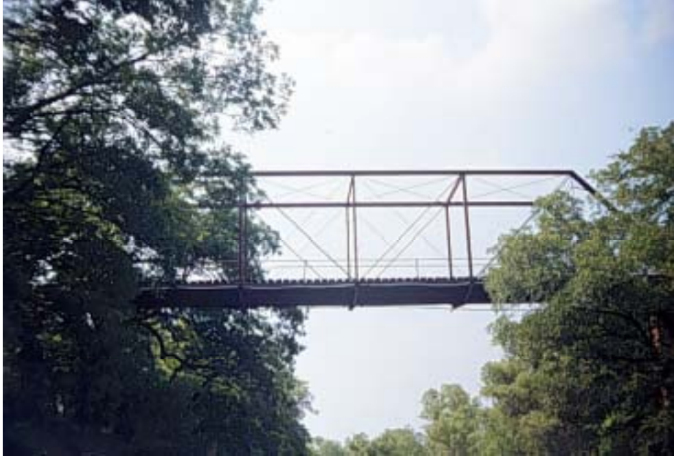
Figure A.3: Main truss span of the bridge
