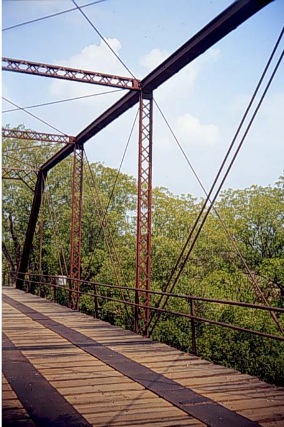
Figure A.6: Downstream truss
