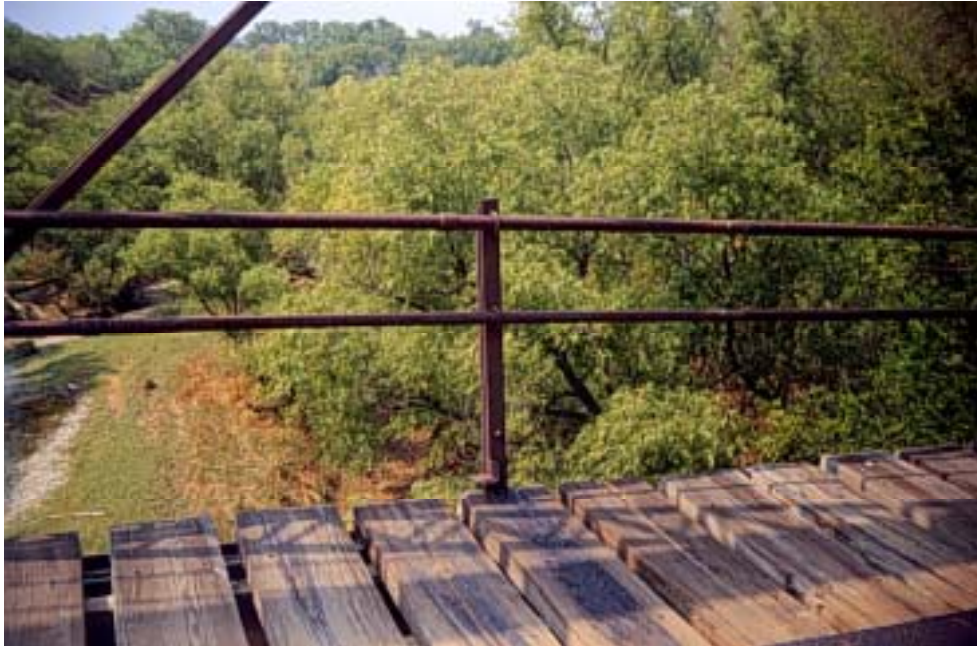
Figure A.23: Metal railing
