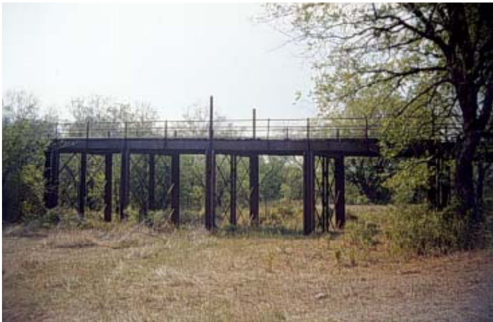
Figure A.4: North approach span
