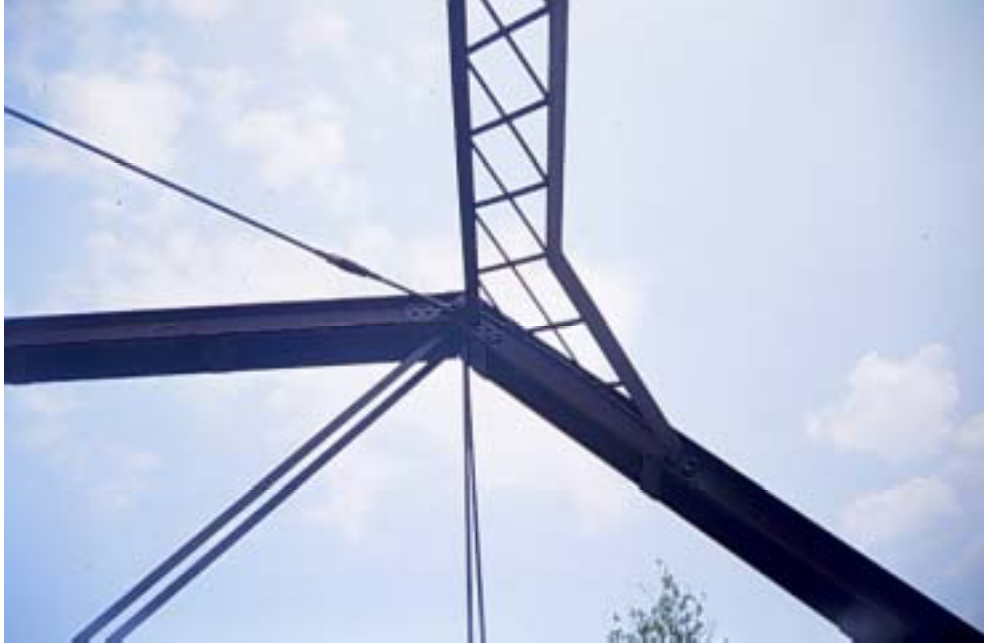
Figure A.14: Upper chord joint U1
