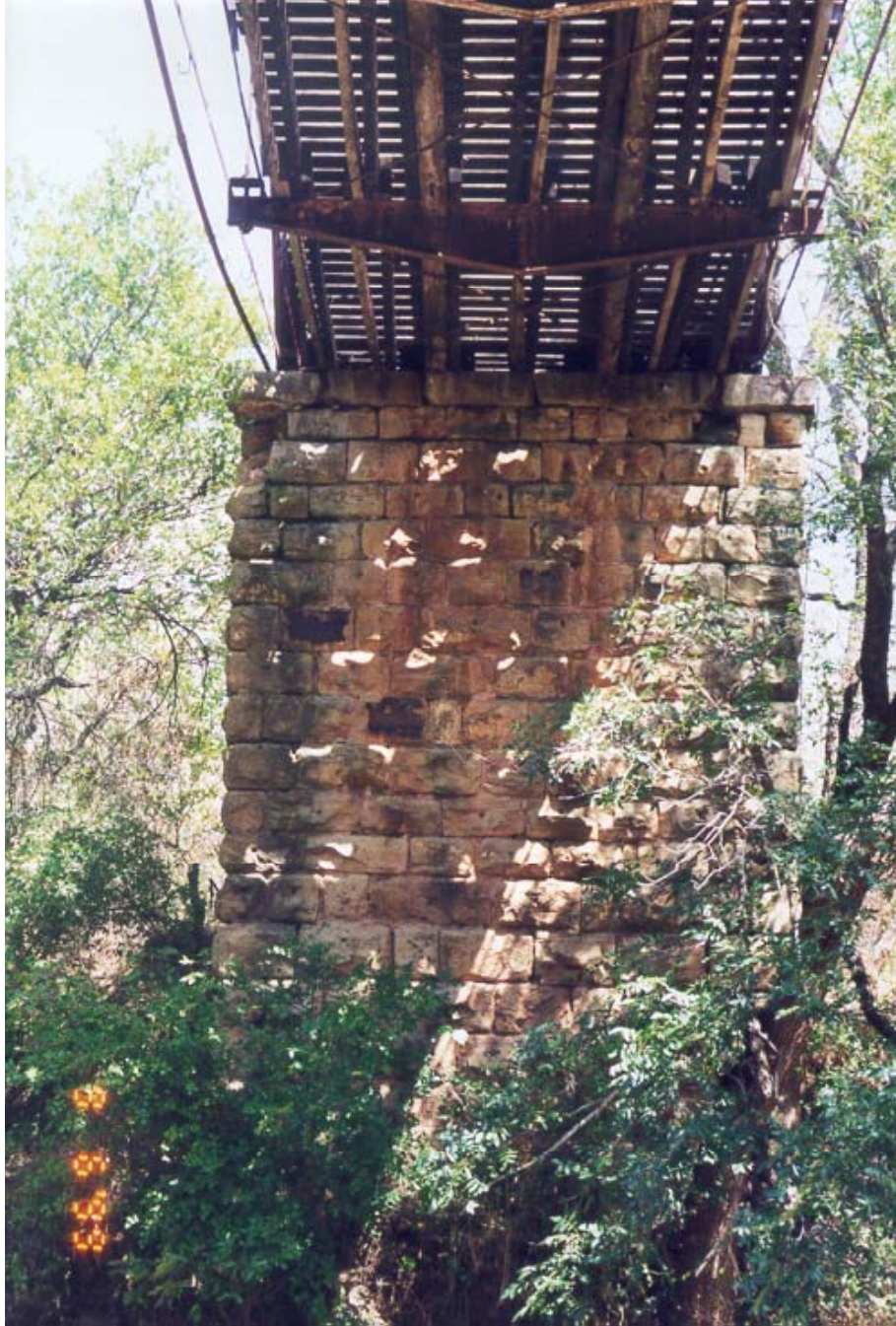
Figure A.19: North stone masonry pier
