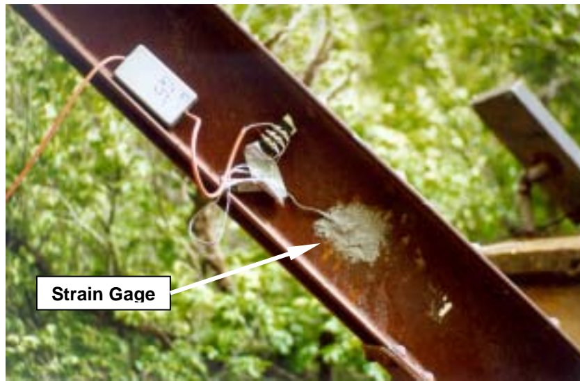
Figure 5.1: Typical strain gage installed on bridge member
