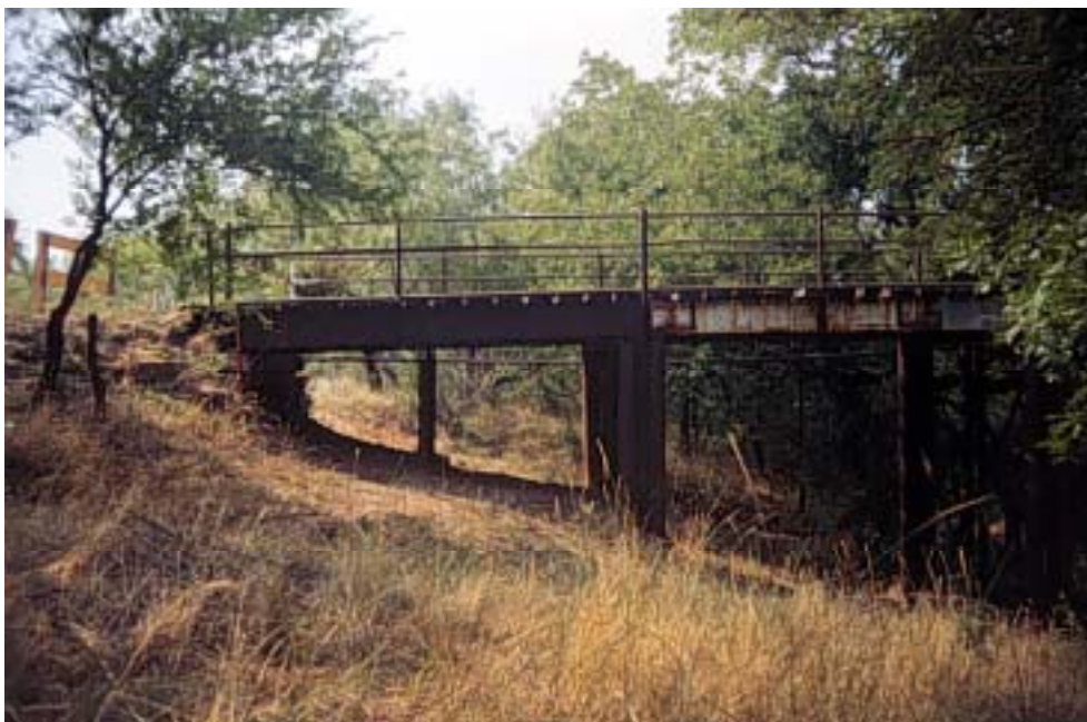
Figure A.2: South approach span
