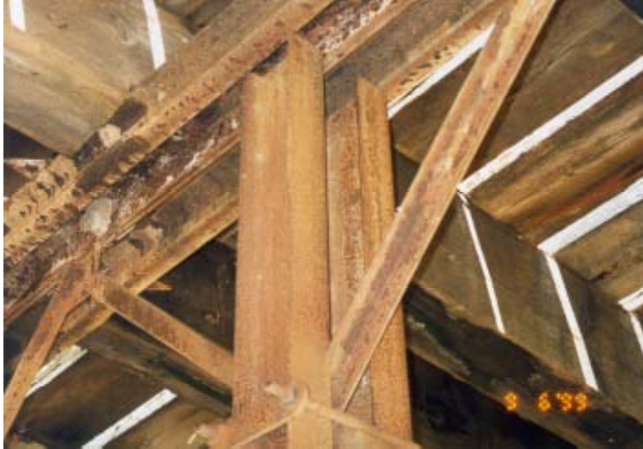
Figure A.36: Metal bent of the north approach span
