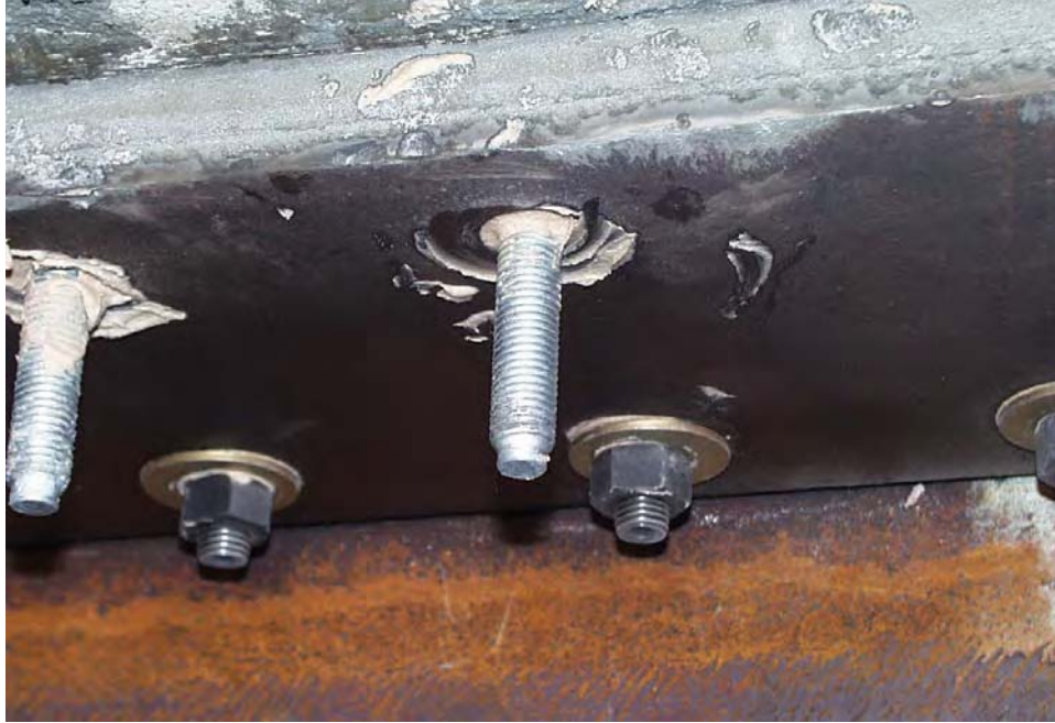
Figure 6.67 Threaded rod installed in slab with epoxy
