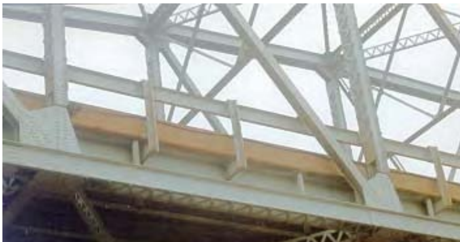
Figure 2.11 Angle attachments of railing to longitudinal stringers
