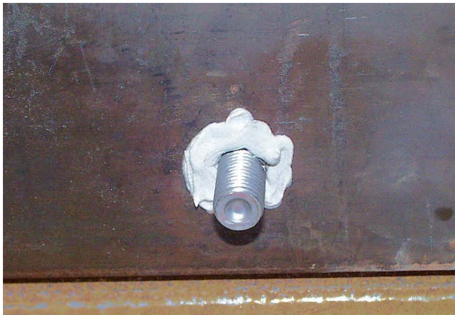
Figure 6.76 Gap filled with HSE 2421 epoxy
