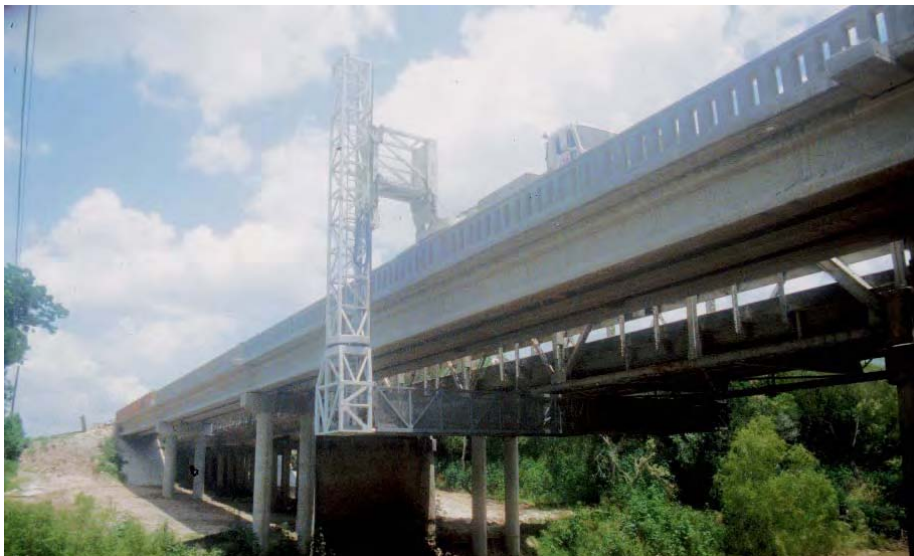
Figure 5.13 Access to bridge deck
