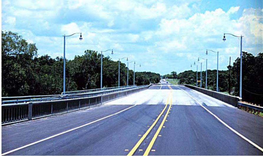
Figure 5.4 View to the north of finished replacement bridge
