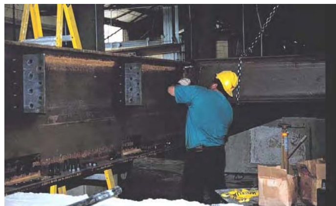
Figure 6.5 Connecting of longitudinal stringer to transverse beam
