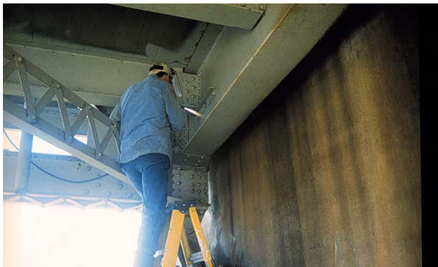
Figure 2.15 Removing the steel sample
