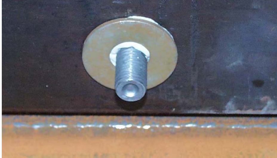
Figure 6.77 Washer covering epoxy filling
