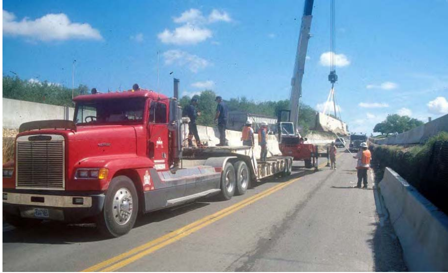
Figure 5.20 Barrier loading to increase axle weight
