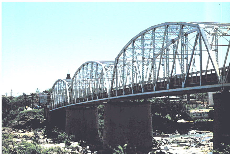
Figure 2.3 Three of the four spans of the Llano Bridge
