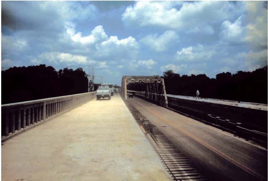
Figure 5.2 Lanes built around the original bridge
