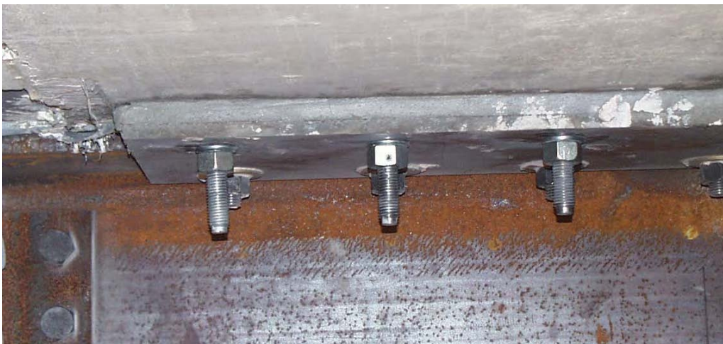
Figure 6.68 Threaded rods bolted to plate
