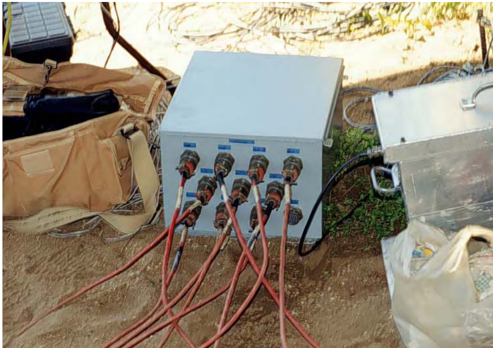
Figure 4.5 CR 9000 data logger
