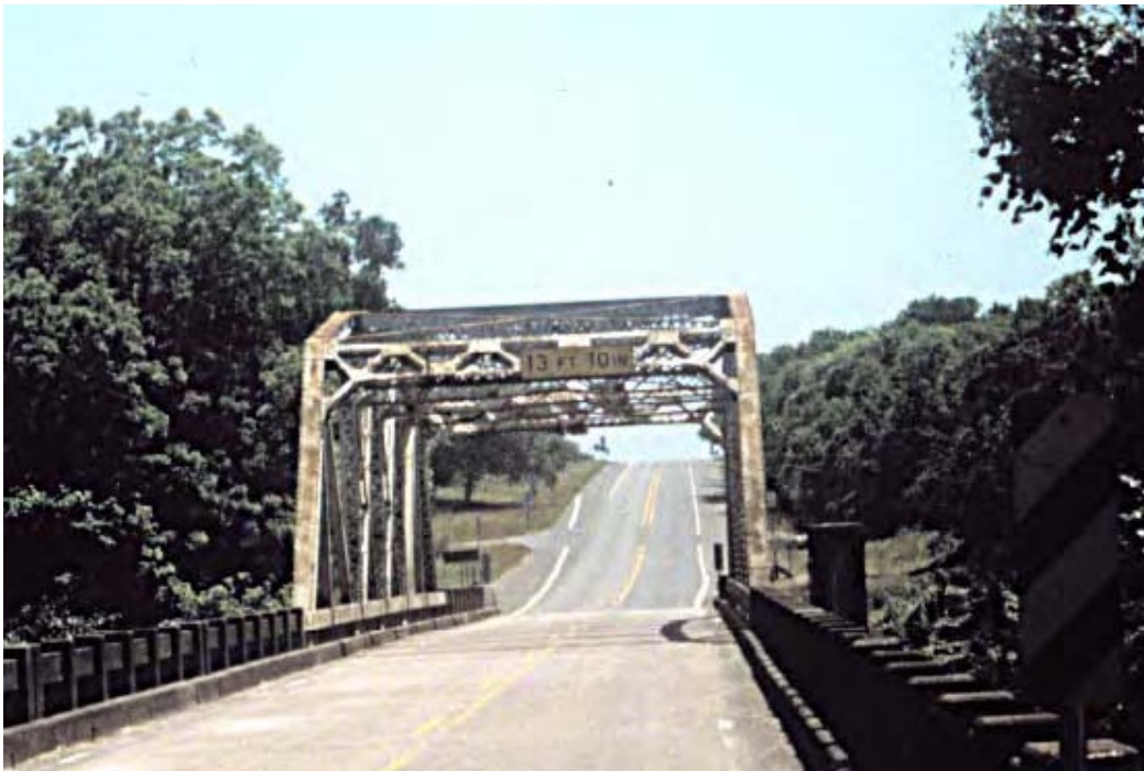
Figure 5.1 Parker truss bridge in Goliad, Texas
