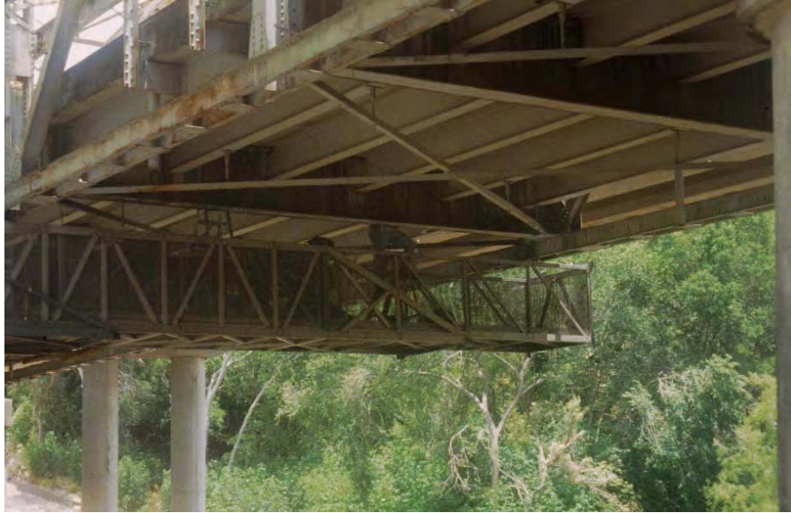
Figure 5.14 Platform extension used to instrument deck
