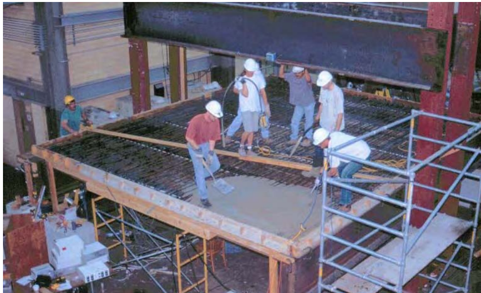
Figure 6.12 Concrete pour and finishing
