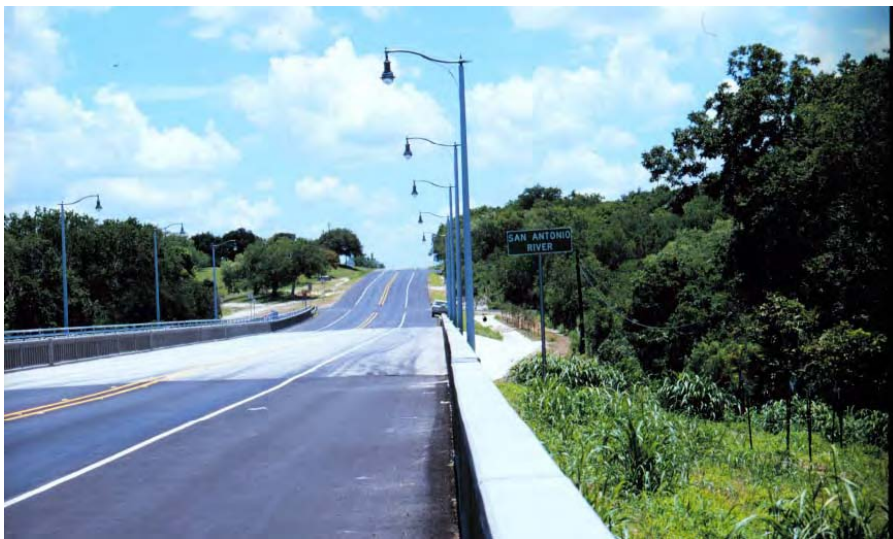
Figure 5.5 South view of finished replacement bridge
