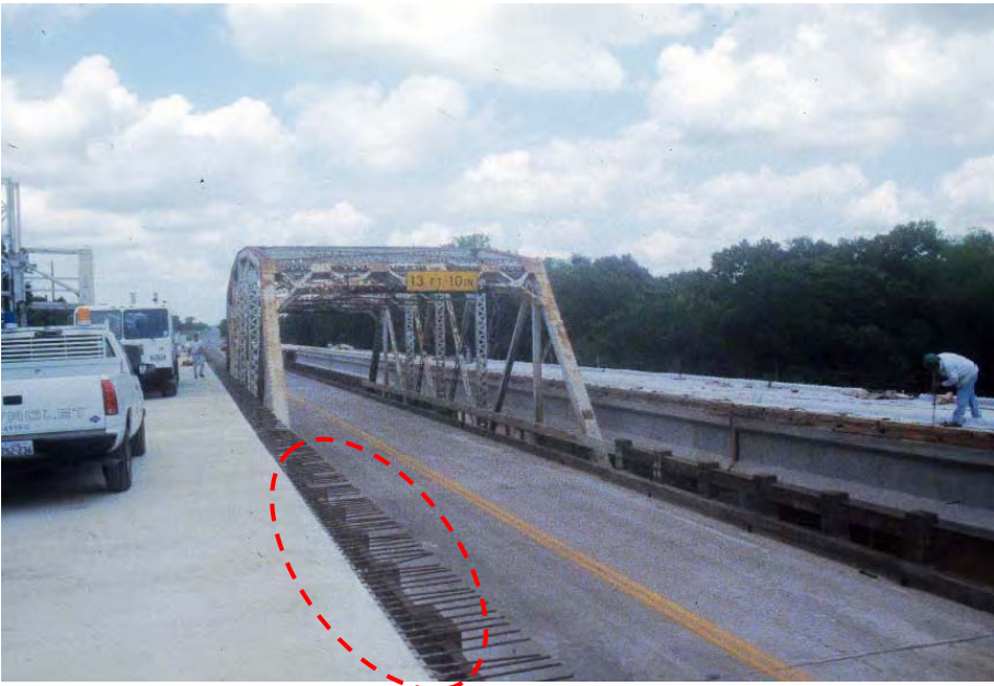
Figure 5.3 Detail showing connecting rebar
