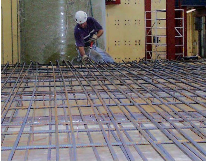
Figure 6.11 Reinforcing bar placement in slab
