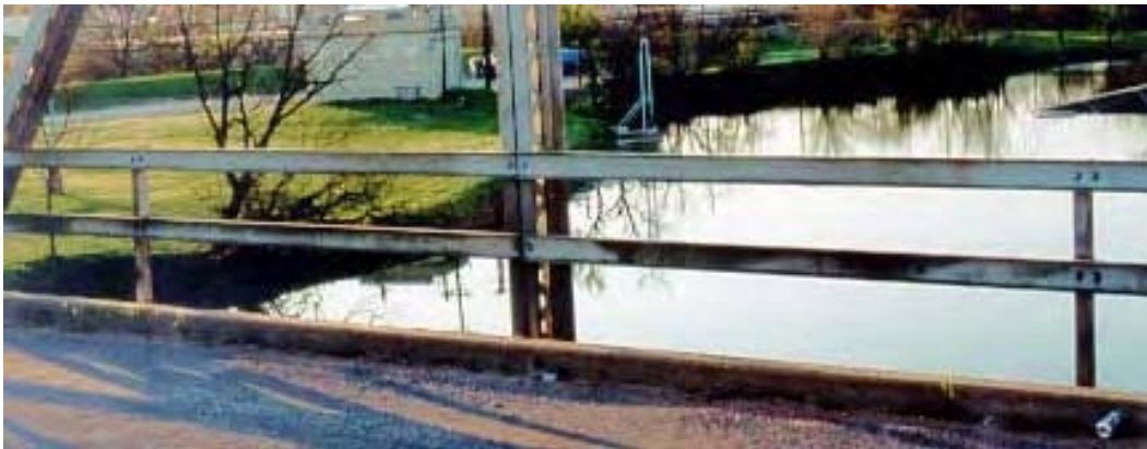
Figure 2.10 Railing attached to vertical and diagonal truss members
