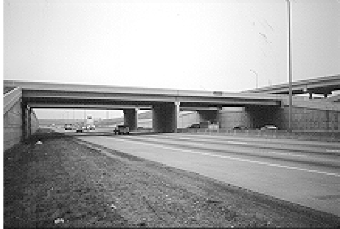
Figure 4.8 A wall substructure unit used for a highway over-pass
