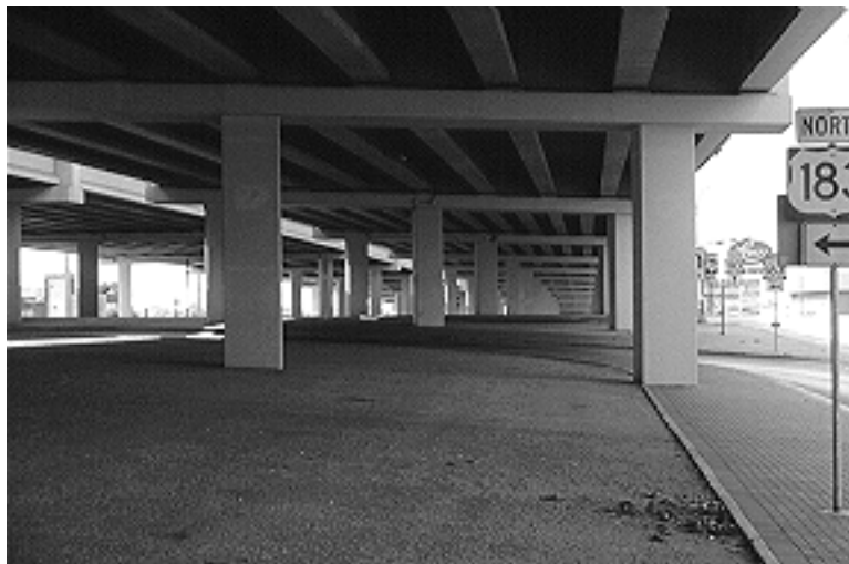
Figure 4.18 Rectangular columns joining a prismatic inverted-T cap
