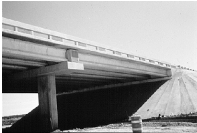
Figure 4.52 Similar formliner patterns used for the railing and the end of the bent cap
