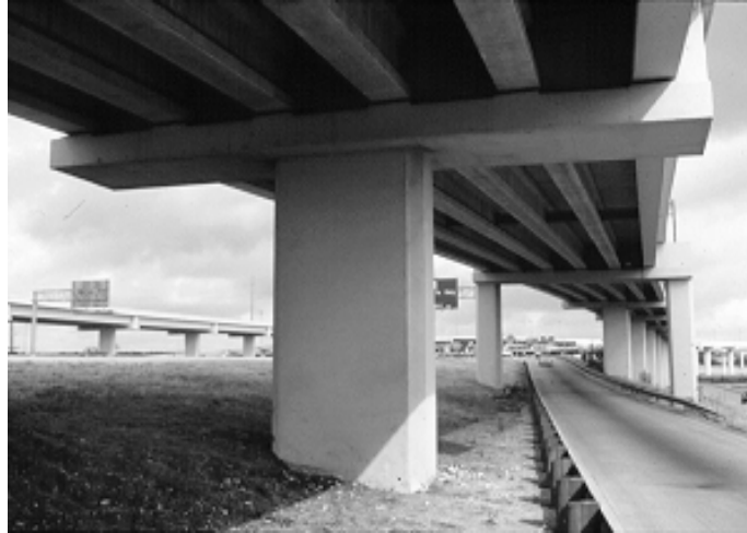
Figure 4.41 Small chamfers on a rectangular column
