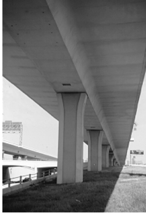
Figure 4.7 Individual columns supporting a single box girder bridge
