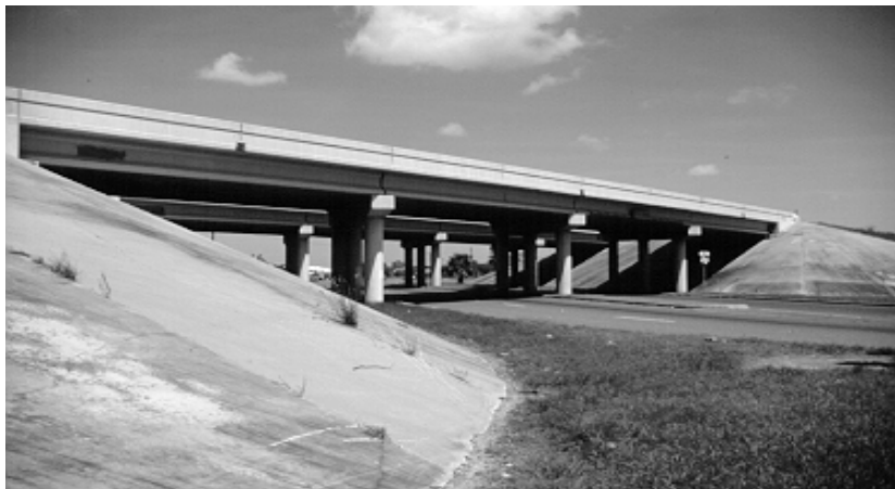
Figure 1.1 A typical standard overpass in Texas
