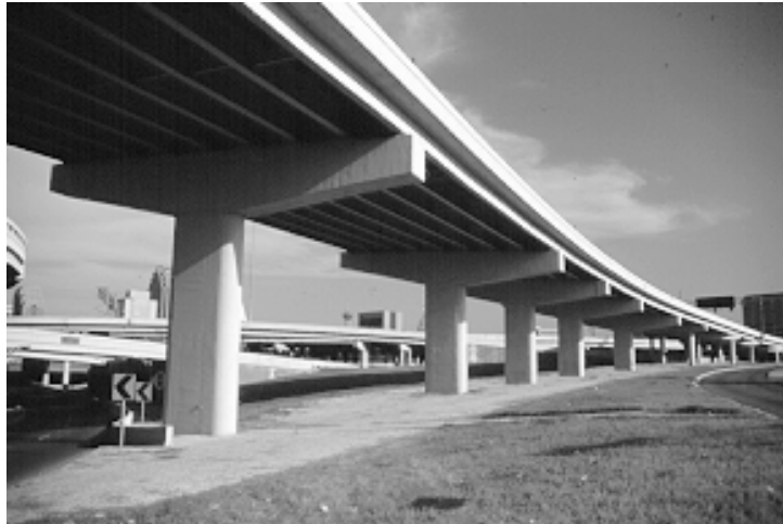
Figure 4.13 Hammerhead bents entirely underneath the superstructure
