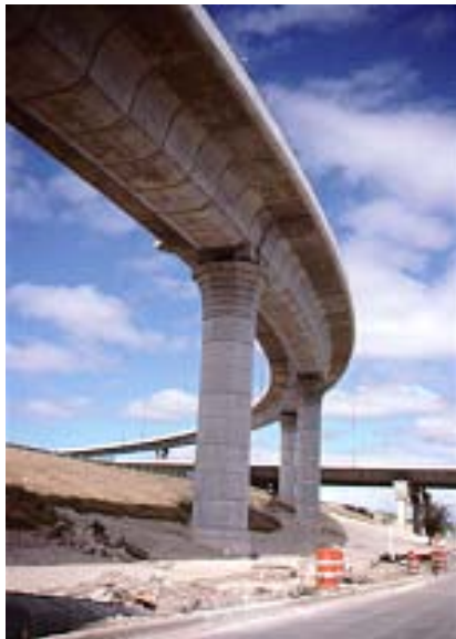
Figure 2.11 Precast segmental piers at US 183 in Austin, Texas
