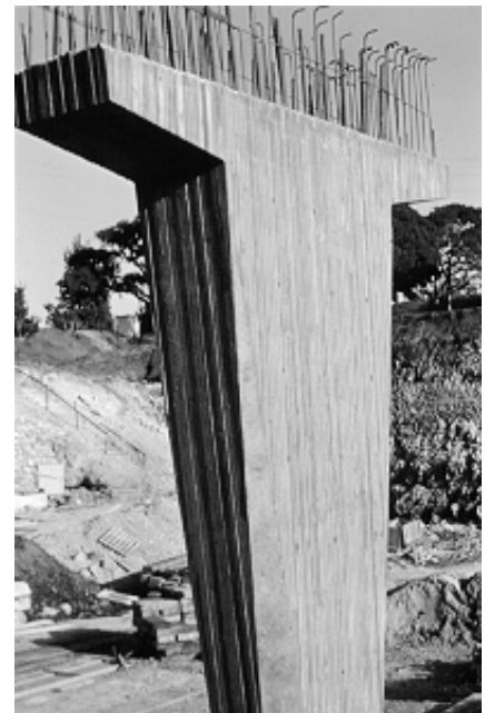
Figure 4.49 Vertical grooves give this wide pier a more slender appearance.
