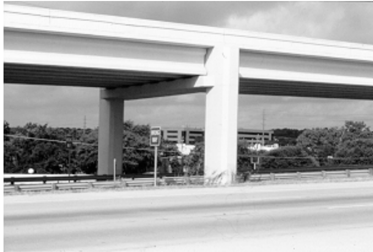
Figure 4.63 Continuation of chamfers from column to bent cap for a well-integrated form
