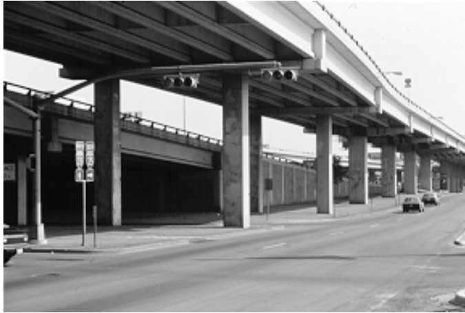
Figure 5.30 View of an I-girder bridge from below
