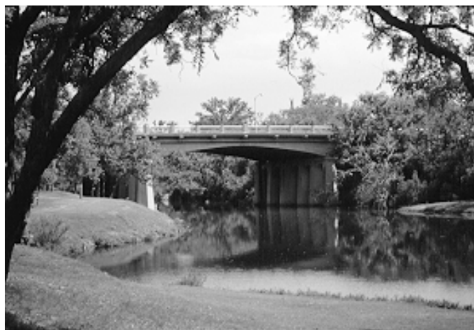
Figure 5.5 One of the older bridges crossing the Concho River in San Angelo
