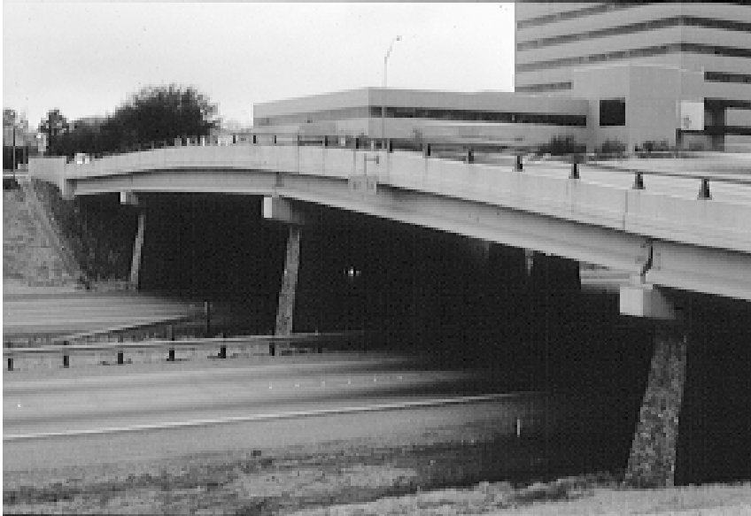
Figure 4.53 Concrete piers formed to appear like stone are foreign to the modern superstructure and urban location.
