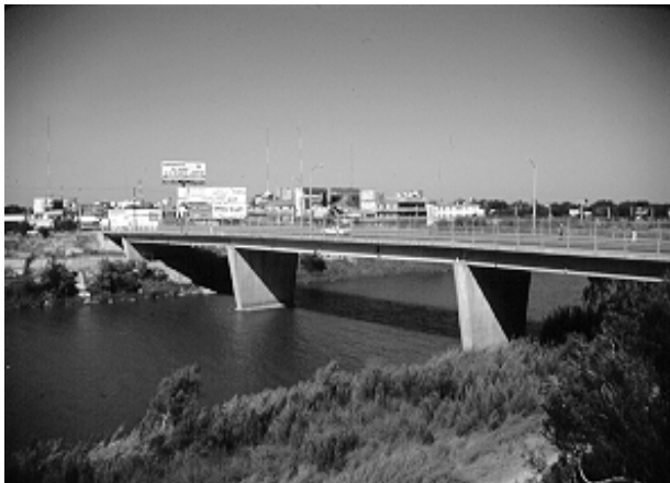
a) Two single-tapered walls with long spans
