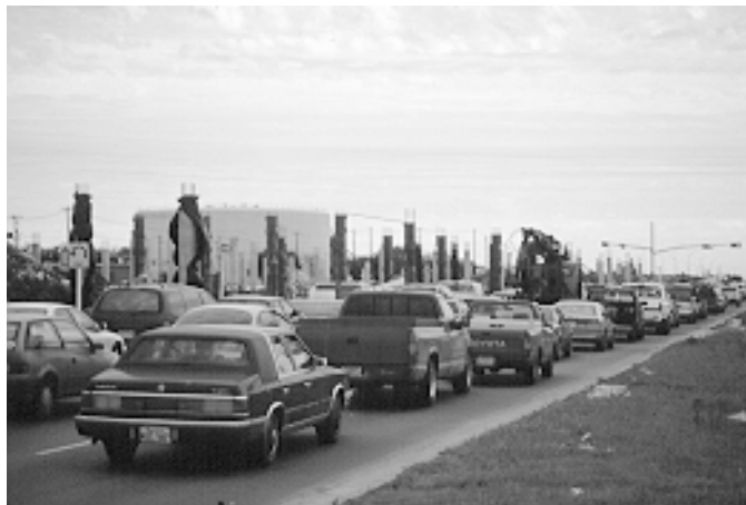
Figure 3.1 Traffic congestion could be relieved sooner with faster highway bridge construction
