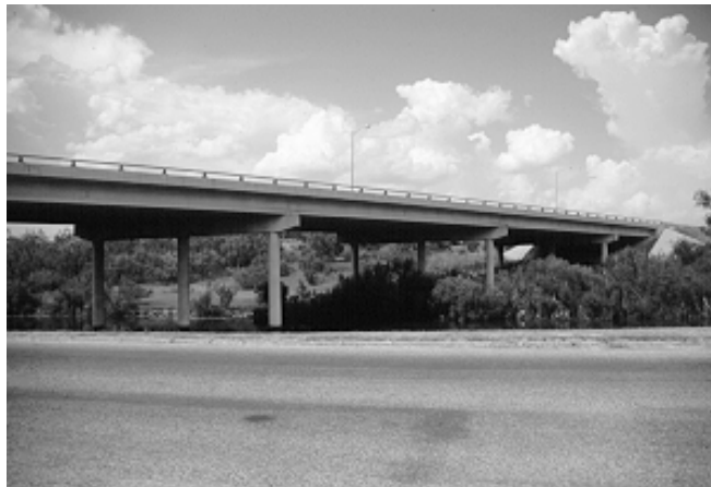
Figure 5.7 A precast prestressed concrete I-girder bridge crossing the Concho River
