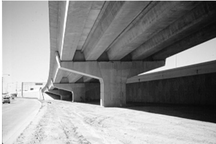
Figure 5.32 View of a U-beam bridge from below
