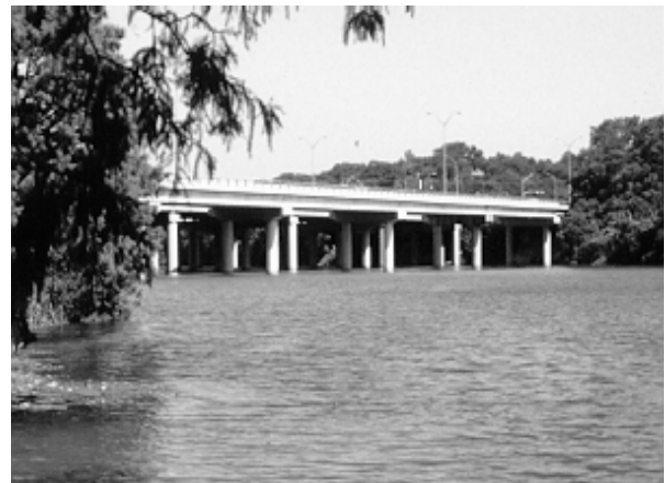
b) multicolumn bents with shorter spans
