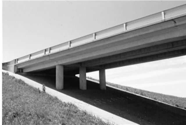
Figure 4.3 Individual columns supporting individual beams
