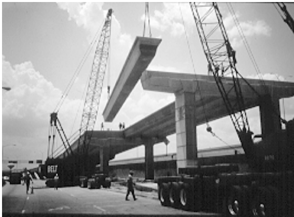
Figure 5.27a Two cranes are required to place precast concrete girders
