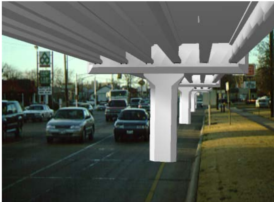
Figure 5.38 Computer rendering of the proposed precast substructure system along the right-of-way on Holliday St. (innermost lane to be removed)
