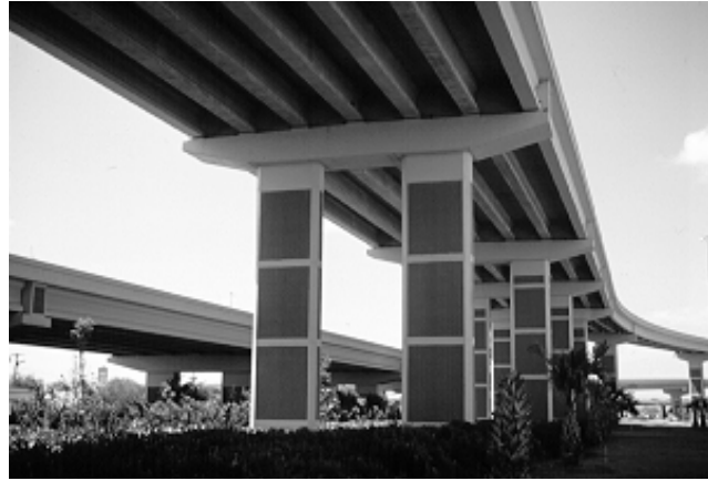
Figure 4.51 Horizontal accents give tall piers a stockier appearance.
