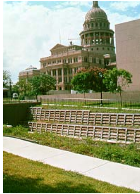
Figure 4.59 Low concrete retaining walls colored to match local building materials
