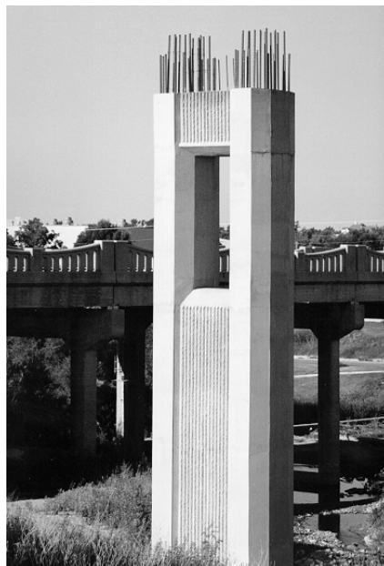
Figure 5.19 A windowed pier under construction for US 67
