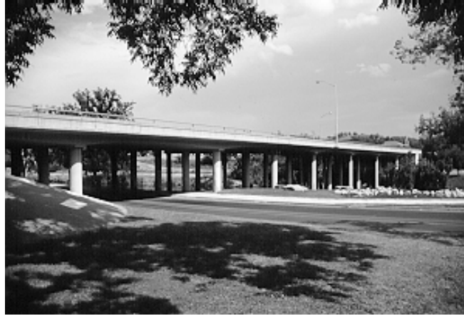
Figure 5.6 A cast-in-place slab bridge crossing the Concho River
