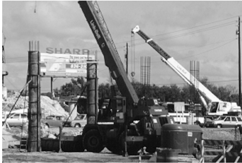
Figure 1.3 Extensive on-site equipment for cast-in-place multicolumn bents
