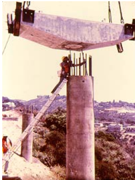
Figure 2.9 Placement of a precast pier cap on a to cast-in-place column
