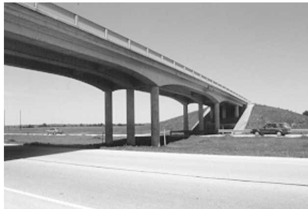
Figure 4.4 Individual columns supporting individual cast-in-place continuous beams
