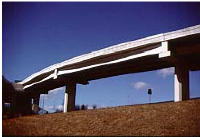
Figure 5.31 Scalloped shadows on curved bridges made up of straight girders
