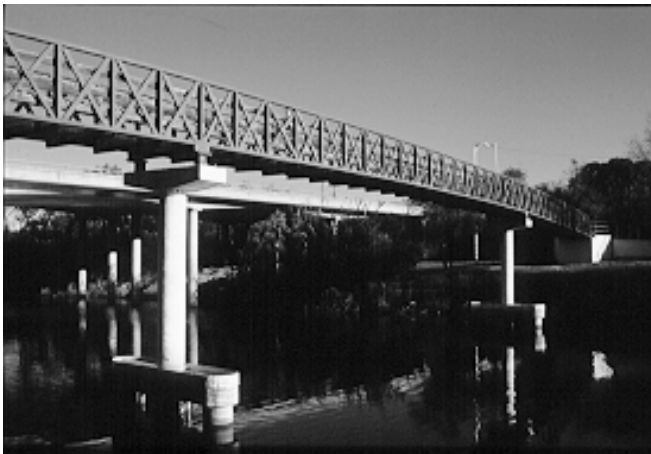
Figure 5.8 One of many pedestrian bridges crossing the Concho River
