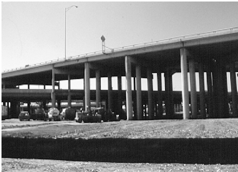
Figure 4.16 Cluttered multicolumn bents create “forests” of columns
