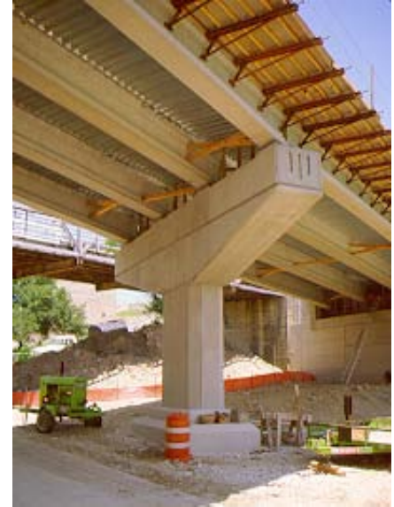
Figure 4.47 An attractive pier with a rubbed concrete finish
