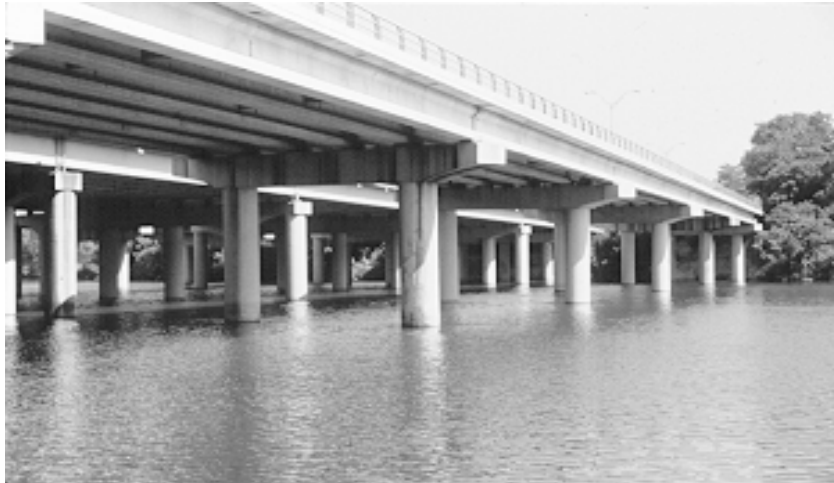
Figure 4.2 Typical cast-in-place substructure system in Texas
