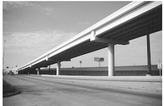
Partially integrated bent caps with rectangular columns and prismatic caps (a) or with round columns and prismatic caps (b)
