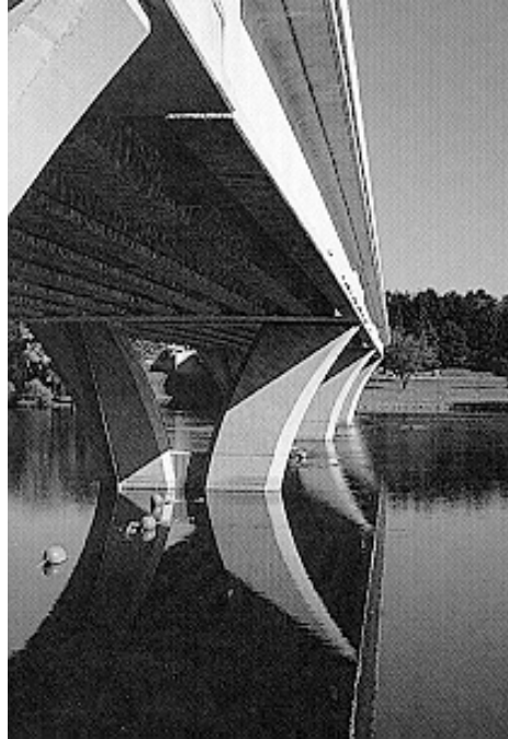
Figure 4.11 Cast-in-place substructures can be curved or tapered
