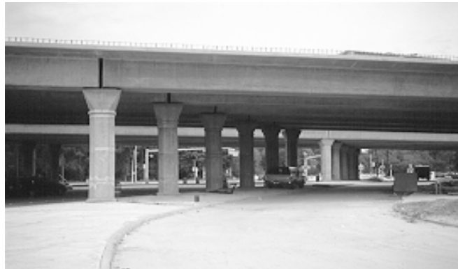
Figure 2.12 Precast piers for a grade separation in Houston, Texas
