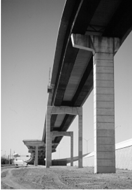
Figure 4.50 Horizontal grooves make concrete appear like masonry.
