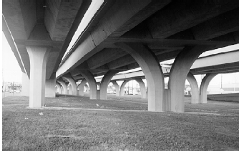
Figure 1.4 An attractive cast-in-place substructure
