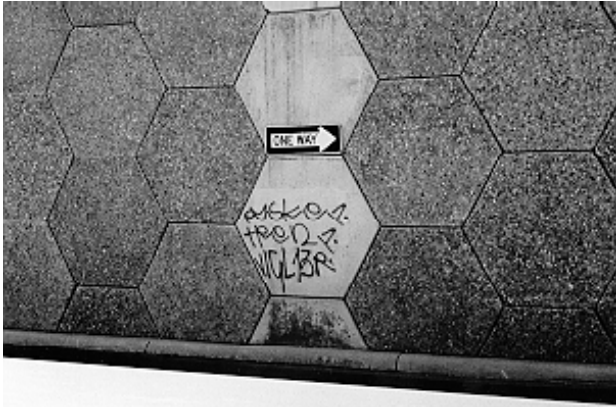
Figure 4.46 Exposed aggregate finishes may be less likely to attract graffiti than plain concrete
