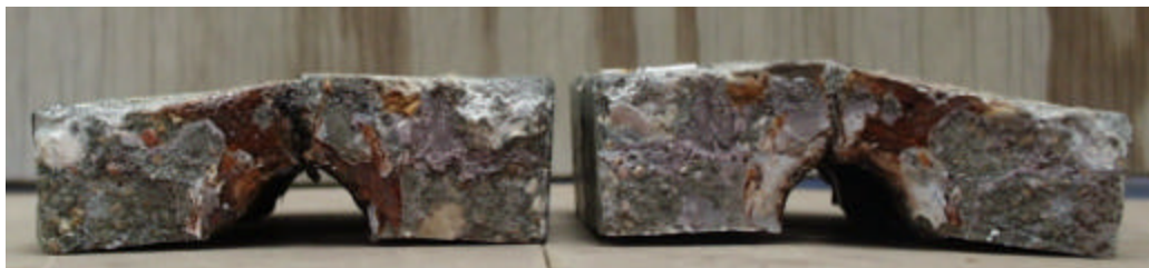
Figure 4.24 Incompletely Filled Epoxy Joint (SE-S-M-CI-1).
