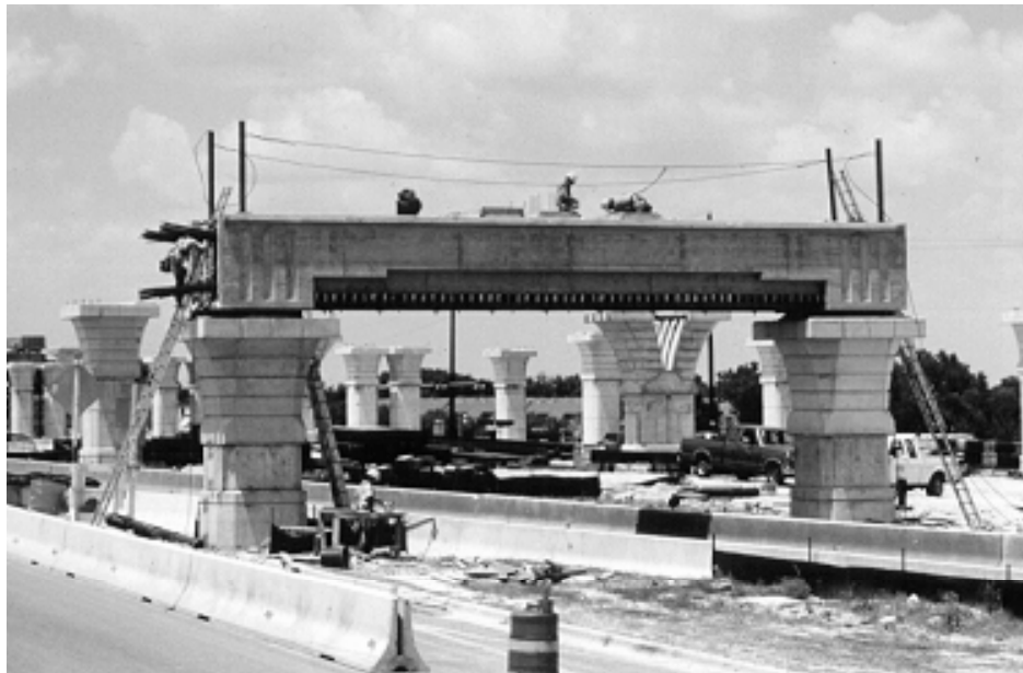
Figure 1.7 - Post-Tensioned Straddle Bent
