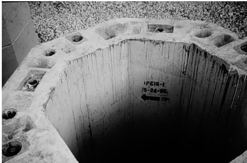
Figure 1.5 - Precast Bridge Pier Segment Close-Up
