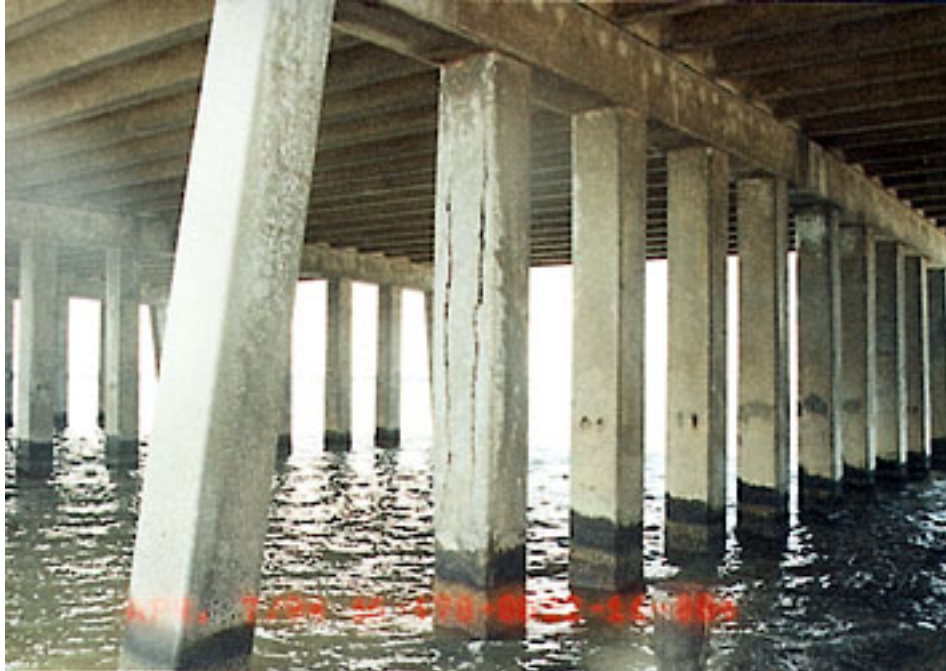
Figure 2.11 - Face Splitting of a Bridge Column in Corpus Christi
