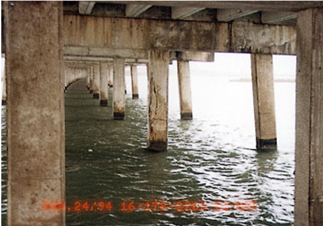
Figure 2.10 - Horizontal Splitting of the Upper and Lower Reinforcement in a Typical Bent Cap
