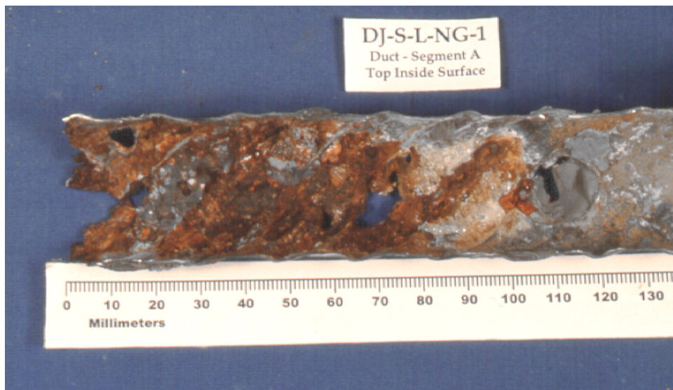
(b) Inside Surface of Duct (joint location at left end)
