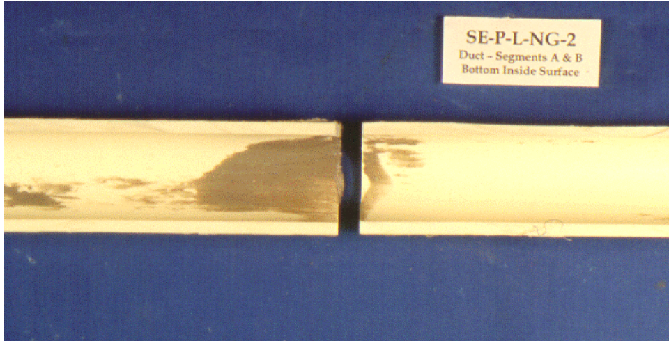
Figure 4.17 – Joint Epoxy Smeared Inside Plastic Duct During Swabbing
