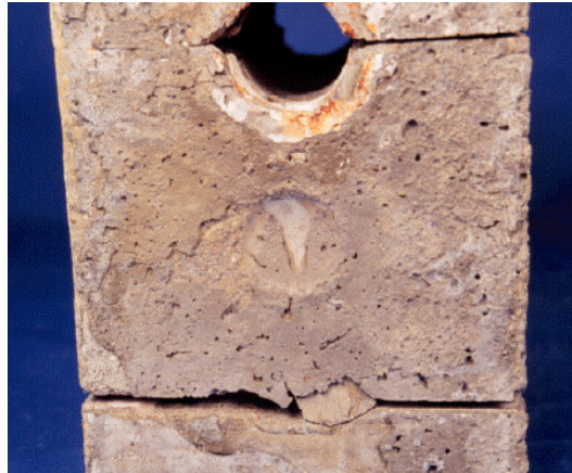
Figure 4.15 – Grout Infiltration Into Joint: Specimen DJ-S-L-CI-1
