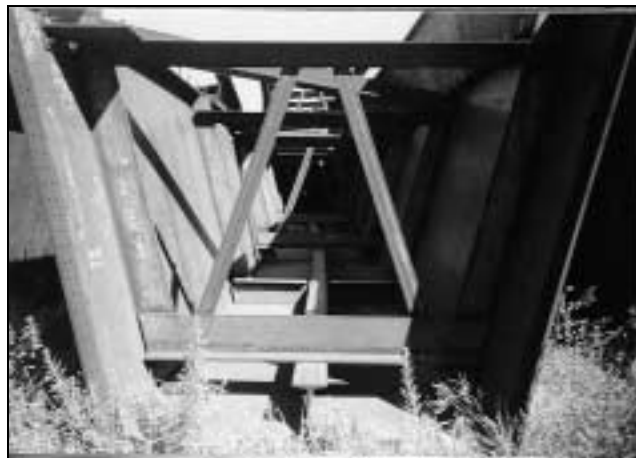
Figure 1.2 Cross Section of U-Shaped Girder Segment (Gilchrist, 1997)
