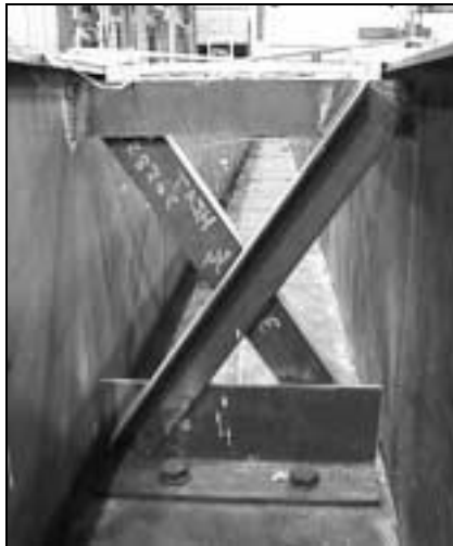
Figure 3.7 X-Brace at Support Location
