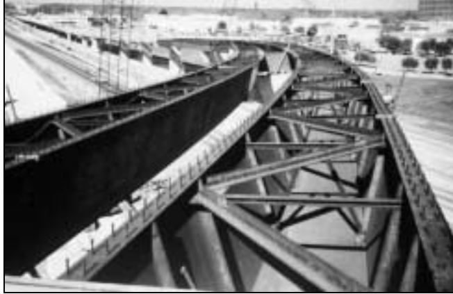
Figure 1.3 U-Shaped Girders During Erection (Gilchrist, 1997)
