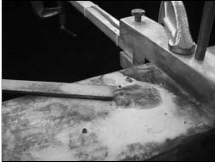
Figure 3.17 Welded Brace Connection Detail
