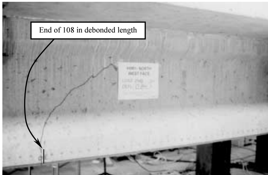
Figure 7.38: Test H9R-C-96H—Crack at End of 108 in (2.74 m) Debonded Length
