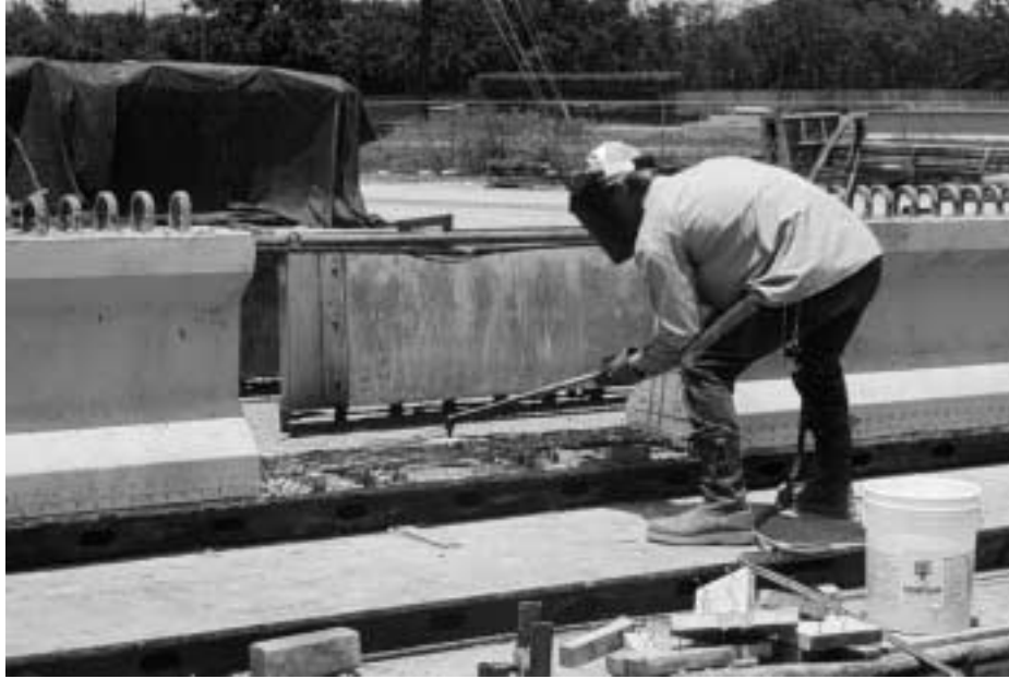
Figure 3.18: Transfer of Prestress by Flame-Cutting
