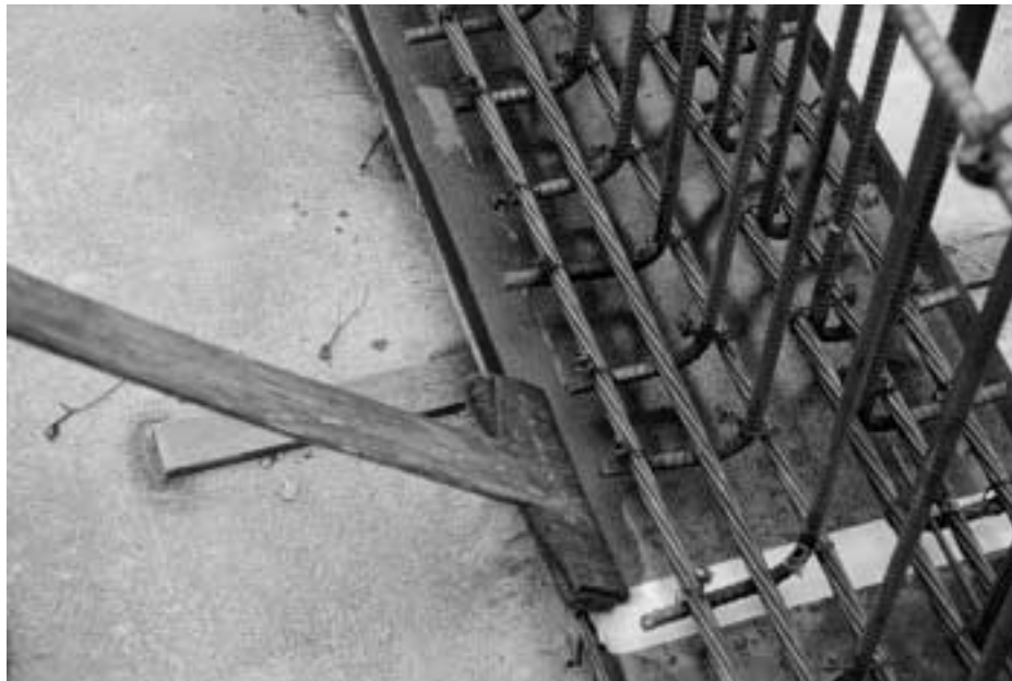
Figure 3.14: Distributing Form Release Agent over Soffit Form Surface
