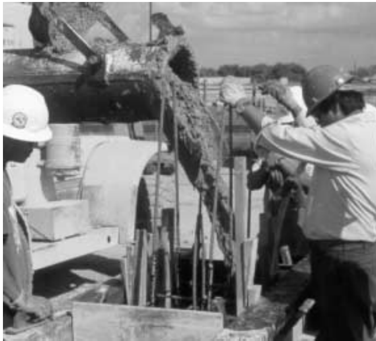
Figure 4.3: Casting Pull-out Test Block
