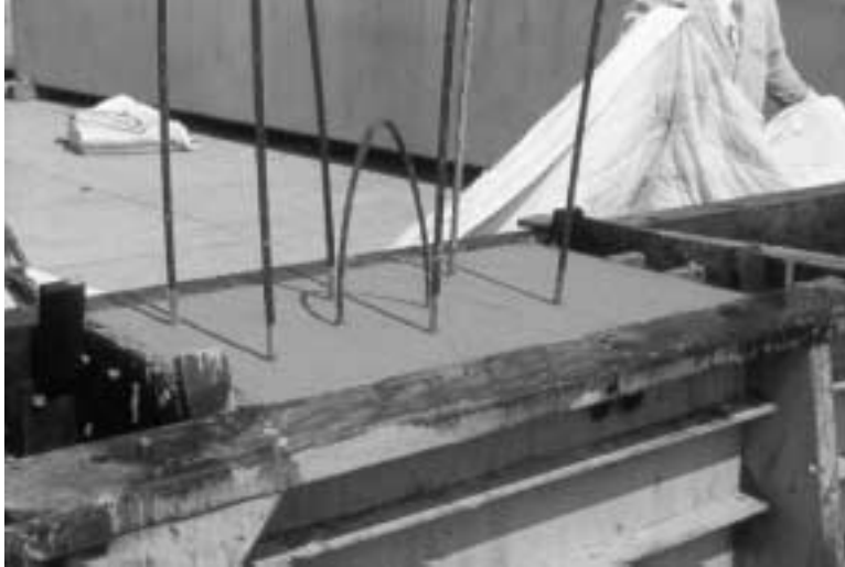
Figure 4.4: Finished Pull-Out Test Block
