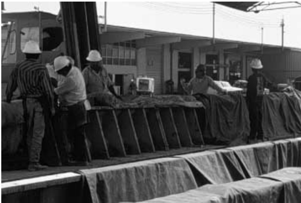
Figure 3.17: Covering Precast Beams with Curing Blankets
