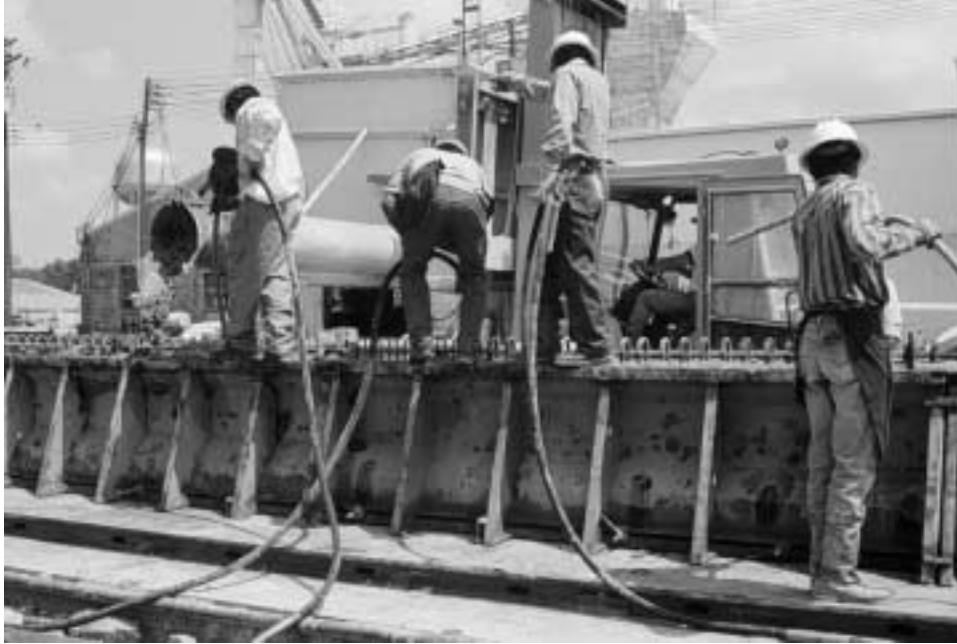
Figure 3.16: Casting and Vibrating Precast Beam Concrete
