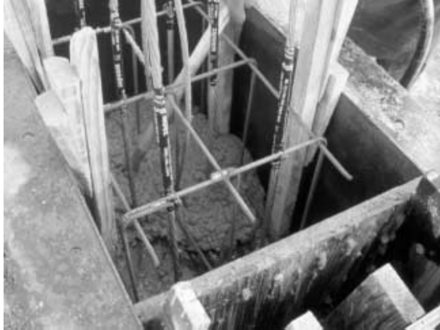
Figure 4.2: Pull-out Test Block at Onset of Casting
