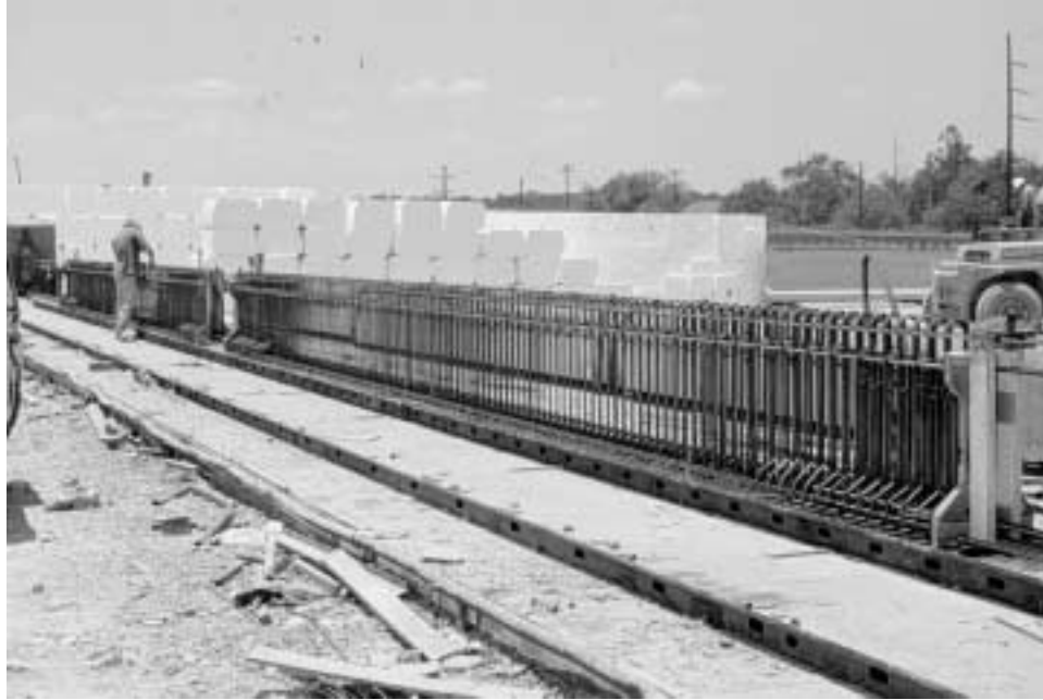
Figure 3.12: Reinforcement for Pair of I-Beams
