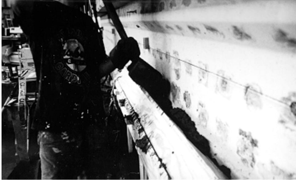
Figure 6- 68 Placement of 928 Fast Patch — final phase of repair — Steck girder
