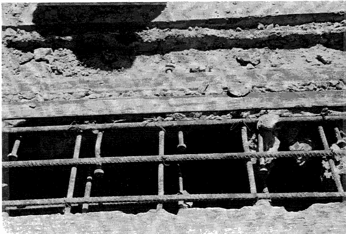
Figure 9 Close placement of the reinforcing steel to the rail
