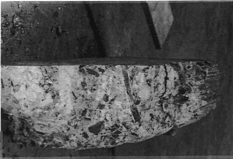
Figure 55 Cross-section of roadway section after removal of stud
