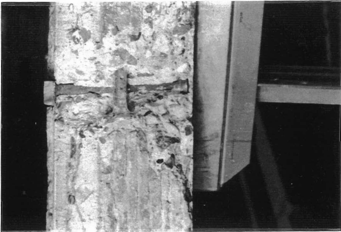
Figure 50 Excavation of study in roadway section
