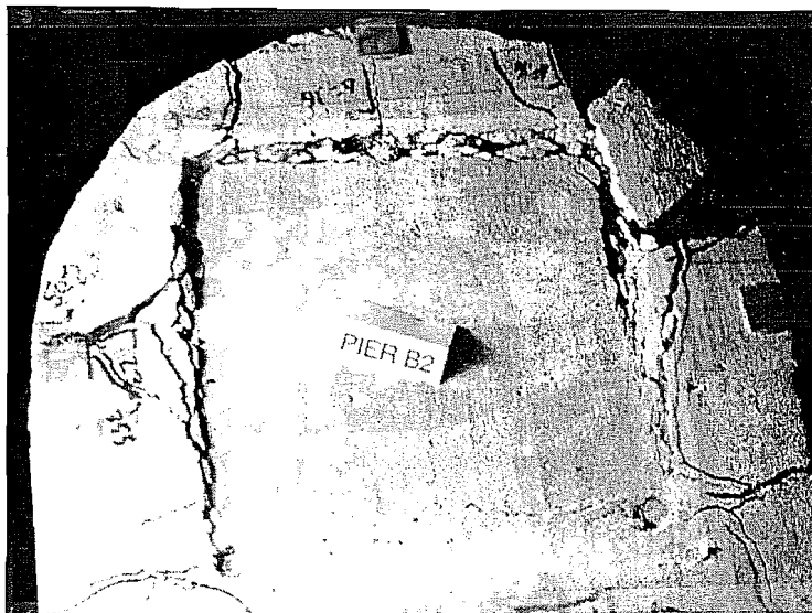
Figure 11- 22 Punching of the base plate into Pier B2-2
