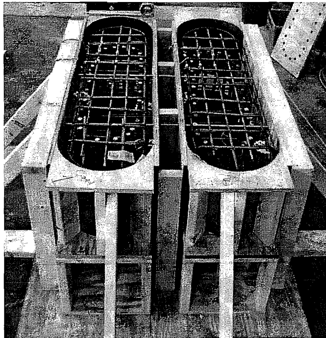
Figure 2.13 Placement of Reinforcing Cages in forms
