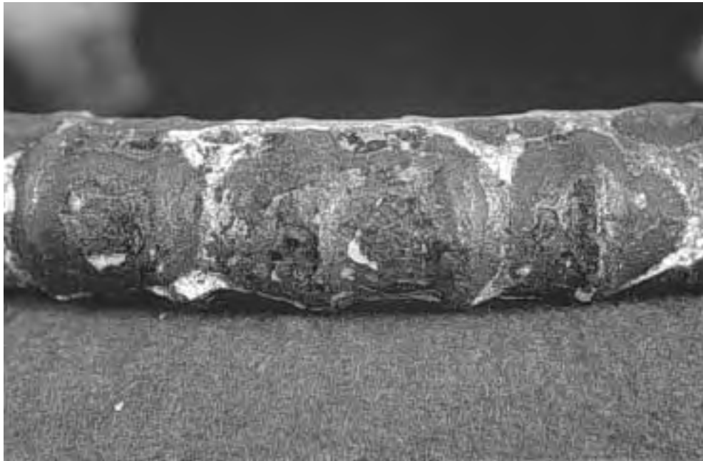
(b) Bar with unpatched damage at outside bend.
