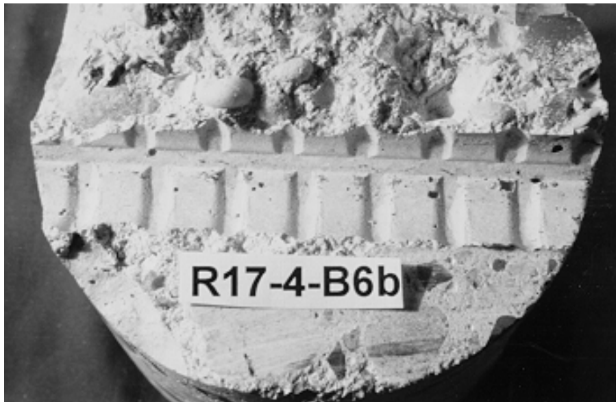
(b) Air voids under bottom bar
