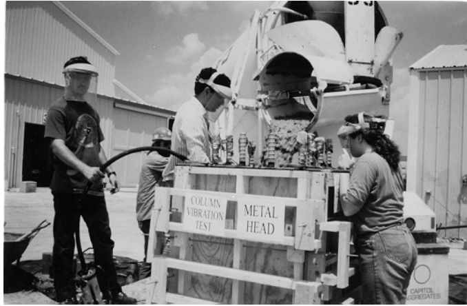
Figure 2.7 Placing concrete in column form
