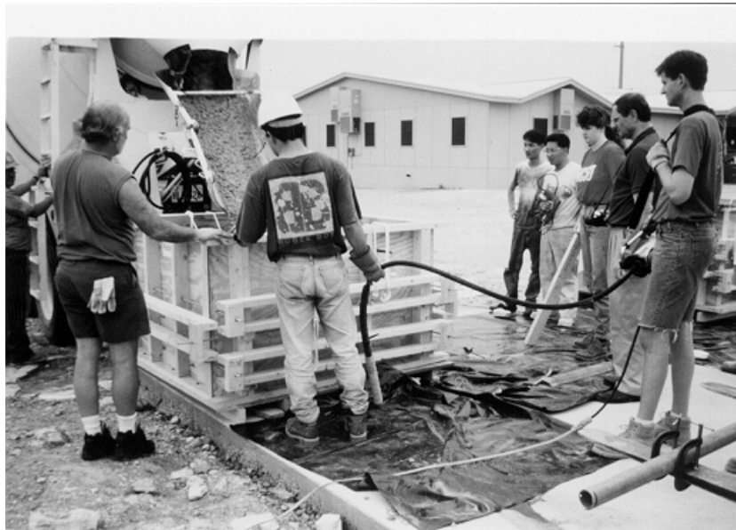
Figure 2. 11 Placing concrete in footing form
