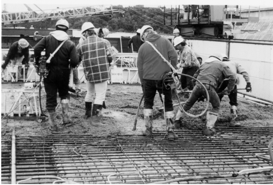
Figure 1.3 Consolidation of concrete in bridge deck
