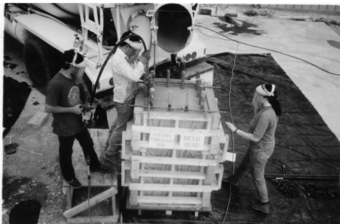
Figure 2.8 Consolidating column specimen
