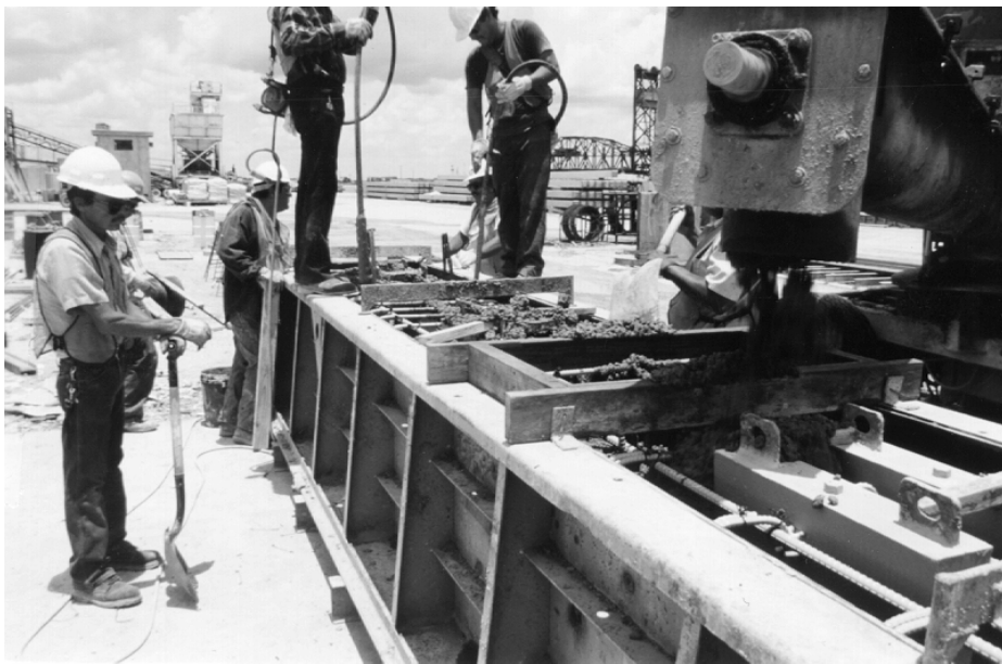
(b) Vibration of concrete in precast element
