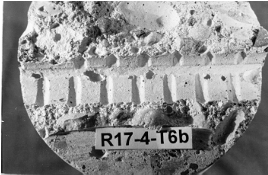
(a) Air voids under top bar
