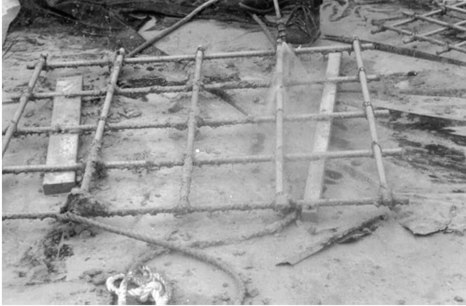
Figure 2. 14 Washing footing reinforcement mat
