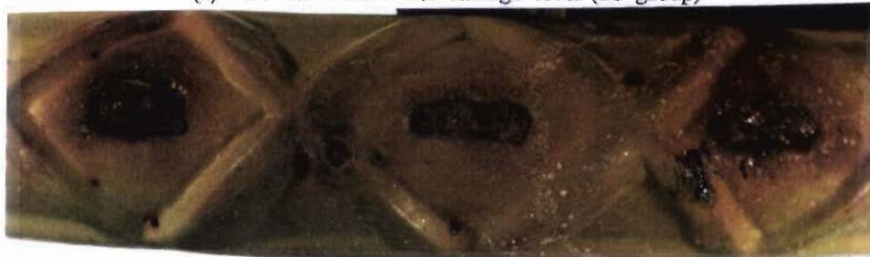
(b) #8 bars with &gt; 2% damage level (B10 group)
