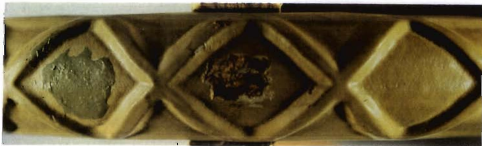
Figure 5.5 Deterioration of exposed areas on #8 bar with cross deformations.
