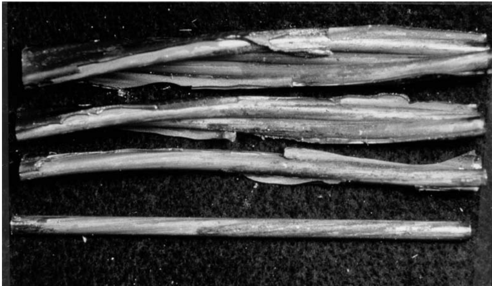
Figure 8-29 Interstitial corrosion of epoxy-coated strand (not filled)
