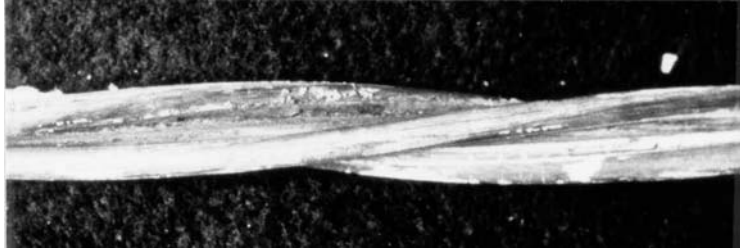
Figure 8- 22 Corrosion in the interstitial space of bare strand
