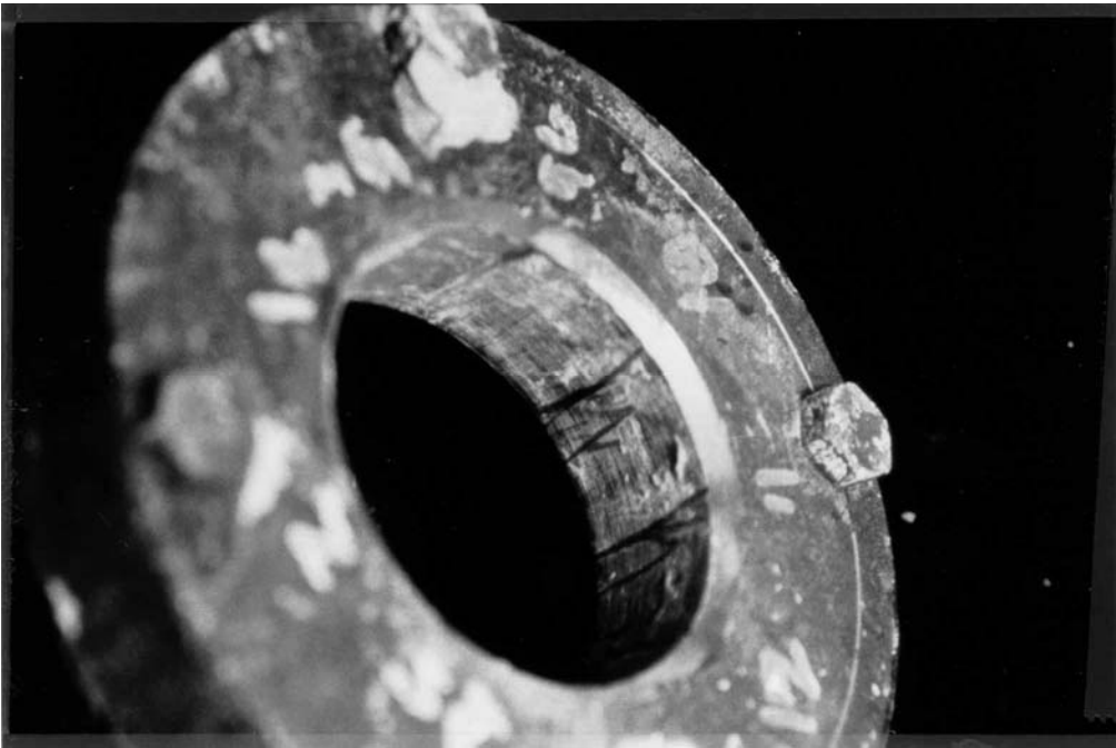
Figure 8- 27 Typical condition of inside face of deviator ring
