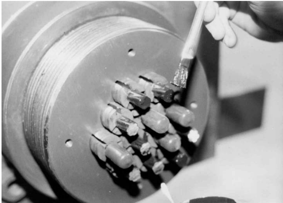
Figure 8-6 Repair of cut ends of epoxy-coated strands
