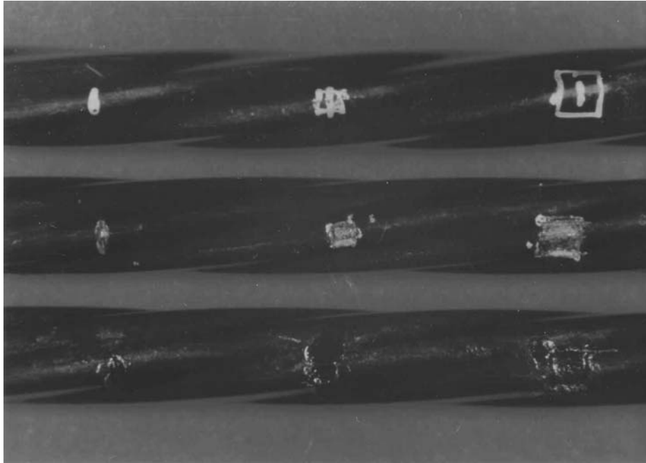
Figure 8- 5 Three sizes of damage made to epoxy coating: Cut, 3.2-mm square and 6.4-mm square (middle). Repaired damages shown at bottom
