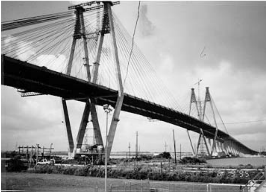
Figure 1-1 Houston Ship Channel Crossing
