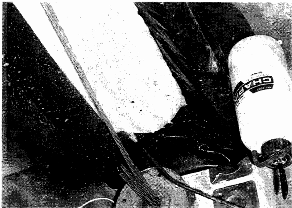
Figure 3.20 Application of lubricant
