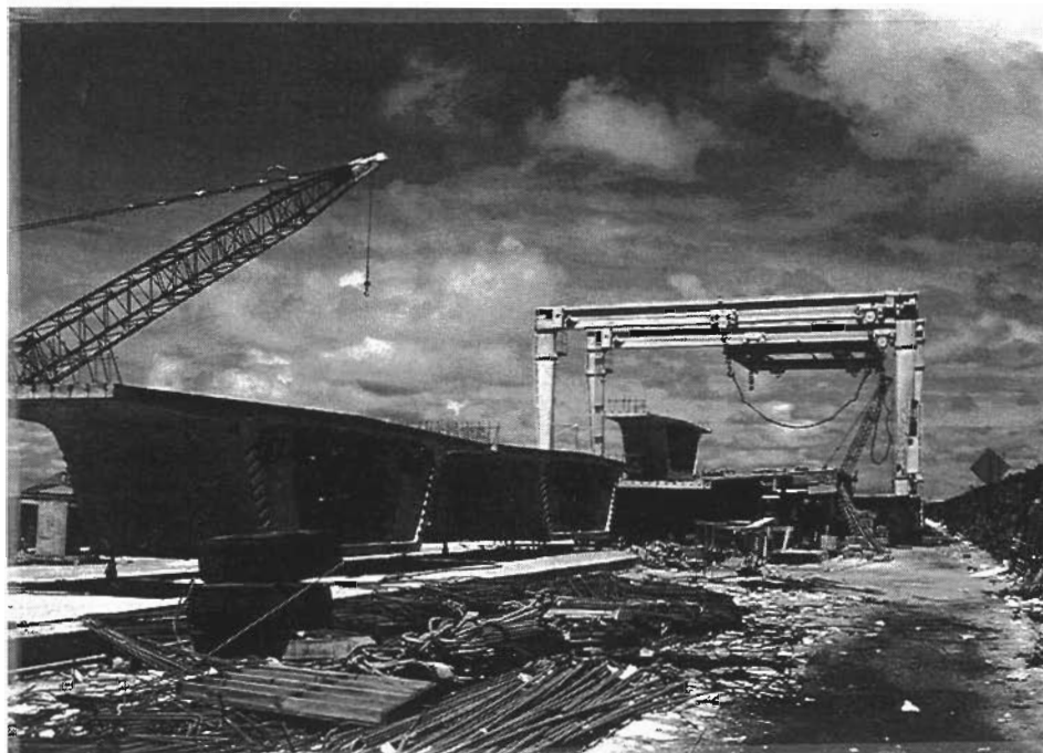
Figure 1.1 Segment fabrication yard.
