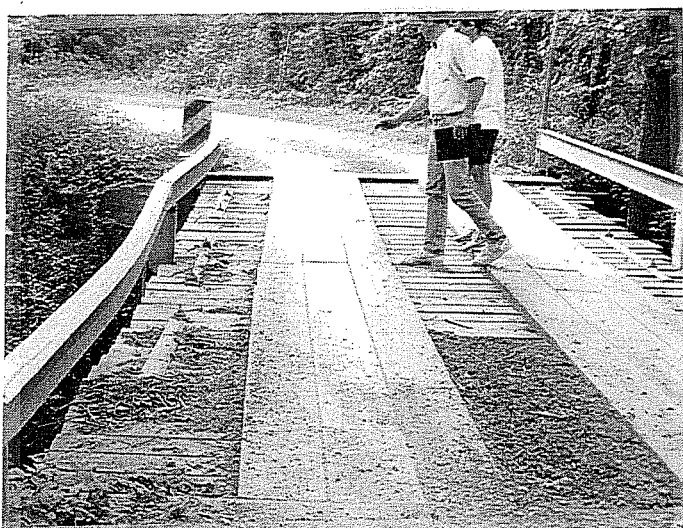
Figure 5.14 Bastrop County Bridge AA-0233-01.
