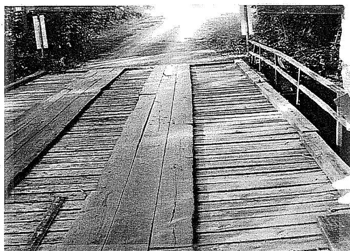
Figure 5.15 Bastrop County Bridge AA-0237-01.
