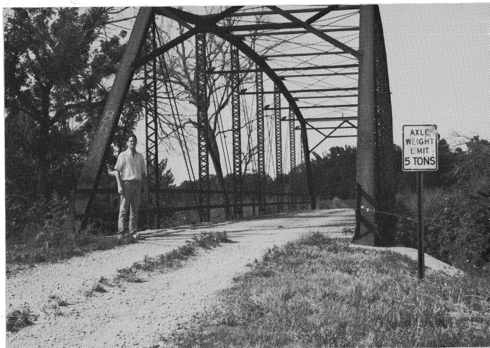
Figure 1.1 Typical off-system bridge with timber deck
