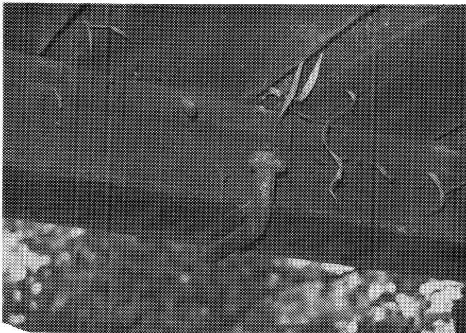
Figure 5.3 Typical J-Bolt Connection at Exterior Stringer
