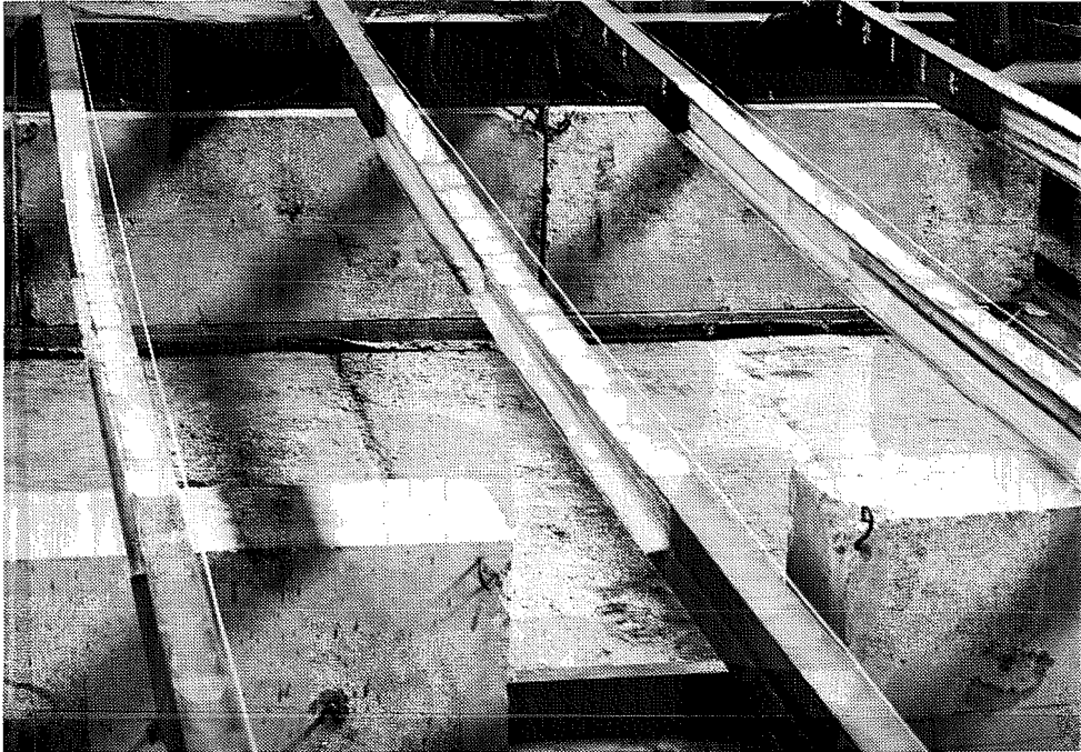
Figure 4.16a Deformed beams after the test.
