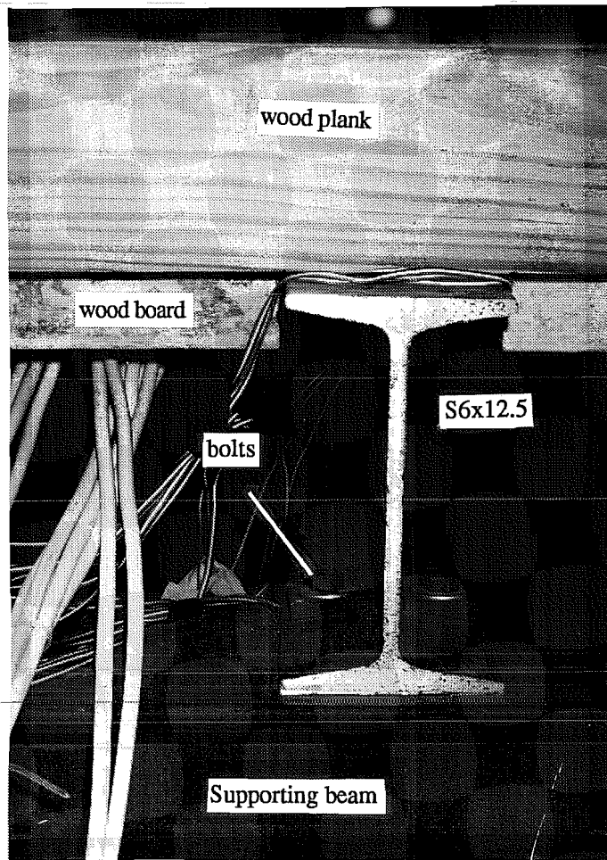
Figure 3.9 Photograph of end support detail.
