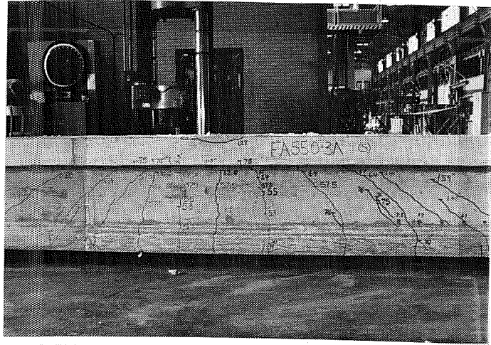
Figure 4.10 Test FA550-3A: Typical Flexural Cracking
