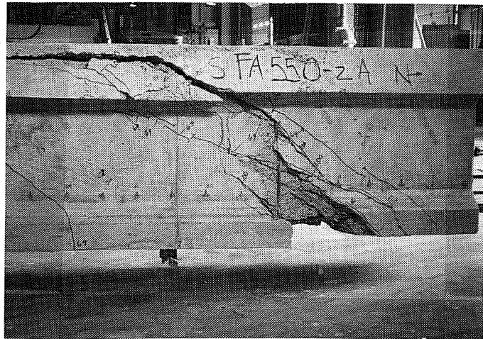
Figure 4.13 Photograph of FA550-2A Explosive Shear Failure
