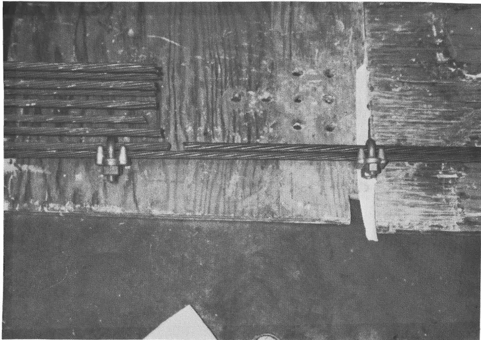
Figure 3.7 Strand Segment Serving as an Energy Dissipater
