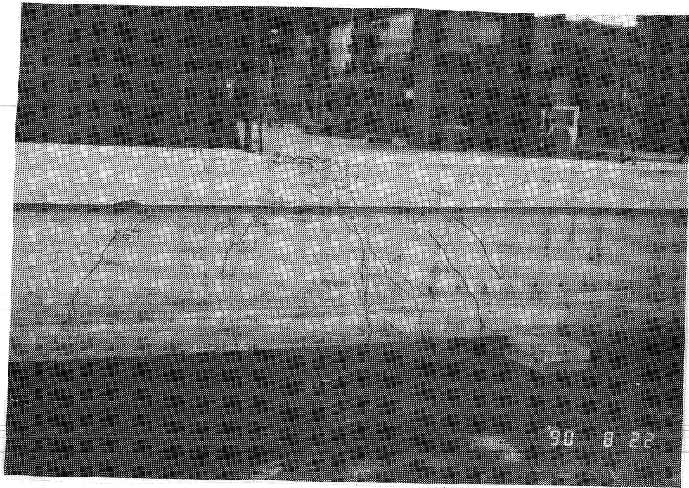
Figure 4.8 Crack pattern for FA460-2A.
