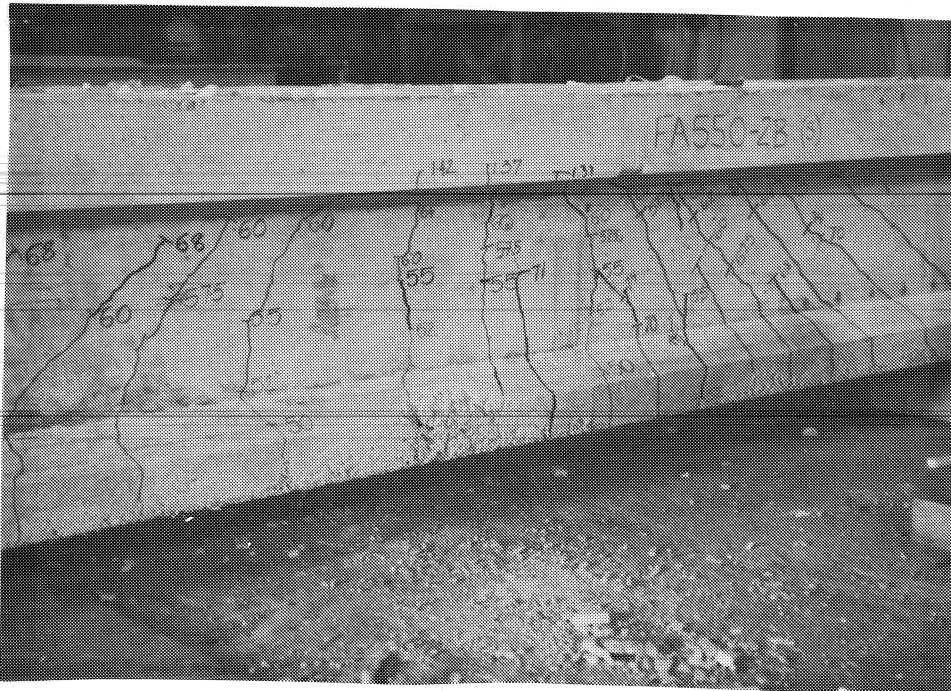
Figure 4.7 Crack pattern for FA550-2B.
