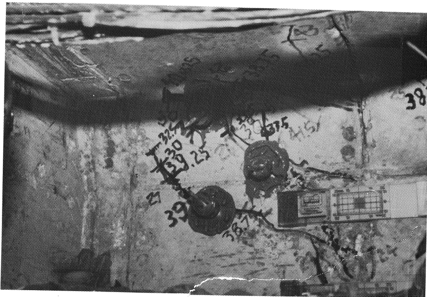
Figure 2.21 Injection ports.
