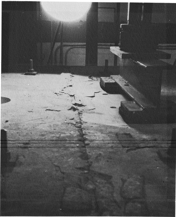
Figure 3.61 Crushing of top flange in epoxy joints span.
