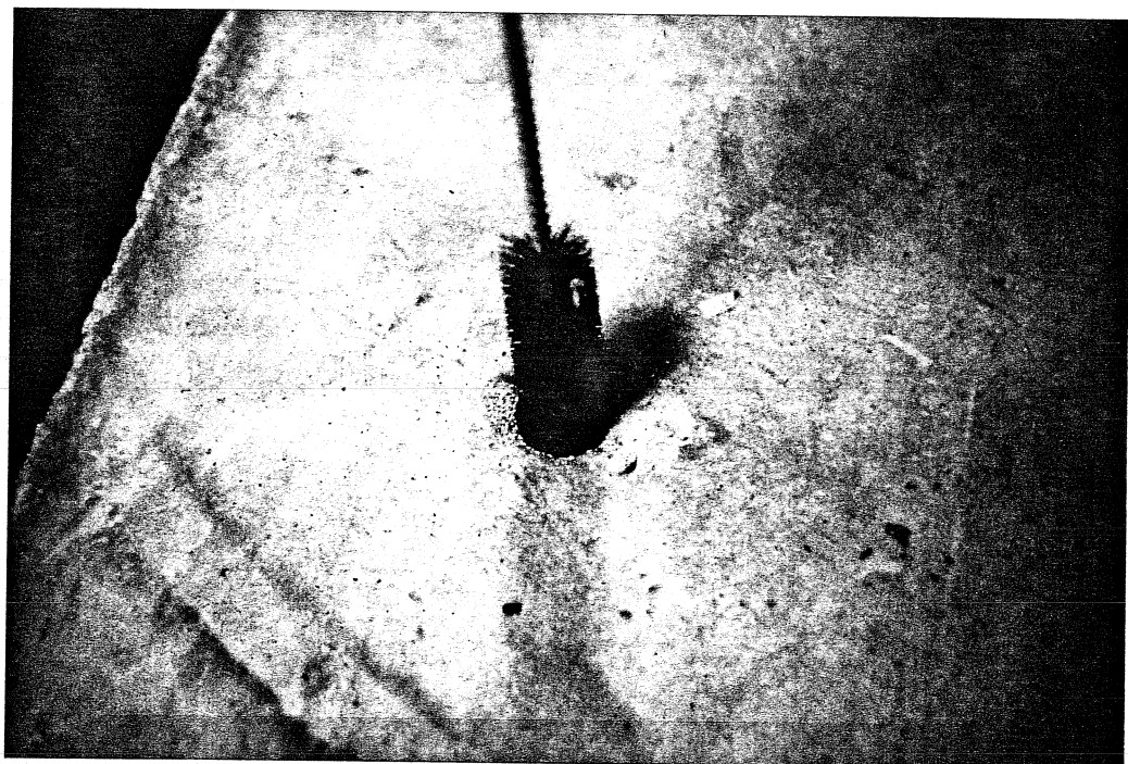
Figure 4.5 Cleaning holes with bottle brush.
