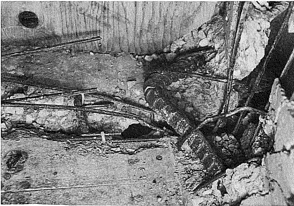
Figure 3.70: Specimen 9MLP22 Interior View of Post-Tensioning Bar
