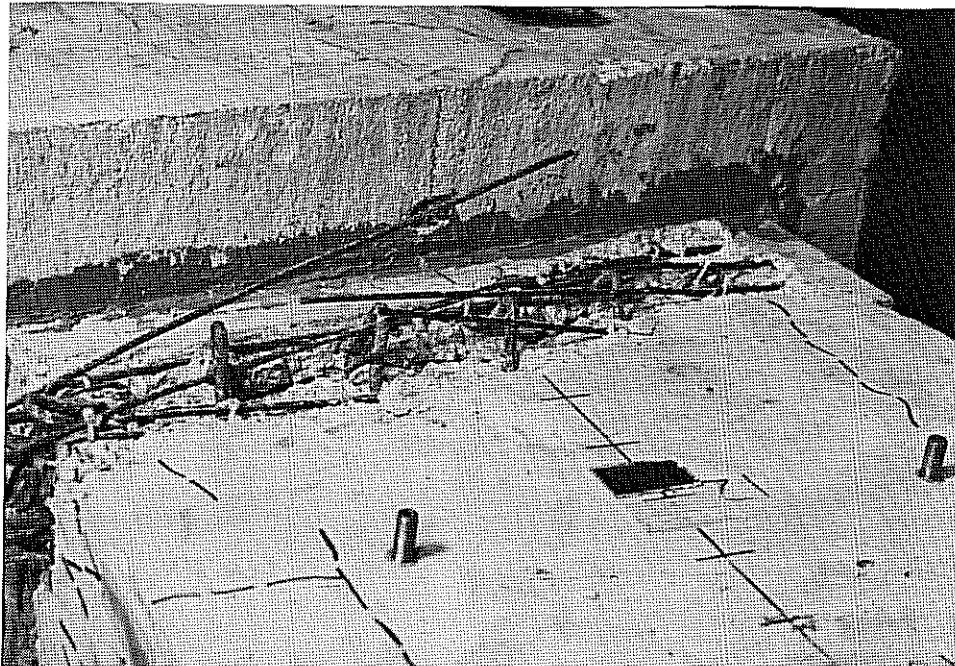
Figure 3.54: Specimen 7S22 Side Face Close-Up
