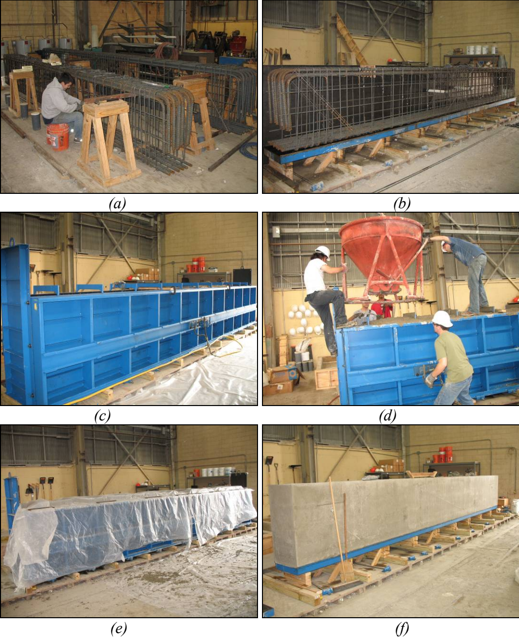
Figure 3.20: Fabrication of a typical beam: (a) assembly of reinforcement cage (b) placement of cage in formwork (c) forms in place prior to concrete placement (d) placement of concrete (e) beam curing (f) test specimen after the removal of forms.
