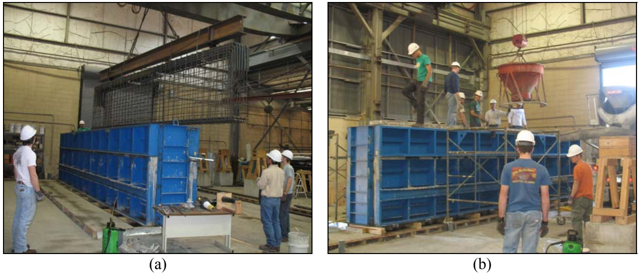
Figure 3.21: Fabrication of a 21''x75'' beam: (a) movement of reinforcement cage into formwork (b) placement of concrete into steel formwork
