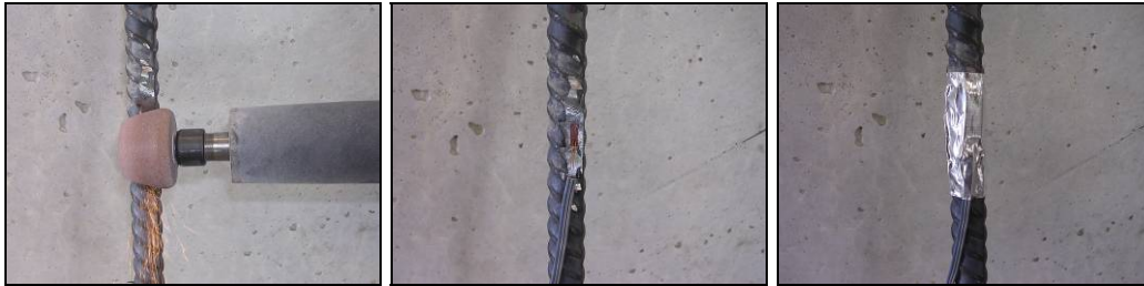
Figure 3.23: Installation of strain gauge for measuring steel strains.
