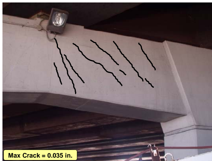
Figure B.1: I-45 over Greens Road Bent Cap
