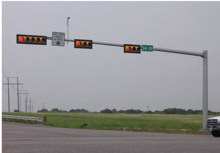
Figure 1.3: Typical Cantilevered Traffic Signal Structure in Texas
