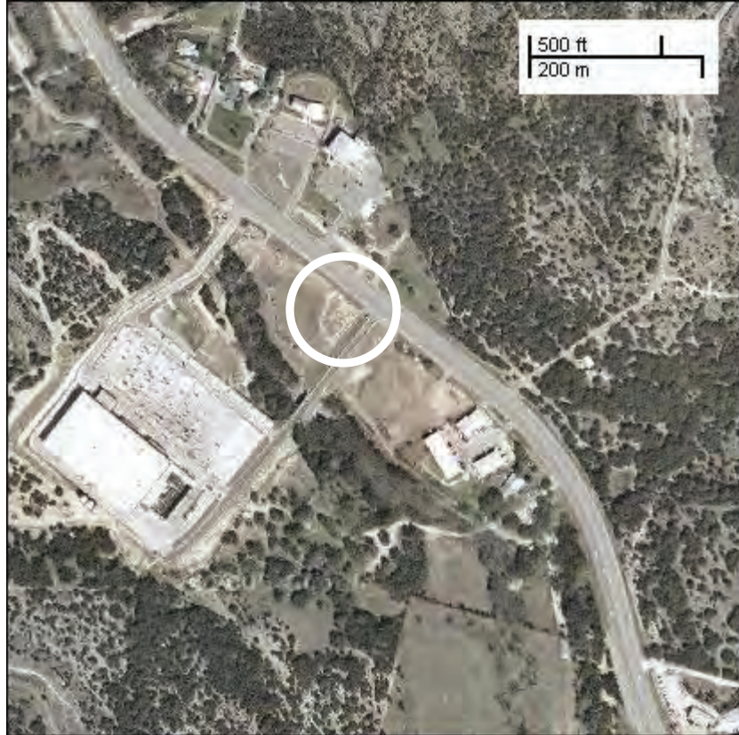
Figure 3.3: Aerial View of the Field Test Site on RM 620 at Home Depot Blvd (Google Maps, 2006)
