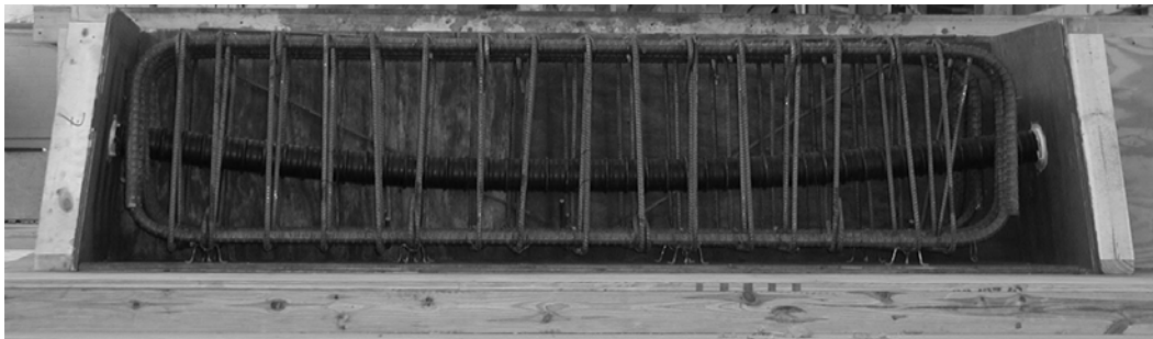
Figure 4-5 Assembled Specimen Cage, Duct, and Formwork
