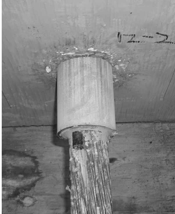
Figure 5-6 Live End of Specimen 0-SP-7.5 o -2 after Testing
