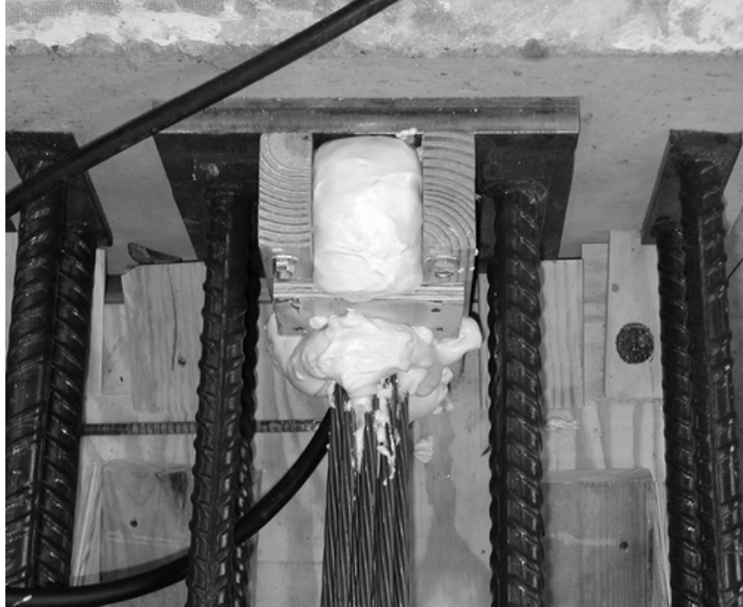
Figure 4-8 Sealing of Duct Ends
