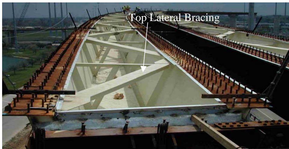
Figure 3.1 Top Flange Lateral Truss
