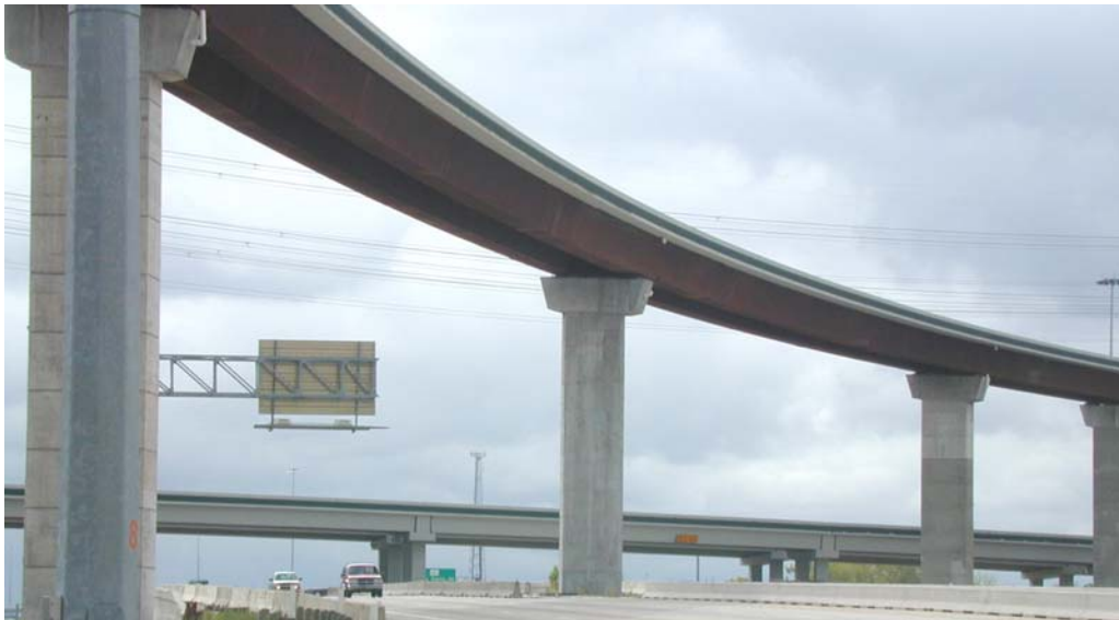
Figure 1.1 Trapezoidal Box Girder Bridge
