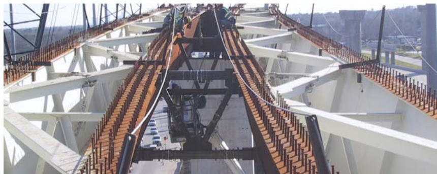
Figure 1.4 External box girder bracing
