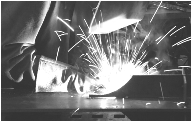
Figure 2-13: Welding the Web to the Flange
