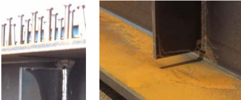
Figure 1-7: Wrapped Intermediate Stiffener Welds
