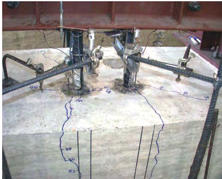
Figure 6.3 Widespread Splitting in Test 13
