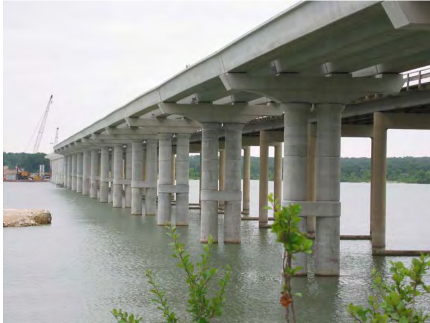
Figure 3.10 Construction of the Lake Belton Bridge
