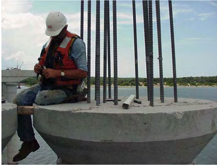
Figure 4.4 Observed Alignment of Connectors – Lake Belton Bridge Project
