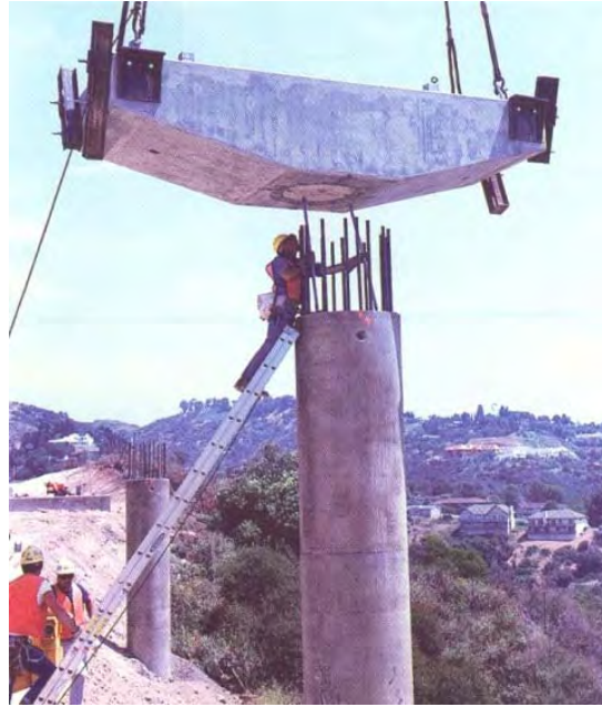
Figure 2.6 Precast Crossheads Used in the Getty Center People-Mover System Project (Josten et al. 1995)
