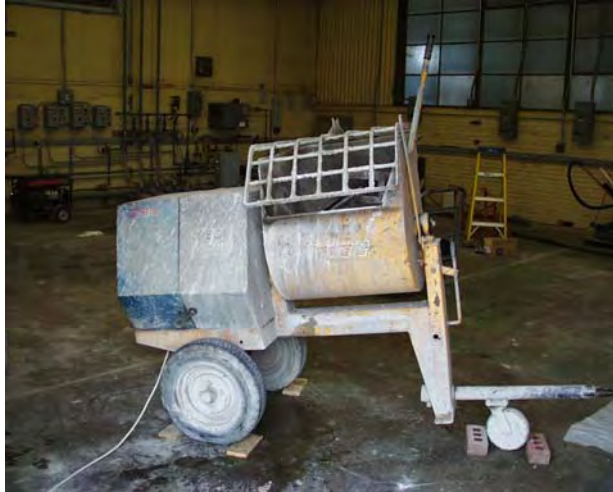
a. Mortar Mixer Used to Mix Grout
