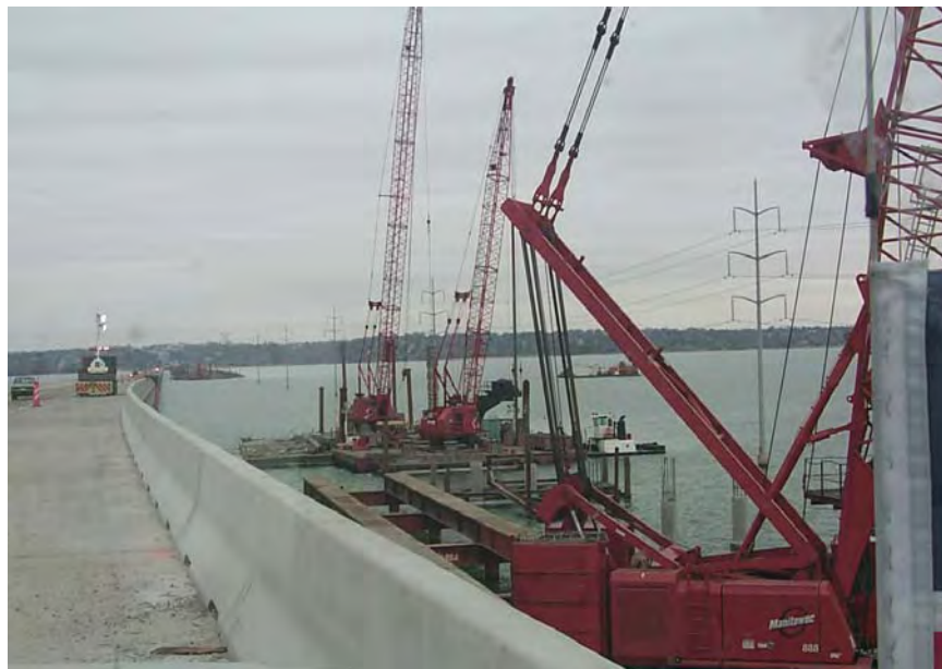
Figure 3.6 Lake Ray Hubbard Bridge Construction Site (Friggle 2002)
