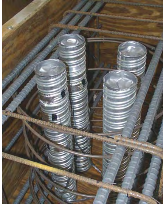
Figure 5.7 Completed Strain Gage Installations on Galvanized Steel Ducts
