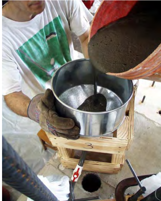
Figure 4.14 Gravity Tremie-tube Technique to Fill Ducts with Grout
