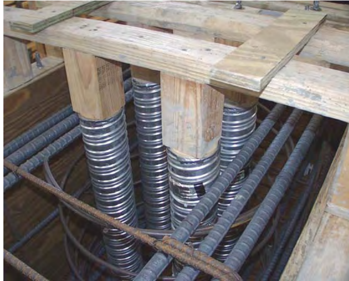
Figure 4.10 Vertical Alignment of Ducts during Concrete Placement
