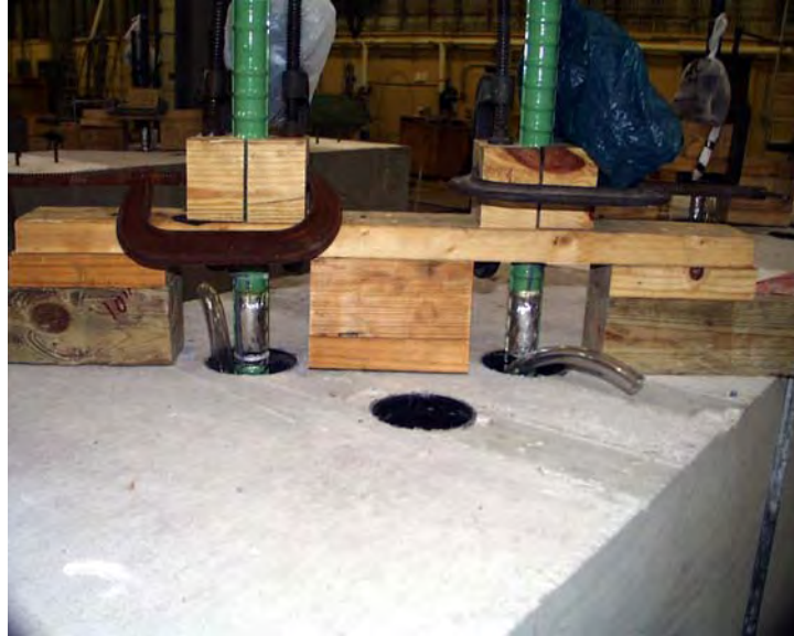
Figure 4.13 Formwork to Hold Connectors Aligned during Grouting
