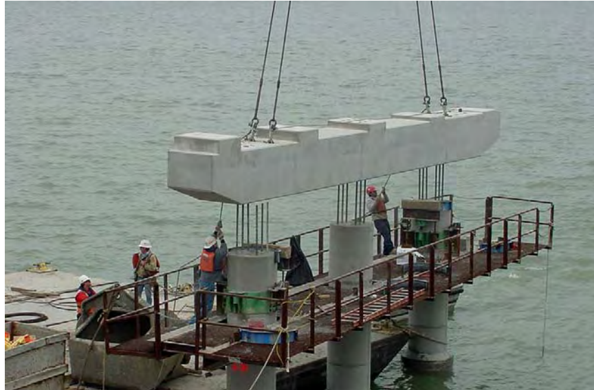
Figure 3.7 Lake Ray Hubbard Bridge Project
