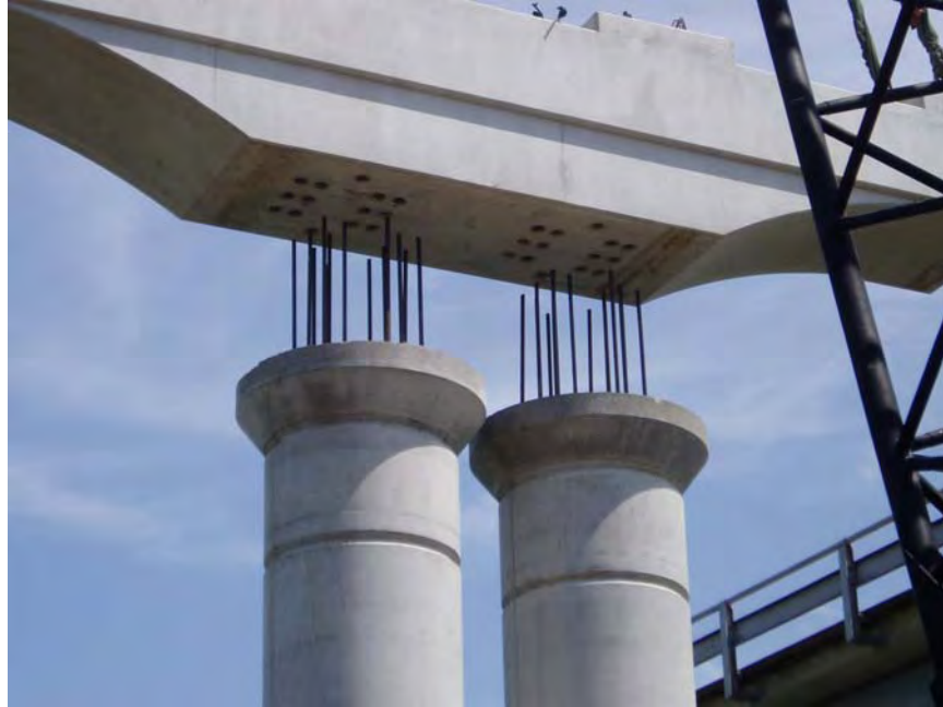
Figure 3.12 Lake Belton Bridge Project
