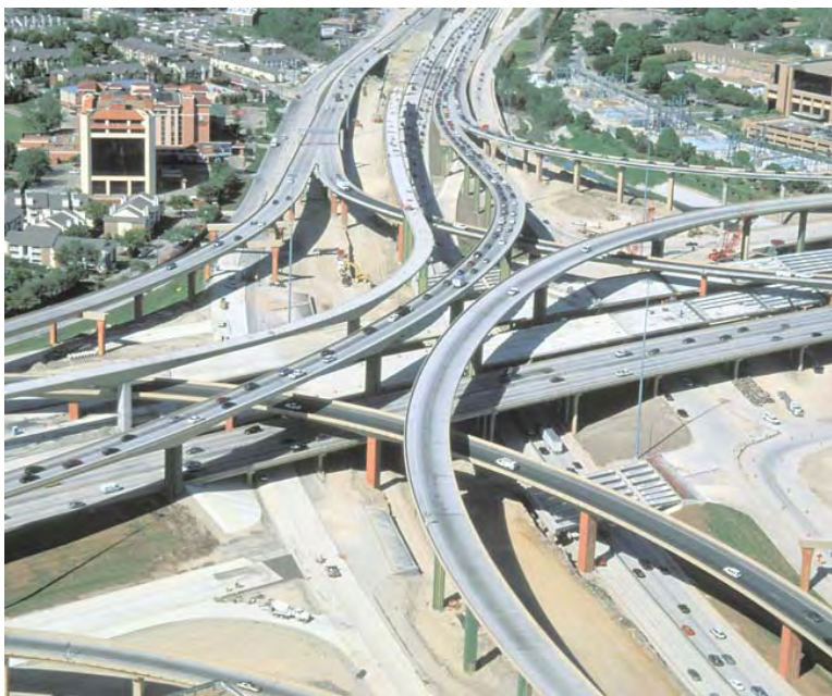
Figure 3.15 Aerial View of Dallas High Five Interchange Construction Site
