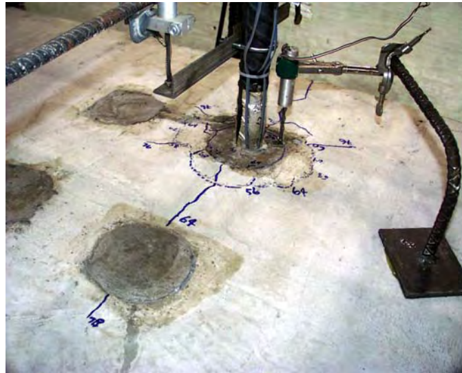
Figure 6.7 Splitting Cracks in Test 9
