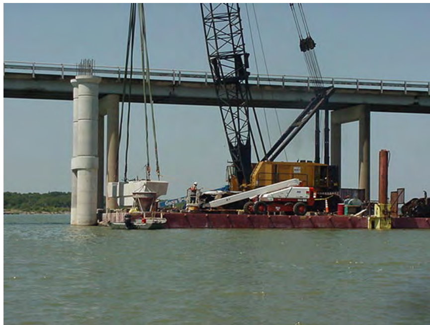
Figure 3.14 Bent Cap Placement Operation with Barge-mounted Crane
