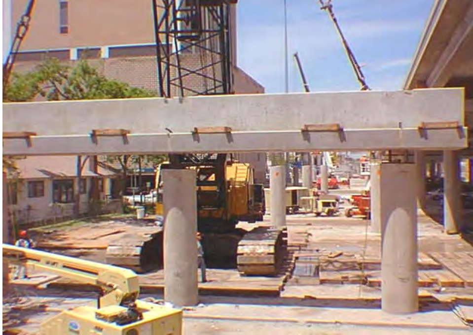
Figure 1.3 Pierce Elevated Project
