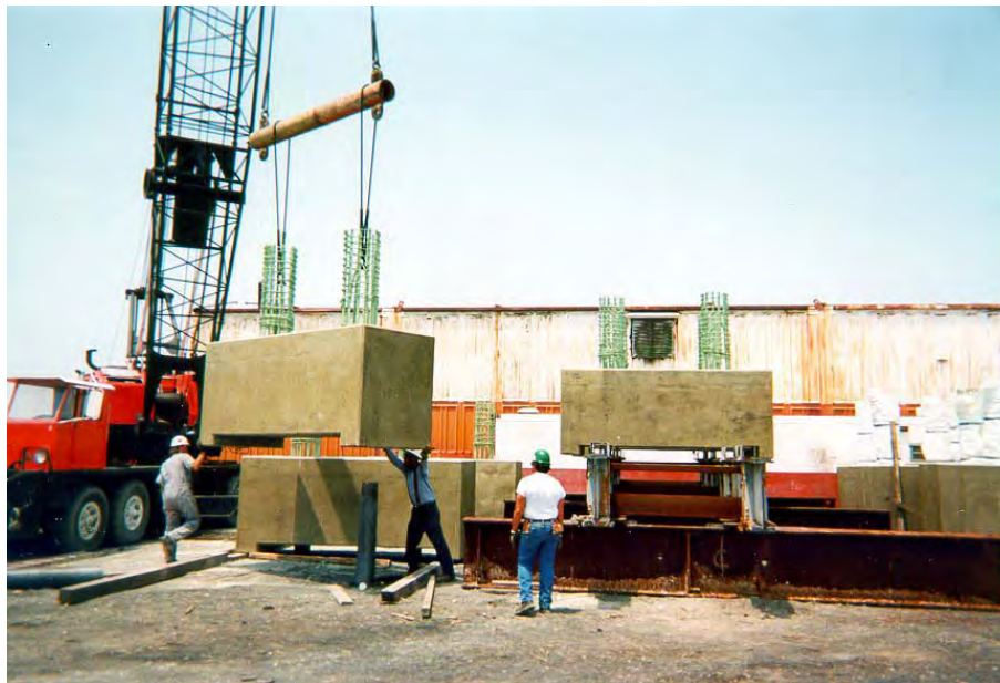
Figure 2.8 Beaufort and Morehead Railroad Trestle Bridge Bent Caps (FHWA 2005a)
