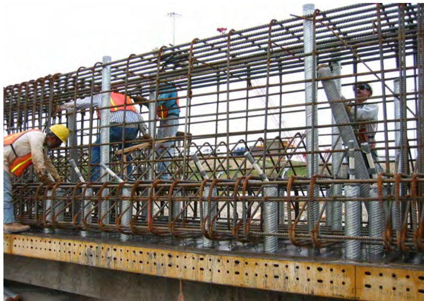
Figure 3.17 Placement of Bent Cap Reinforcement and Ducts
