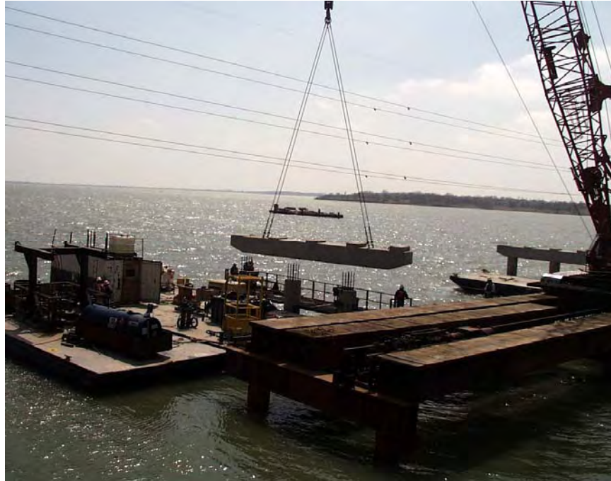
Figure 3.9 Bent Cap Placement Operations
