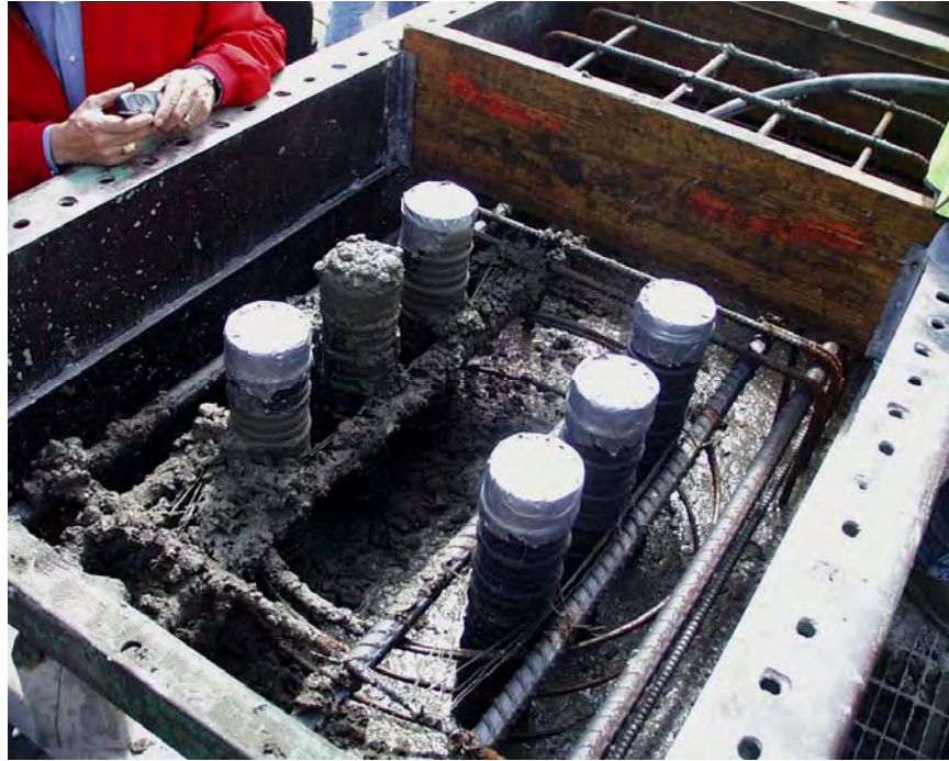
Figure 3.8 Bent Cap Connection Zone under Construction
