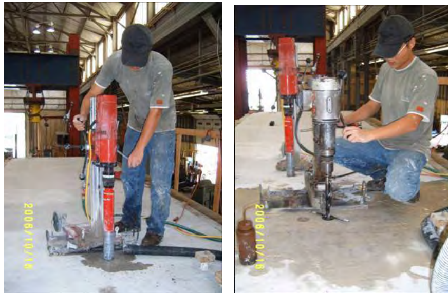
Figure 5.5: Coring and drilling into the specimen
