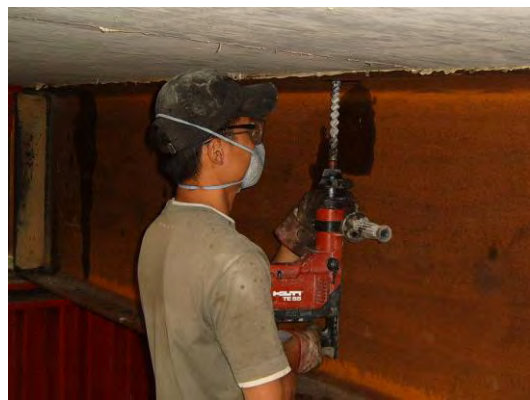
b) Drilling into the concrete
