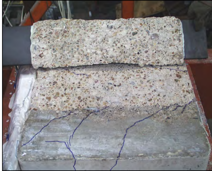
Figure 3.25: Epoxy plate failure of the concrete below the adhered surface (3MEPX)
