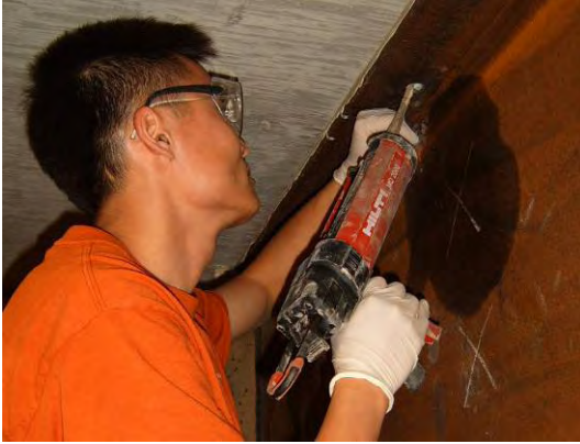
c) Injecting adhesive
