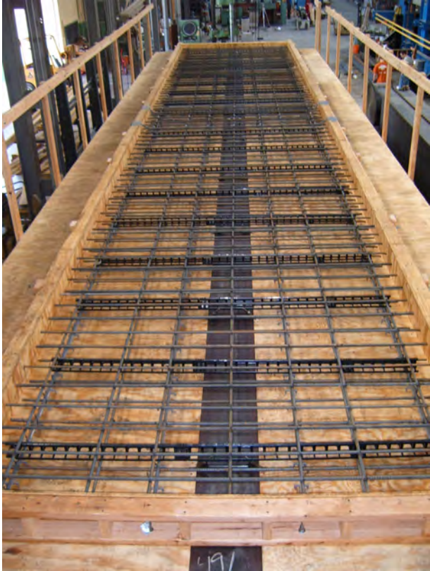
Figure 5.2: Reinforcement layout
