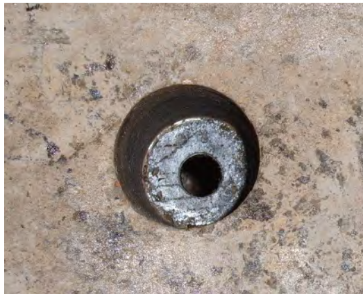
Figure 5.7: Drilled holes for DBLNB installation
