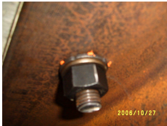
Figure 5.8: Use of "Squirter" Direct Tension Indicating (SDTI) washer
