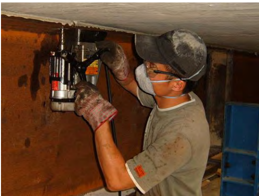
a) Drilling through the steel flange
