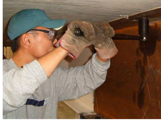
d) Tightening with torque wrench
